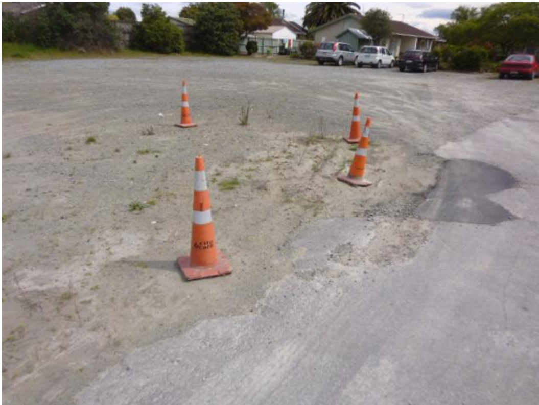
Photograph 10 Evidence of liquefaction occurring in the car park
