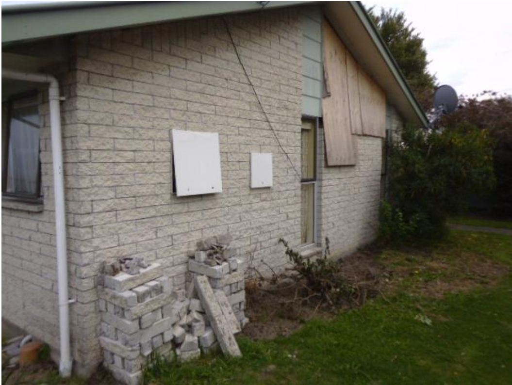
Photograph 5 View of collapsed brick gable veneer at north-eastern end of Block C
