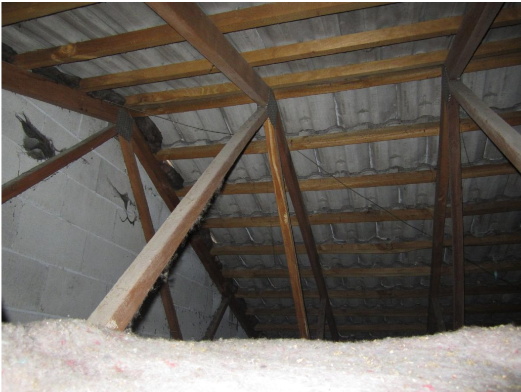
Photograph 12 Timber nail plate roof trusses and concrete tile cladding
