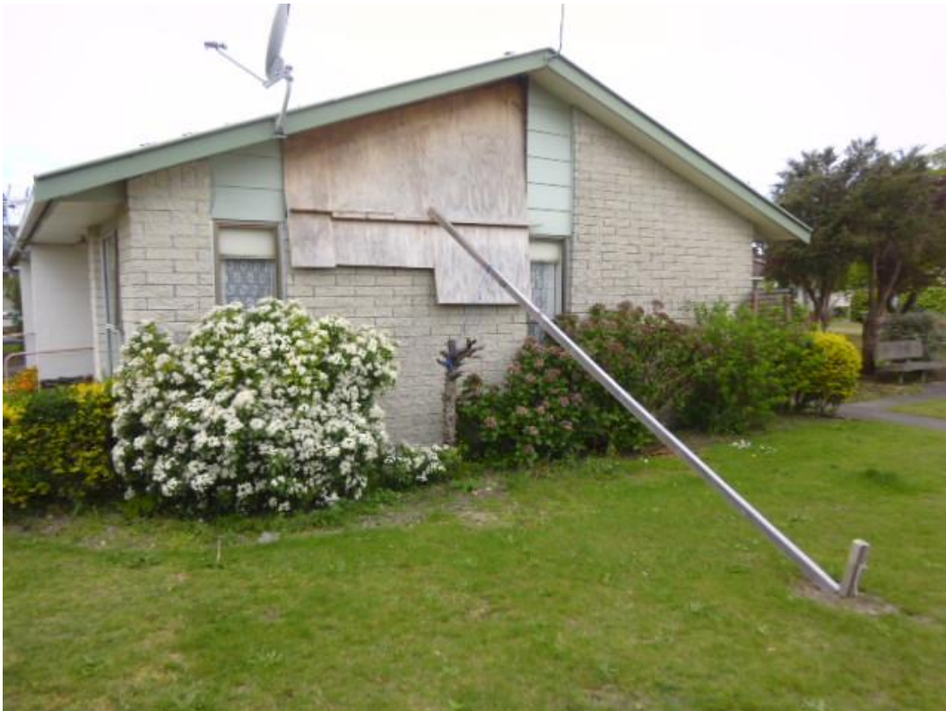
Photograph 6 View of collapsed brick gable veneer at south-western end of Block C
