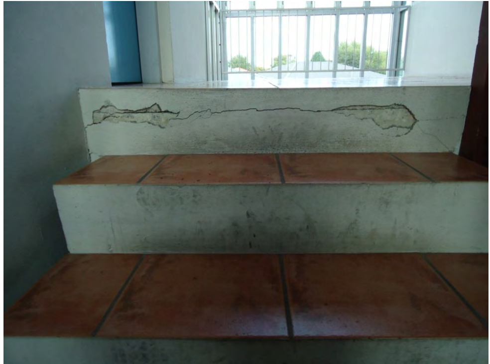
Photograph 4 Minor Spalling and Cracking at the Construction Joint between Landing Slab and Staircase
