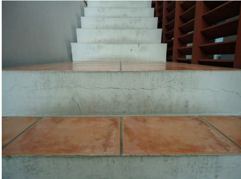
Photograph 6 Minor Spalling and Cracking at the Construction Joint between Landing Slab and Staircase
