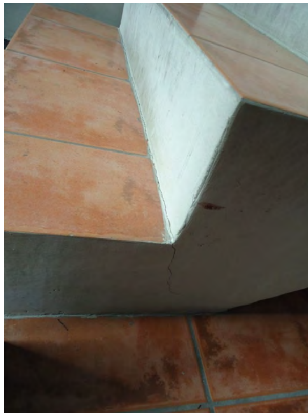
Photograph 5 Hairline Cracking at the Bottom of the Staircases
