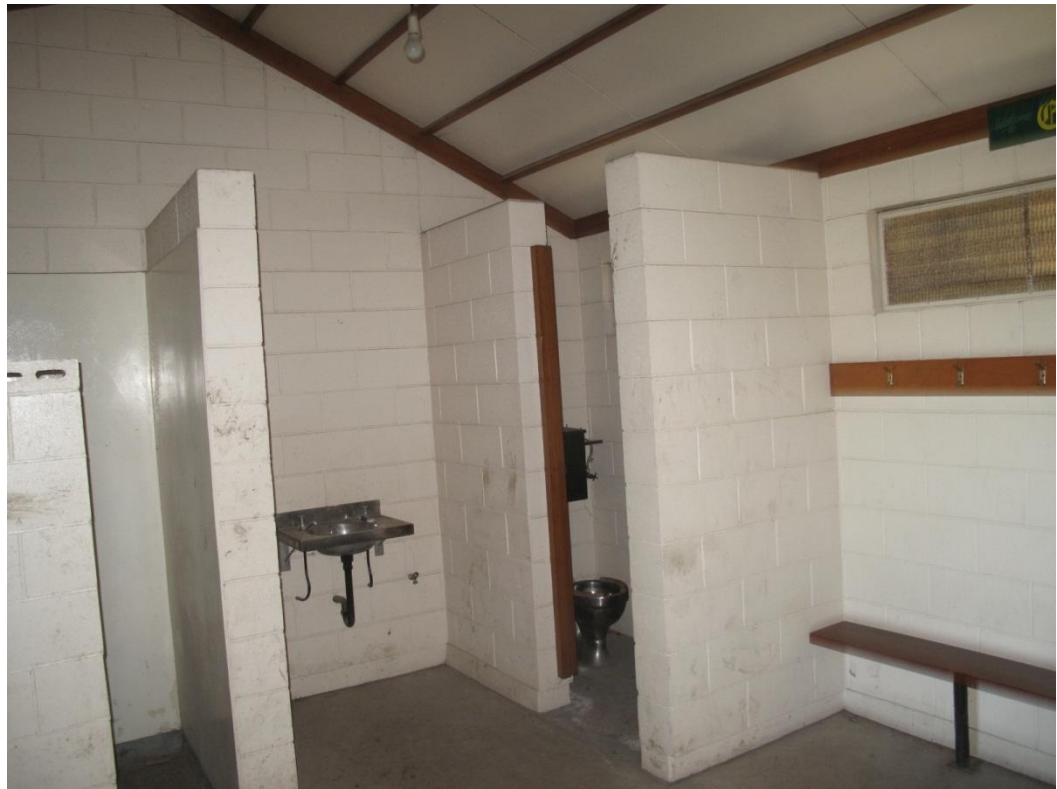
Photograph 8 Timber beam on the side and back walls connecting the roof to the masonry walls.
