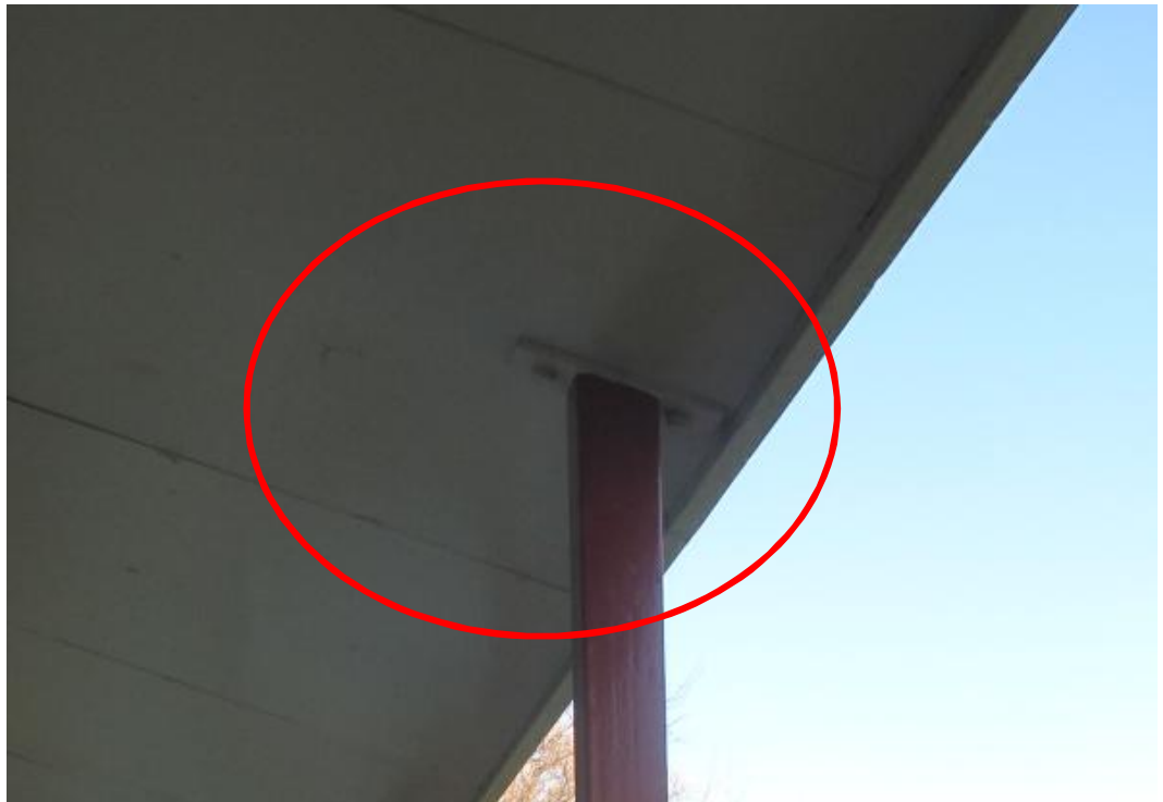
Photograph 10 Connection of steel canopy supports with timber beams.
