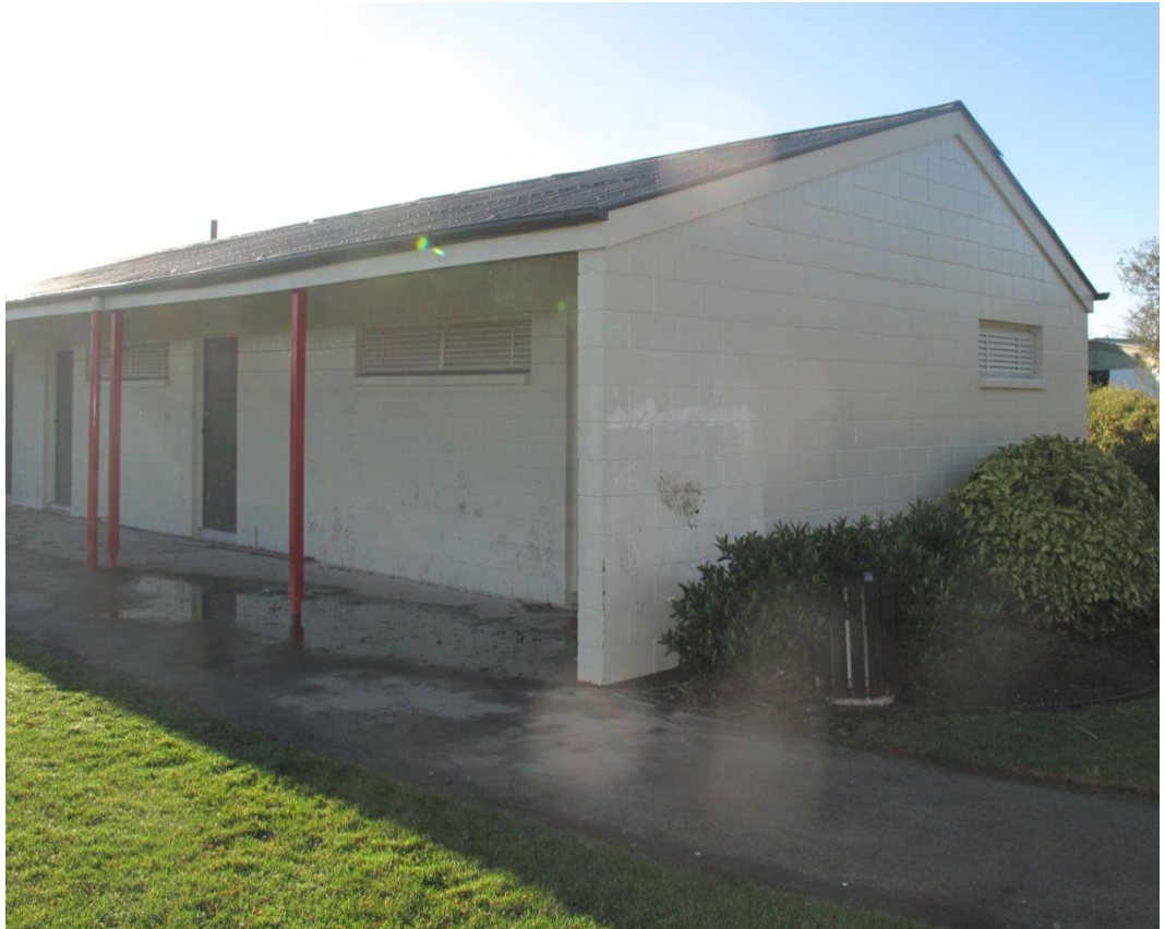
Photograph 9 Canopy over veranda area on the western side of pavilion.
