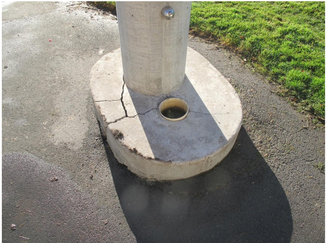
Photograph 5 Cracking in base of adjacent drinking fountain.
