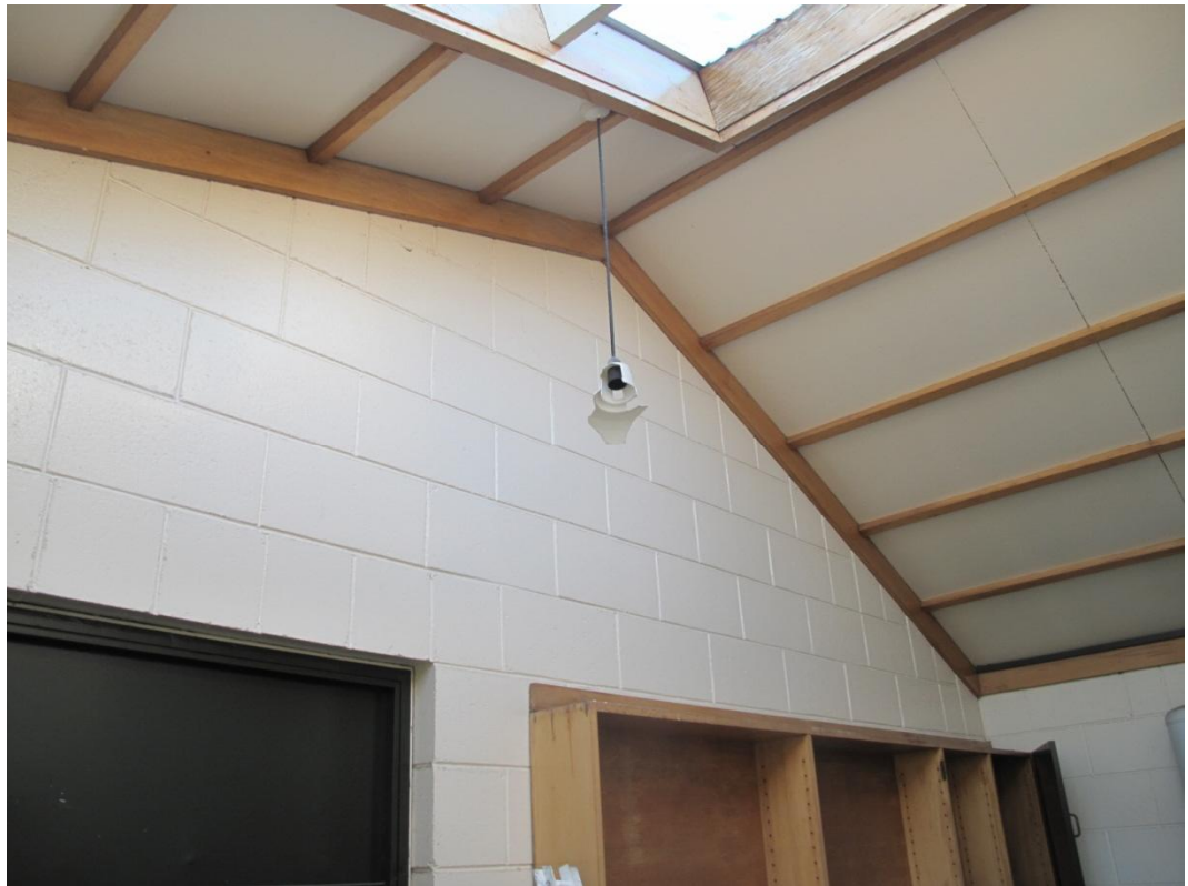
Photograph 7 Timber end beams and purlin edges.
