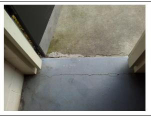
9 Separation of internal wall from external wall
