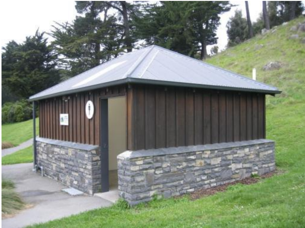
Photograph 2 View of toilet from the west.
