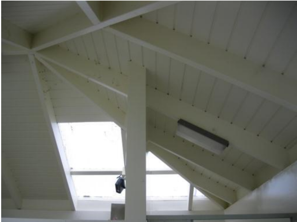
Photograph 7 Partition support to mid-point of rafter and hip beam.
