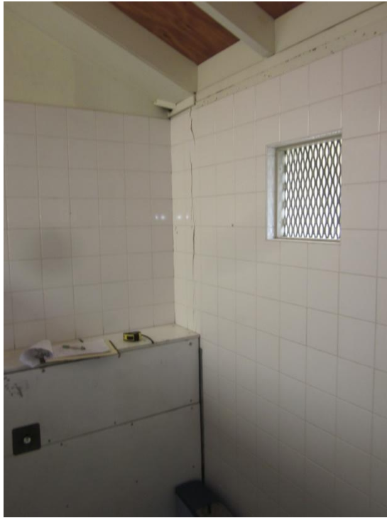
PHOTO 43: Vertical rupture in wall junction at 3/B.
