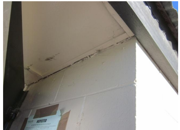
PHOTO 24: Gap opening up at wall and roof cladding at north toilet entrance.
