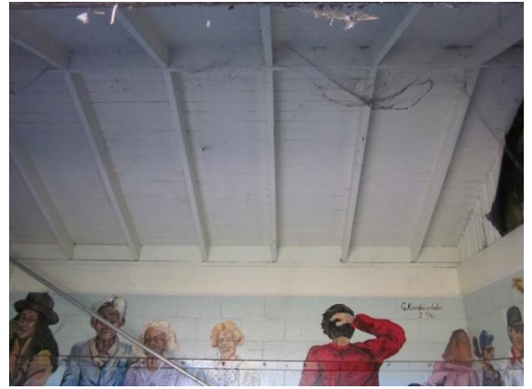
PHOTO 10: Timber-framed roof inside storage area.
