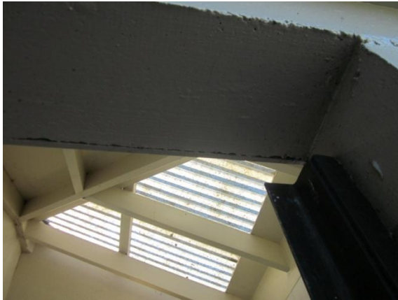
PHOTO 17: Gap opening up between masonry wall and internal wall cladding in locked toilet.
