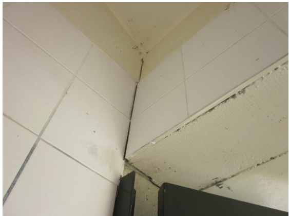
PHOTO 23: Gap opening up at interior wall cladding joints in north toilets.
