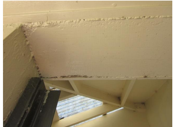
PHOTO 22: Gap opening up between interior cladding and masonry wall in north toilets (typical for both entrances).
