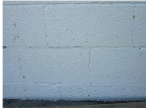
PHOTO 14: Step cracking along mortar joints on the east wall.
