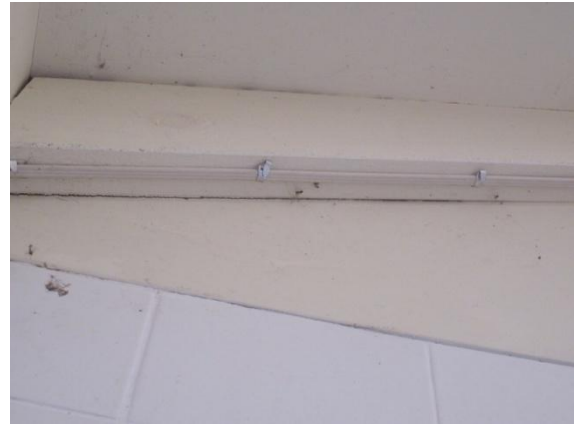
PHOTO 18: Gap opening up between interior wall and ceiling cladding and timber rafter in locked toilet..
