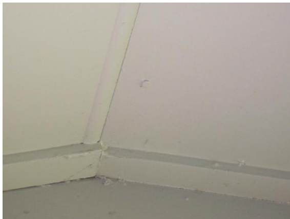
PHOTO 27: Gap opening up between joints in soffit lining on west side.
