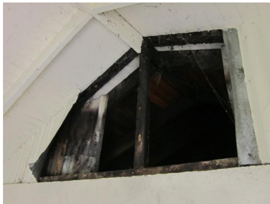
PHOTO 45: Roof timber elements compromised by fire – Stage 1 building (grid line 2/B-C)
