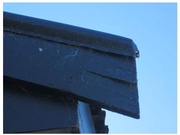
PHOTO 30: Existing defect to end of timber fascia on south side.
