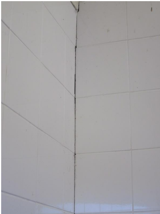
PHOTO 19: Gap opening up at internal wall joint in locked toilet.
