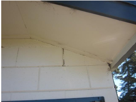
PHOTO 21: Existing low quality pointing on northeast corner.
