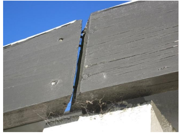
PHOTO 26: Gap opening up at connection between timber beams at roof level on the north side.
