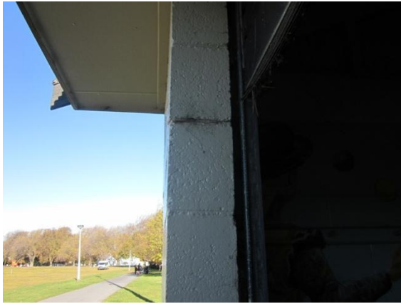
PHOTO 9: Joint between masonry wall and roller door for southern-most storage area.
