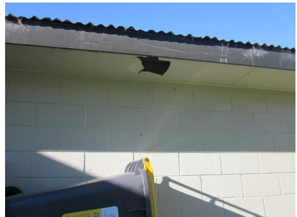
PHOTO 28: Existing impact damage to soffit lining on west side (not earthquake related).
