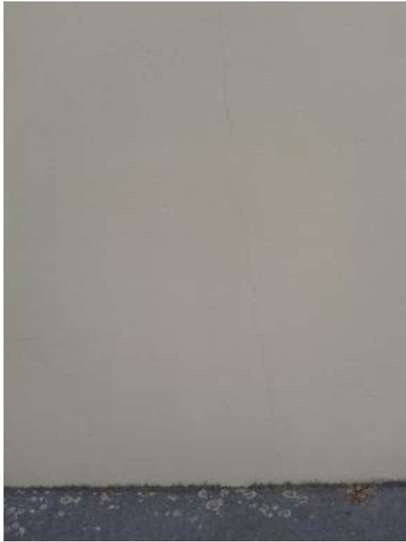
Photo 5. Hairline crack in the gable end wall.
