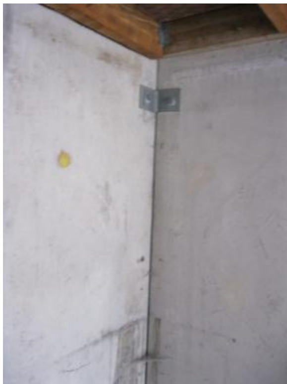
Photo 4. Cleat connection between rear and partition walls.
