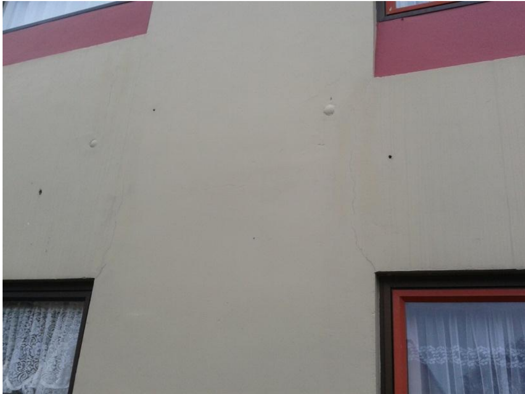
Photograph 3 Cracking to exterior walls at window corners.
