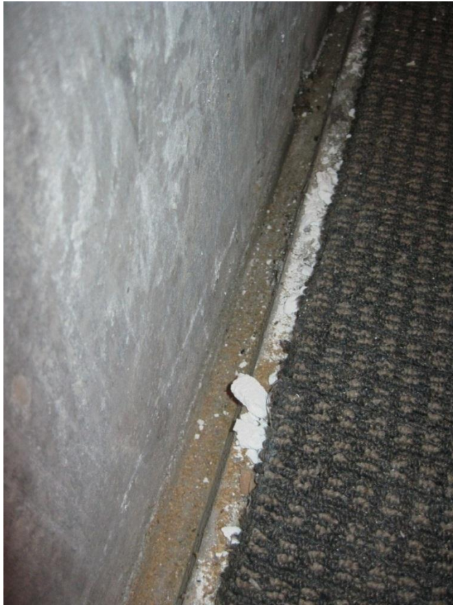
Photograph 15 Connection between cast in situ floor slab and precast panel wall at second floor level.
