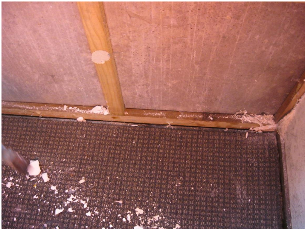
Photograph 14 Removal of wall linings to expose concrete panel wall to allow scanning for reinforcement details at second floor level.
