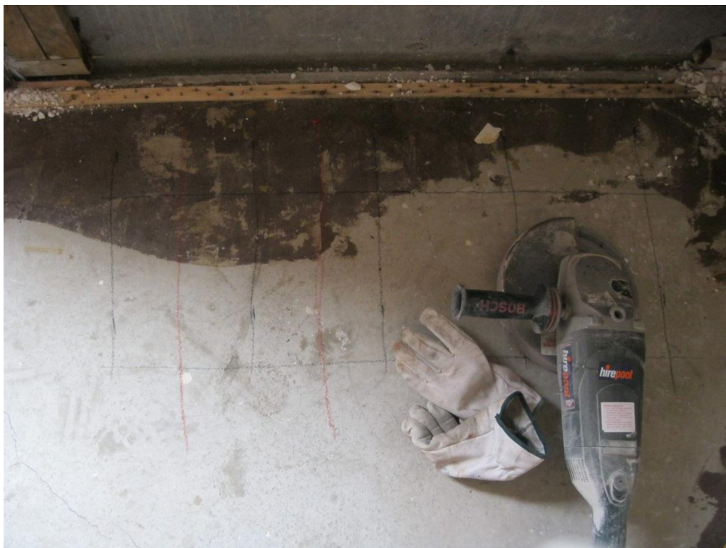
Photograph 20 Black lines indicating where reinforcement is expected to be found and red lines indicating area to be exposed.
