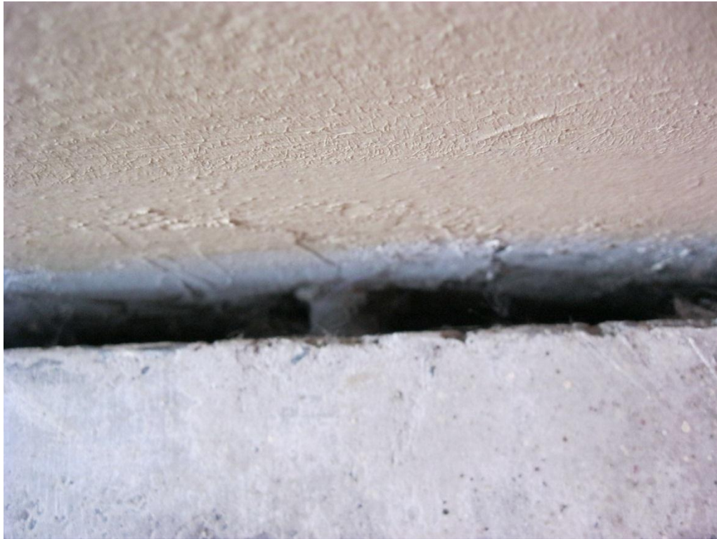
Photograph 9 Seismic gap between stairs landing and precast concrete wall panel showing steel dowel pin connection.
