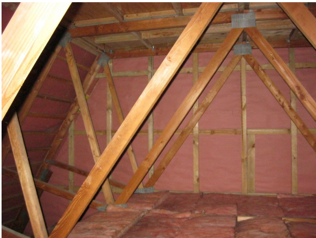
Photograph 10 Internal view of roof space showing inclined members of the timber truss and timber framing of the roof/gable wall.
