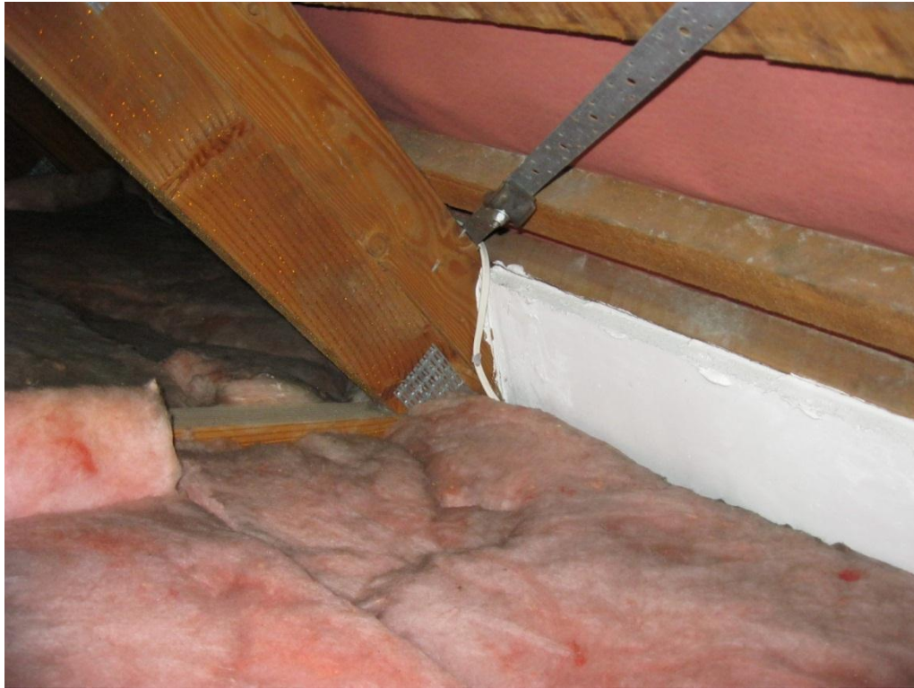
Photograph 13 End connection of flat steel strap roof cross bracing.
