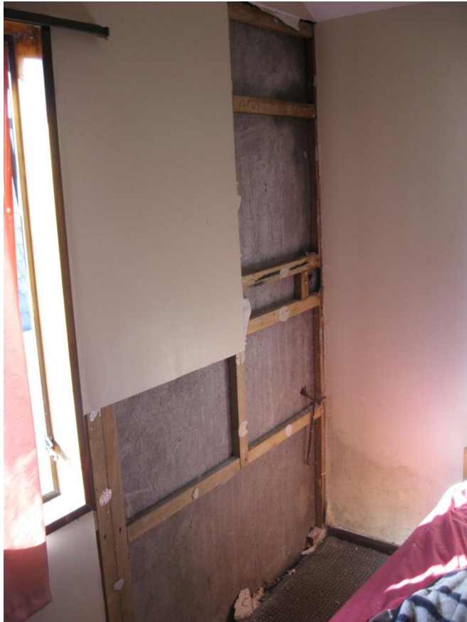
Photograph 17 Wall linings removed to expose angle cleat connection and precast concrete panel at second floor level.
