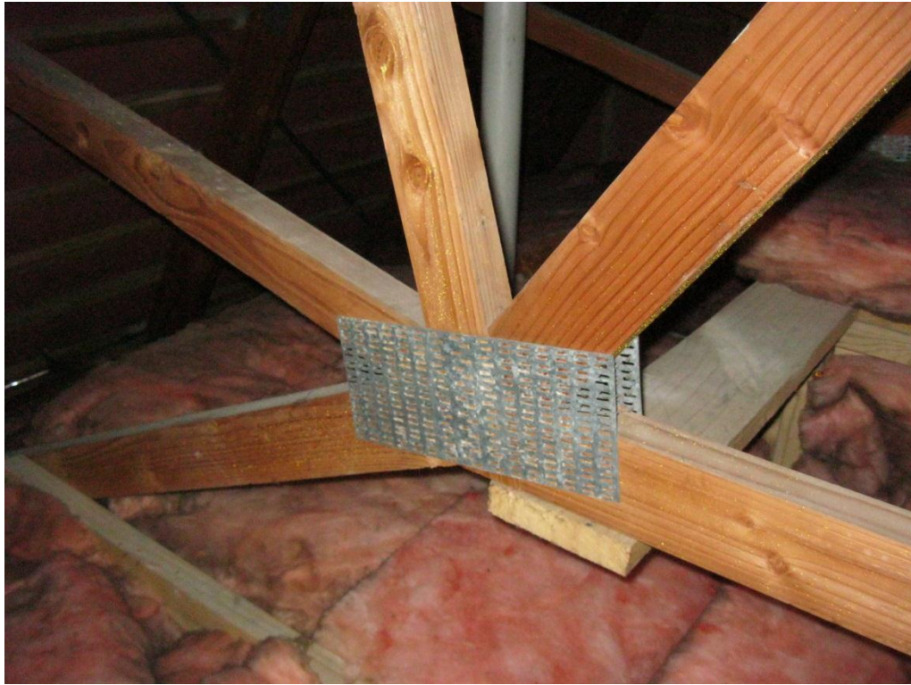
Photograph 11 Connection of timber roof truss members.
