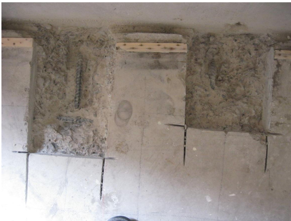
Photograph 22 Further opening up of the suspended slab showed the steel reinforcement cage not to be tied into precast wall from the top.
