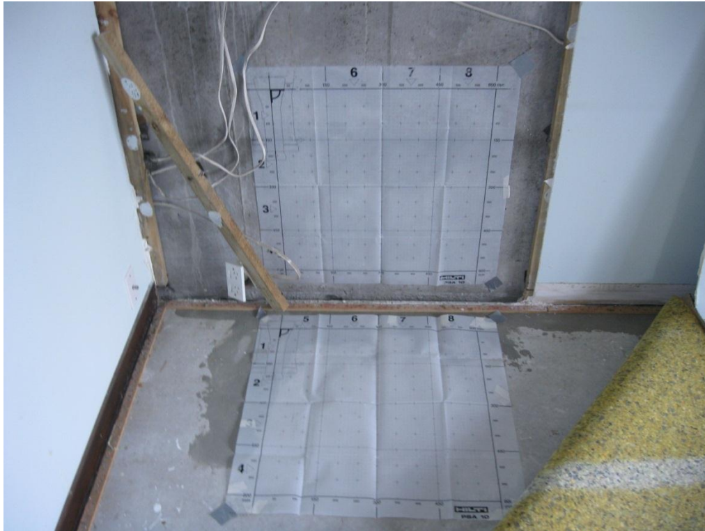
Photograph 19 Scan locations looking for details of connection between the precast panel and the cast in-situ suspended floor slab.
