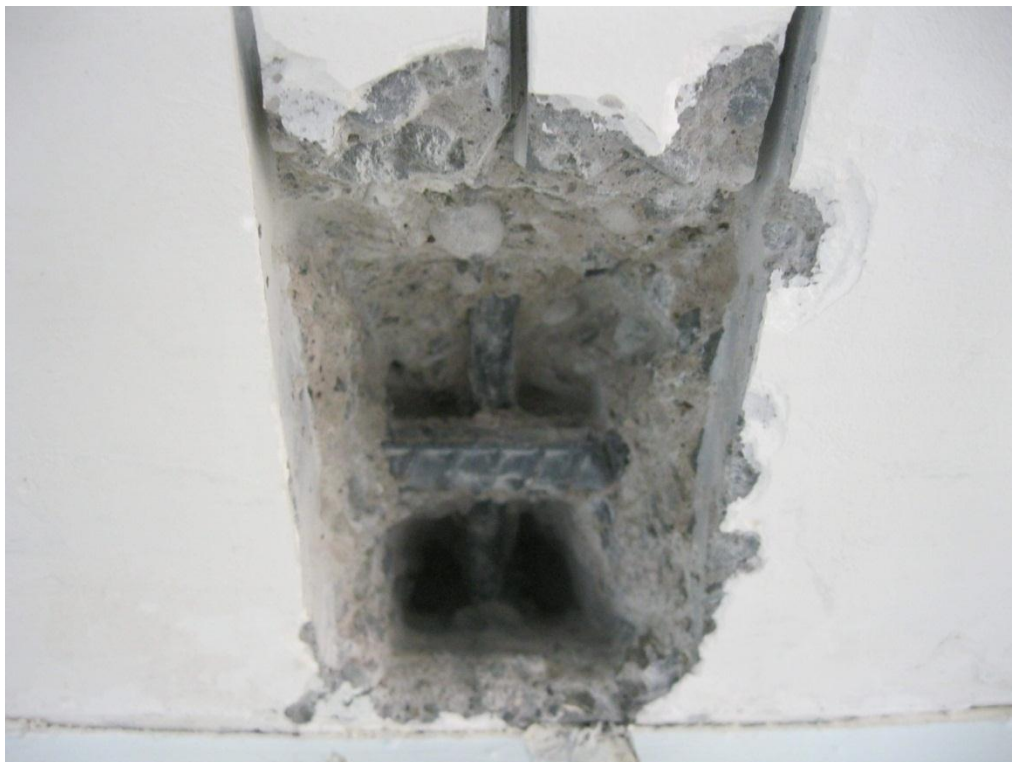
Photograph 24 Opening up in another location revealed a 10mm diameter steel bar tying the suspended slab back into the precast concrete wall panels.
