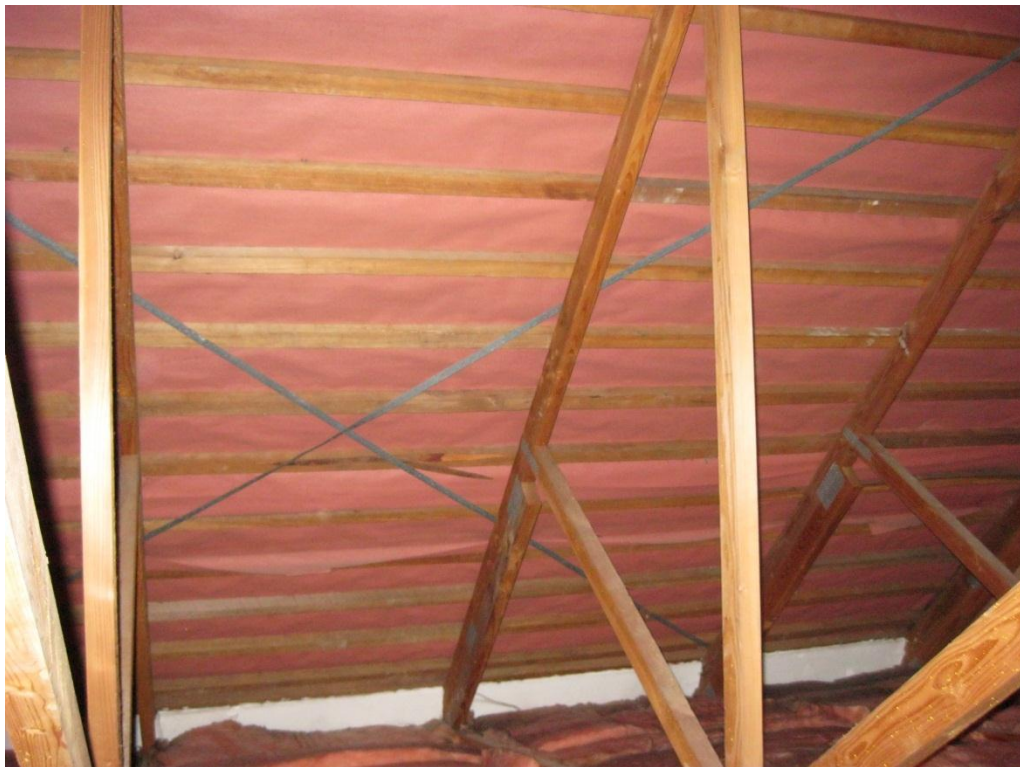
Photograph 12 Flat steel strap roof cross bracing.
