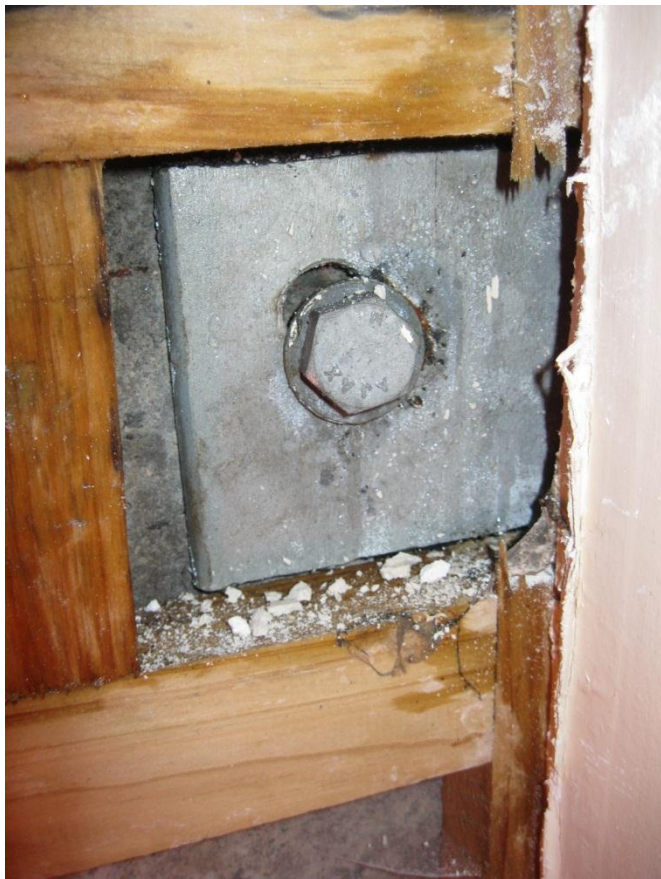
Photograph 16 Angle cleat connection between precast wall panels at second floor.
