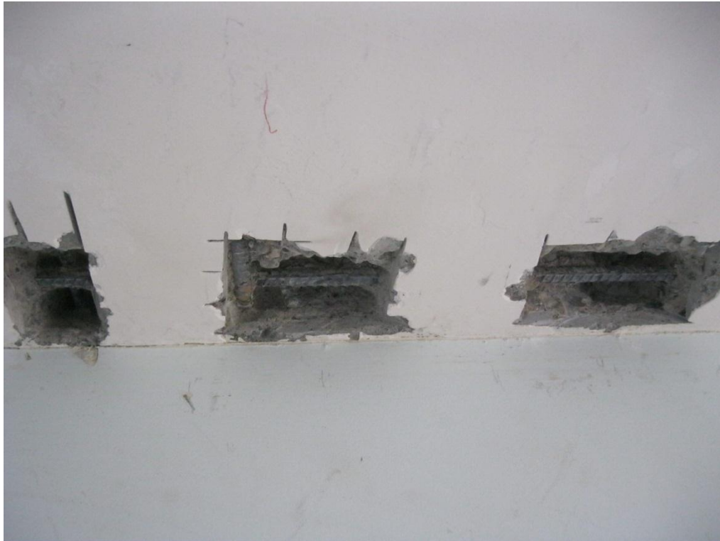
Photograph 25 Further opening up and reinforcement scanning revealed regular spacing of bars tying the slab into the precast panels at 250mm centres along all walls.
