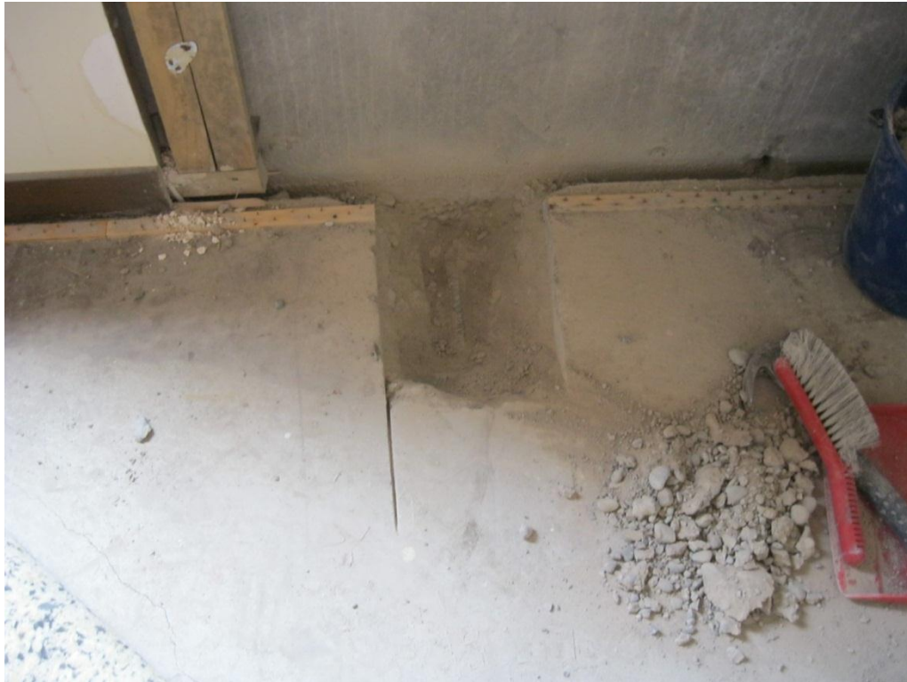
Photograph 21 Suspended slab steel reinforcement cage found not to be tied into precast wall from the top.
