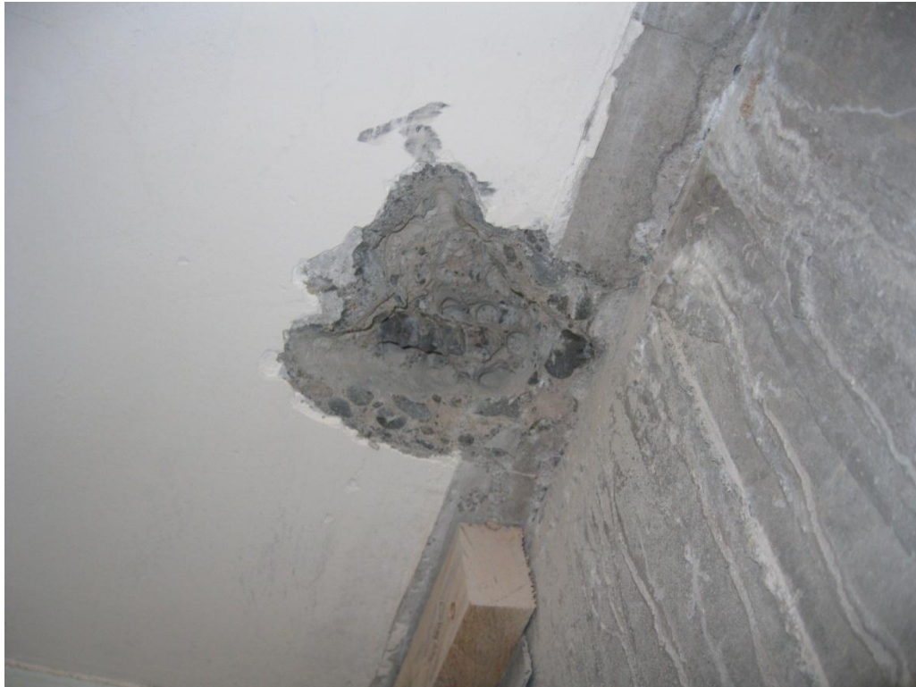
Photograph 23 Opening up to the underside of the second floor suspended slab showed the steel cage reinforcement not tied into the precast wall.
