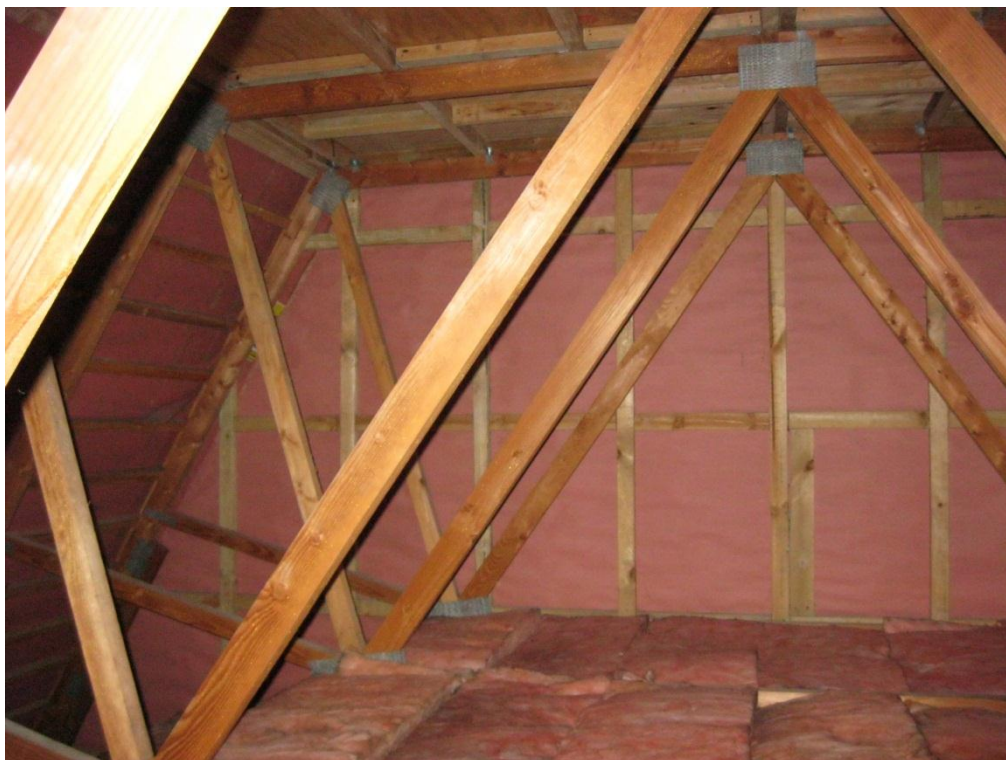
Photograph 9 Internal view of roof space showing inclined members of the timber truss and timber framing of the roof/gable wall.
