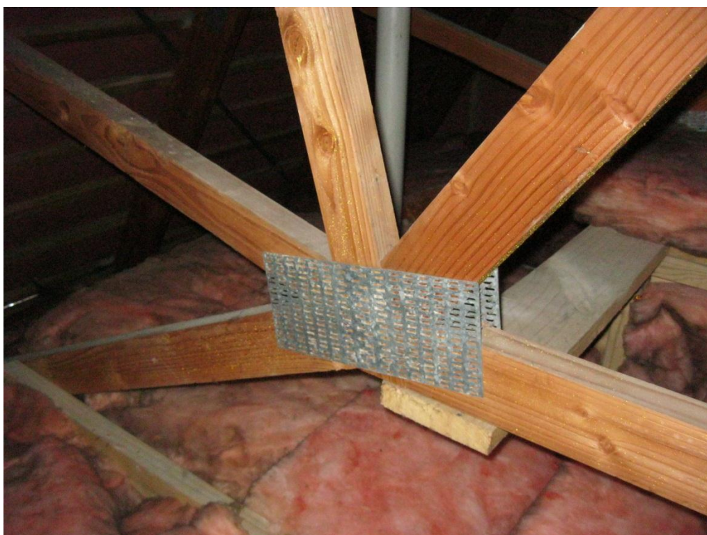
Photograph 9 Internal view of roof space showing inclined members of the timber truss and timber framing of the roof/gable wall.
