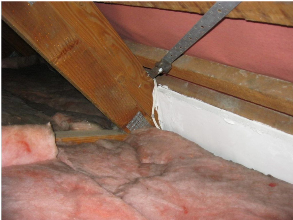
Photograph 12 End connection of flat steel strap roof cross bracing.
