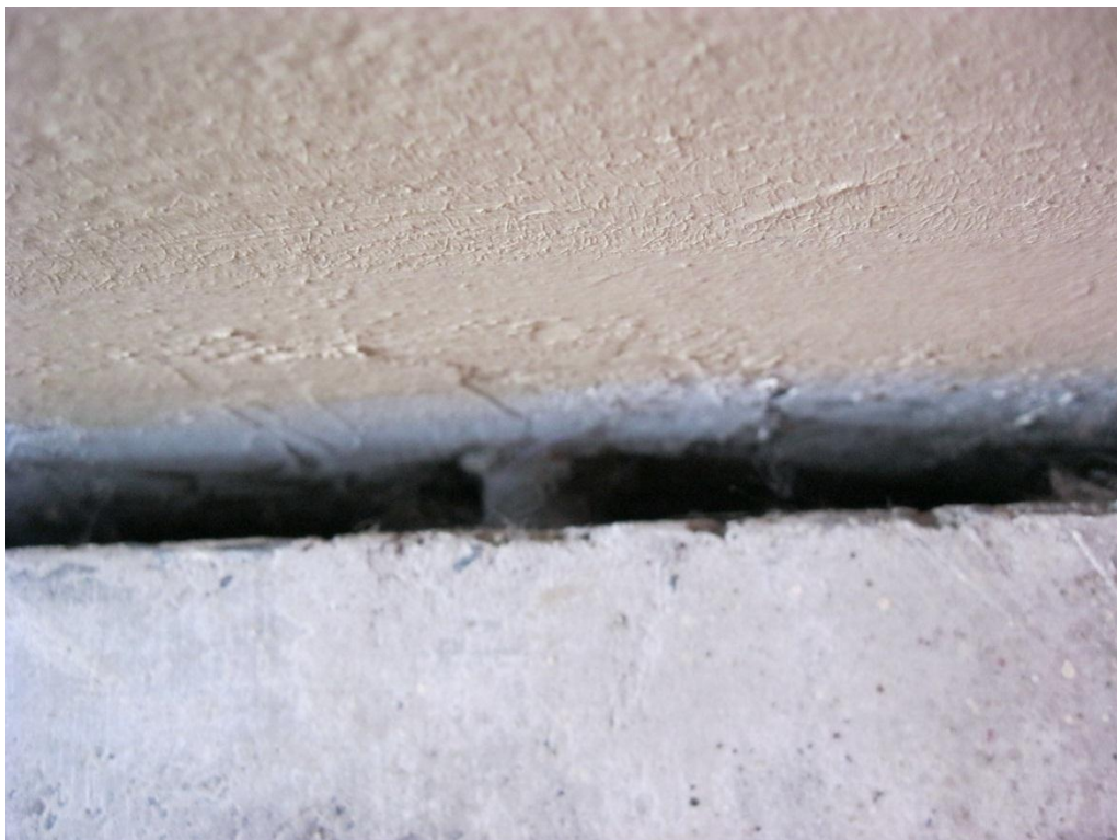
Photograph 8 Seismic gap between stairs landing and precast concrete wall panel showing steel dowel pin connection.
