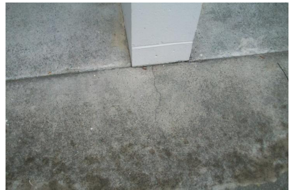
Photo 8: Minor cracking extending from the end of masonry walls
