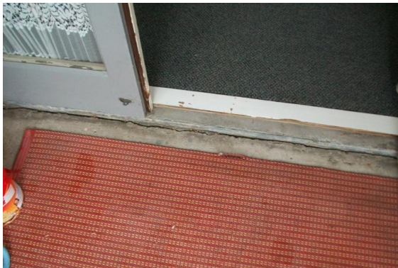
Photo 9: Concrete separation from the door penetration
