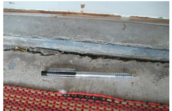
Photo 10: Gap opening of approximately 2mm with 5mm wide spalled at top
