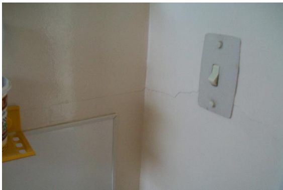
Photo 7: Hairline cracking through plasterboard lining extending from plasterboard penetrations
