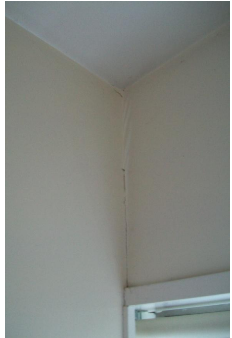
Photo 6: Vertical separation between plasterboard wall elements
