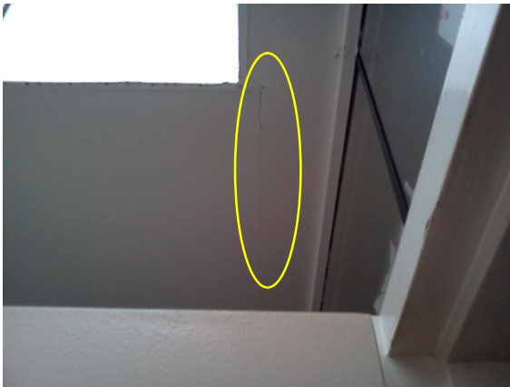
Photo 11: Cracking to the plasterboard ceiling linings extending from the skylight
