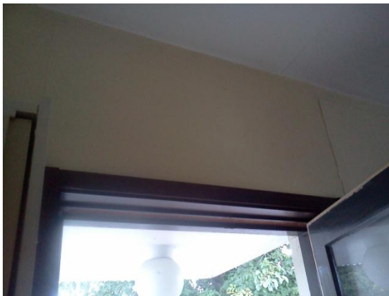
Photo 15: Separations between plasterboard sheets along the join
