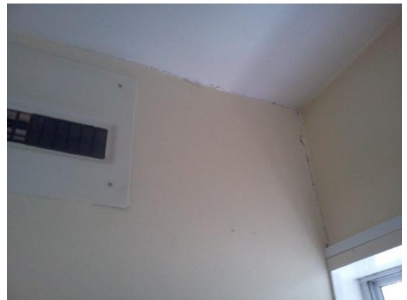
Photo 16: Junction separation
