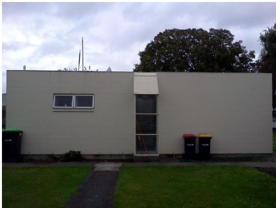
Photo 3: Typical block end walls consist of 200 series block
