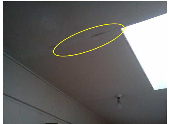
Photo 12: Cracking to the plasterboard ceiling linings extending from the skylight
