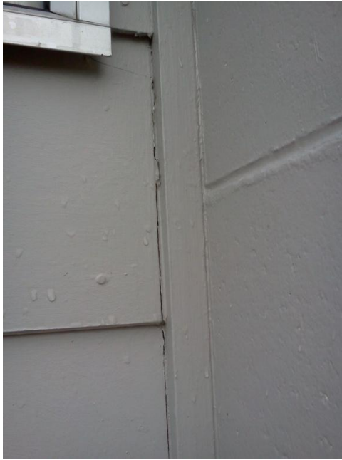
Photo 5: Separation along the weatherboards at the the wall junction
