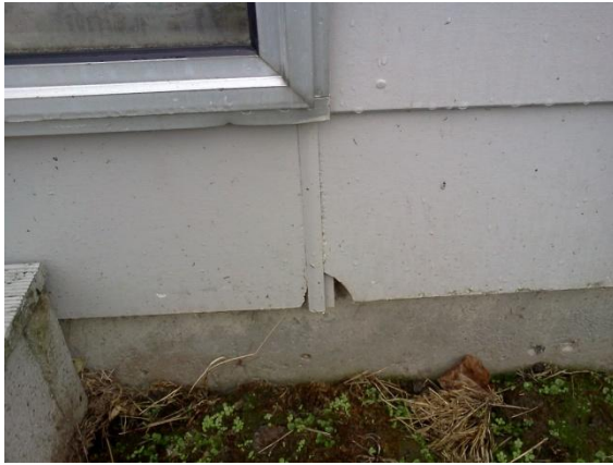
Photo 13: Typical damage to the weatherboard corners
