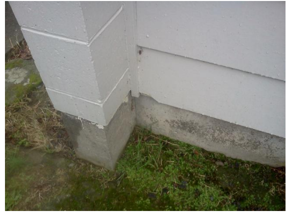
Photo 14: Timber to masonry wall junction detail and strip foundation
