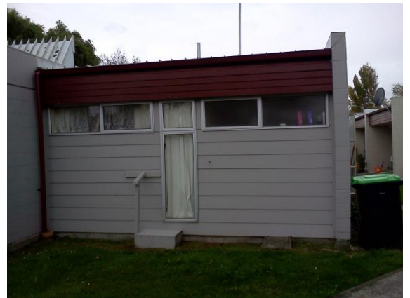
Photo 4: Typical rear of unit, light timber framed with weatherboard cladding.
