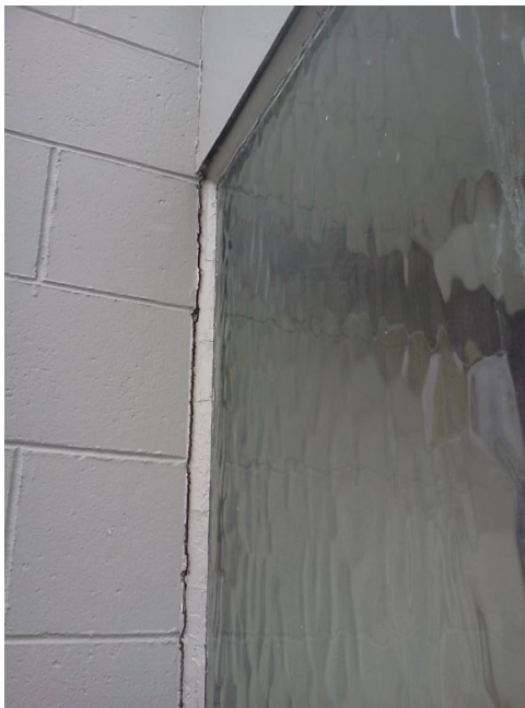
Photo 11: Separation between the masonry brick work and light timber framed wall
