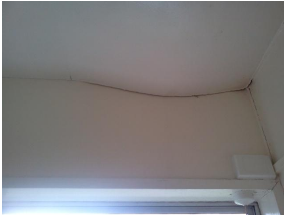
Photo 9: Sagging of the roof lining, unclear whether this is due to the individual boards
