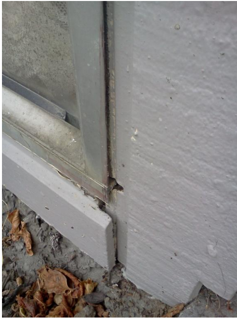
Photo 5: Gap opening around the window frames
