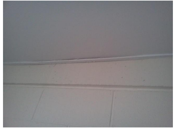
Photo 10: Sagging to the roof linings
