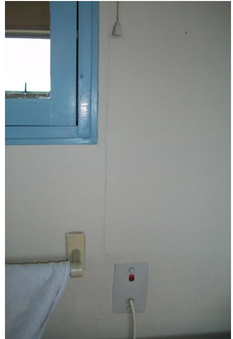
Photo 7: Vertical cracking through the plasterboard linings
