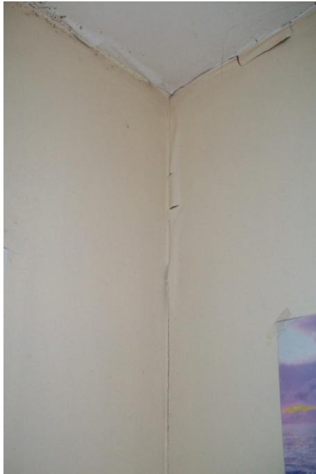
Photo 5: Photo 6: Separation of the plasterboard linings along the wall to ceiling junction and wall to wall junction
