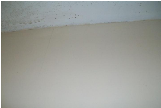
Photo 3: Vertical separation along the plasterboard
