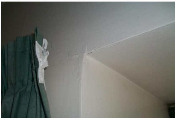
Photo 8: diagonal cracking from door penetrations
