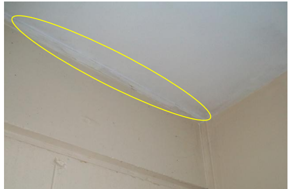
Photo 4: Separation along the roof and wall junctions
