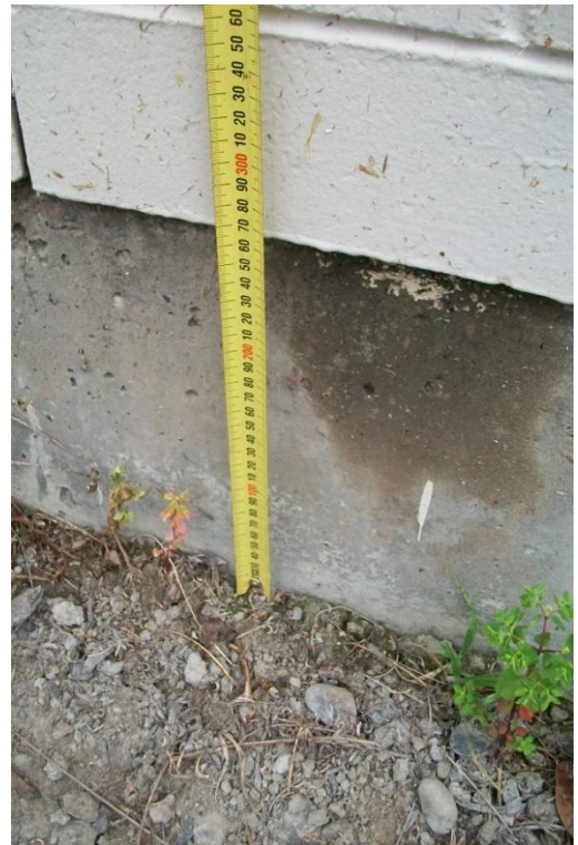
Photo 11: Strip footing 500mm deep with 300 mm above ground
