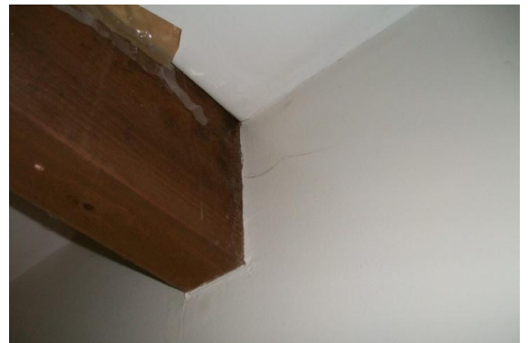
Photo 9: Plasterboard cracking around the timber roof beams
