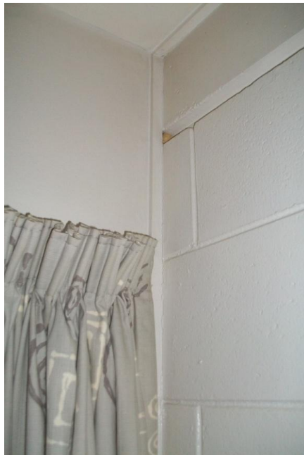
Photo 7: Top of the concrete masonry walls and transition to concrete bond beam
