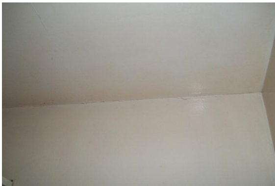
Photo 11: Wall ceiling junction separation
