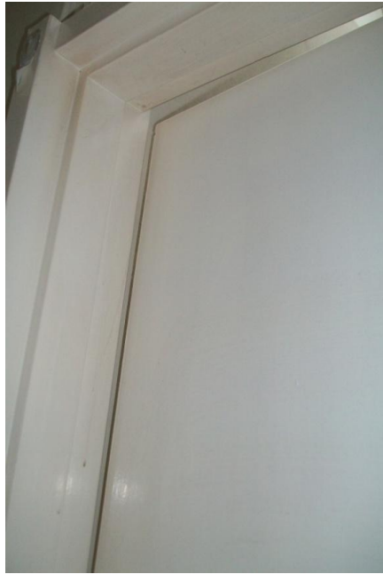
Photo 5: Door Frame skew has caused the door pictured to jam.
