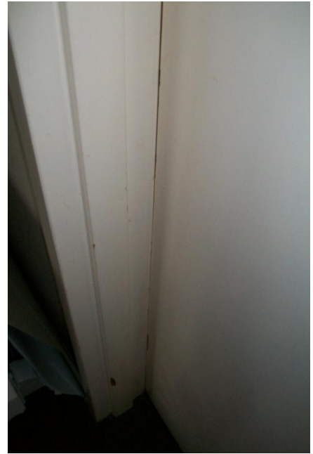
Photo 6: Door jamming over the bottom third of the door
