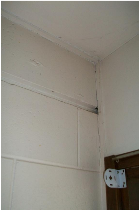
Photo 9: Wall junction separation
