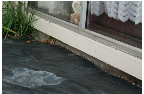
Photo 12: Separation between the the window framing and the timber cladding
