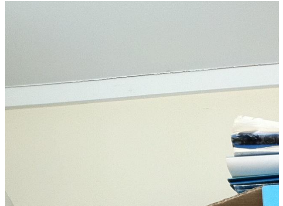
Photo 18: Cracking along ceiling lining & scotia
