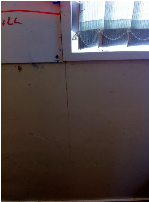
Photo 15: Vertical crack at gib joint below window corner
