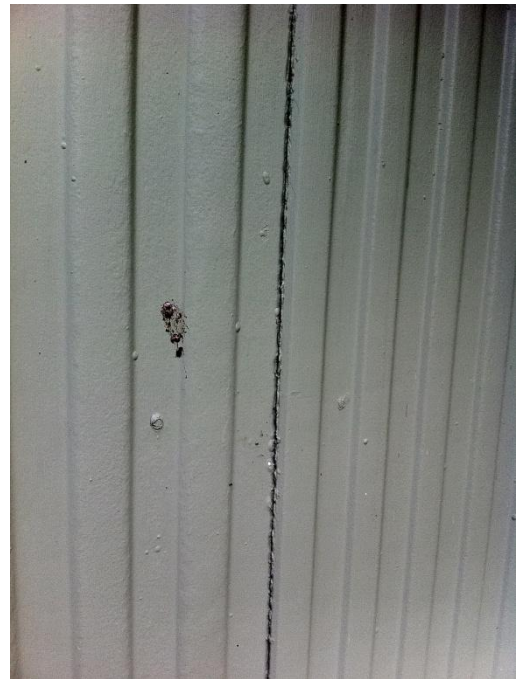
Photo 8: Crack in timber exterior cladding joint
