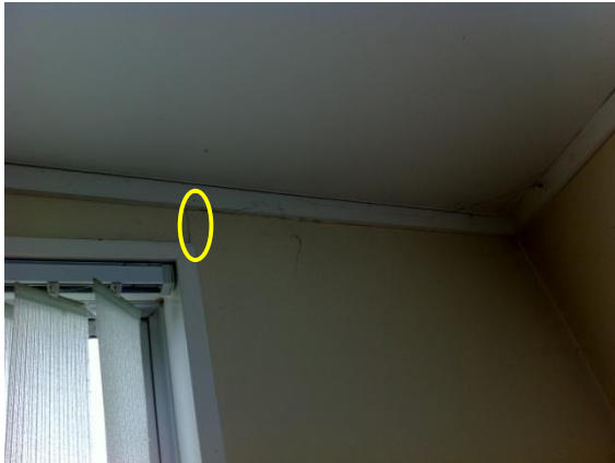
Photo 17: Small vertical cracks at upper window corners 2
