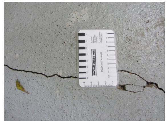
Photo 8: Close up view of 1.5mm crack from photo 7
