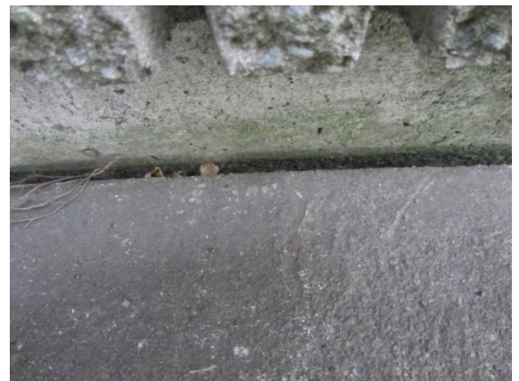
Photo 12: Close up of edge of pavement showing separation away from the structure
