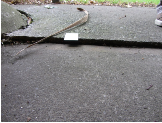
Photo 16: Close up of settled pavement from photo 16
