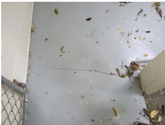
Photo 7: Entrance to the men's toilet showing 1.5mm crack
