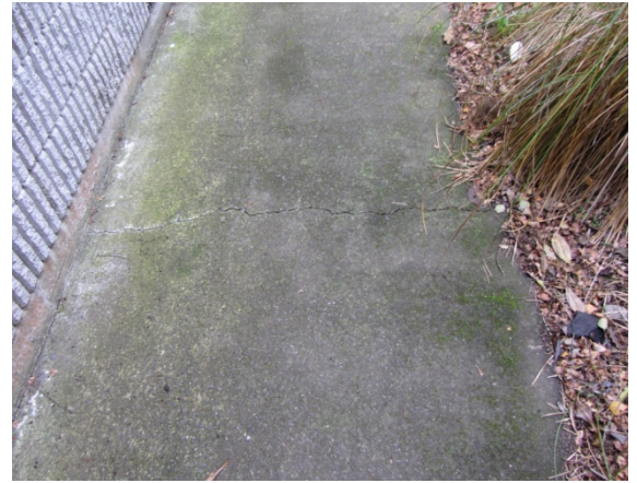
Photo 17: crack in the front of the toilet block (North Side)
