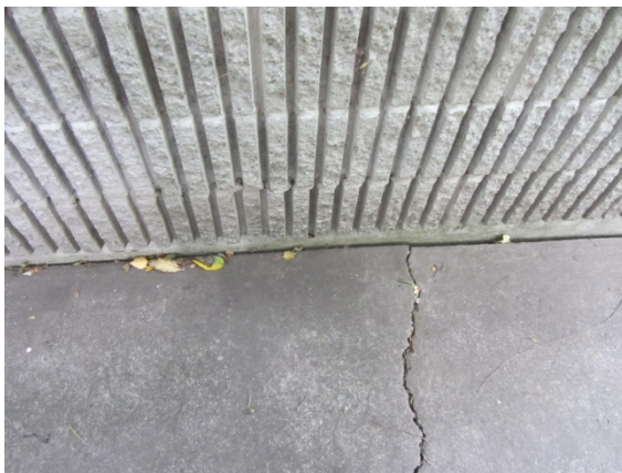
Photo 11: Pavement leading up to men's toilet showing crack.
