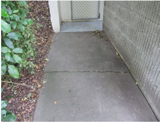
Photo 13: Same crack as found in photo 1, showing its full length
