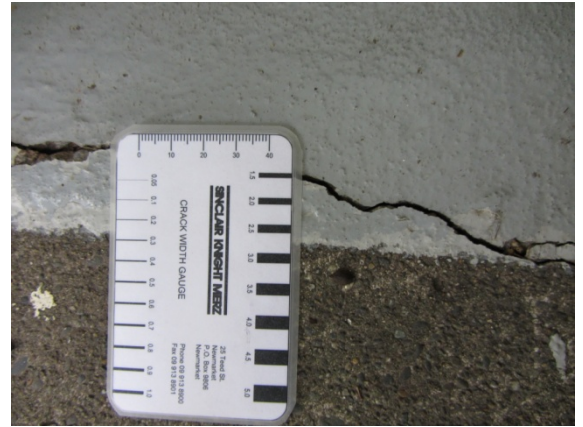
Photo 10: close up of 1.5mm crack in photo 9
