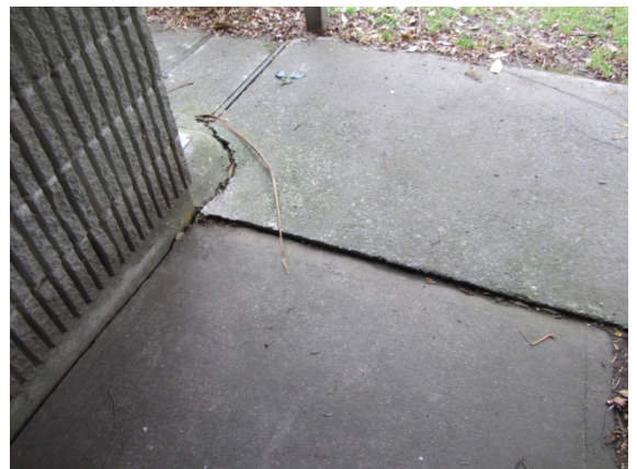
Photo 15: Mens toilet pavement showing the settlement, and the small trip hazard
