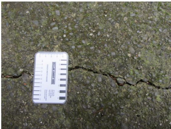
Photo 18: Close up of crack found in photo 18
