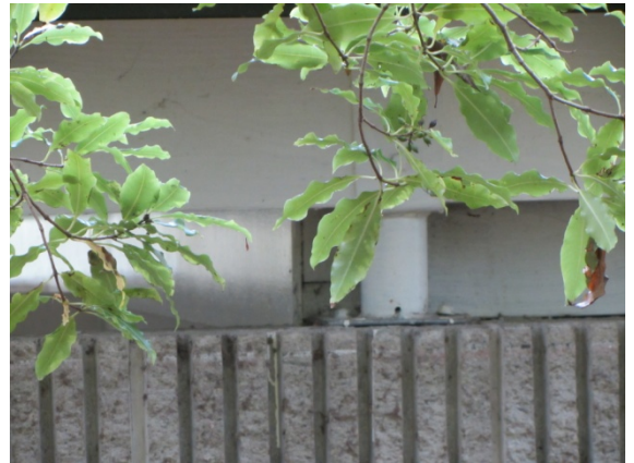
Photo 4: 100mm proud steel tube connecting the timber frame roof to the masonry walls
