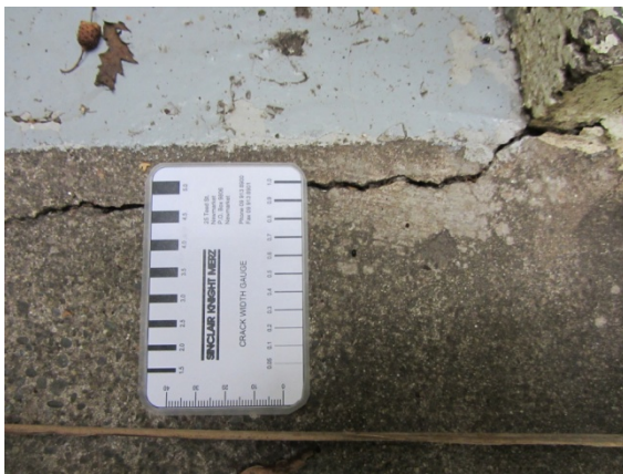
Photo 14: Close up of crack found in photo 14
