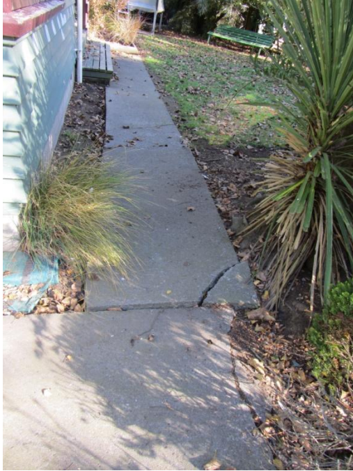
Photo 9: Damage to Pathway on North Side of Dwelling
