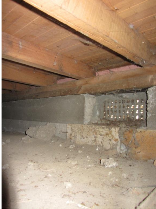
Photo 69: View of subfloor concrete perimeter ring beam.
