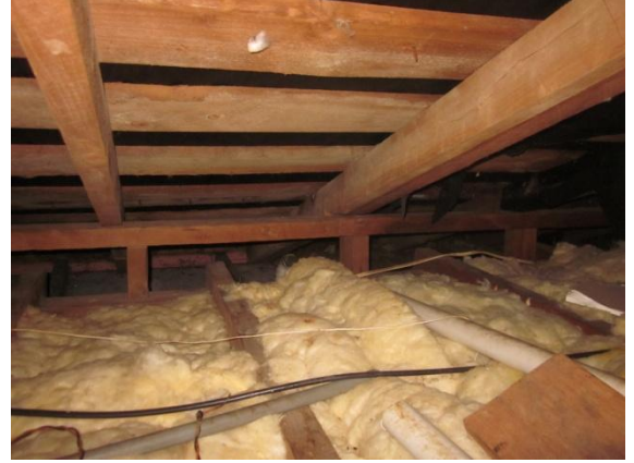
Photo 74: View of rafters and flat purlins at the roof.
