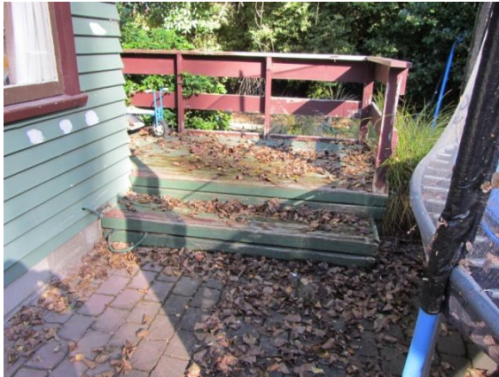
Photo 11: Northern Deck has Pulled Away from House Structure
