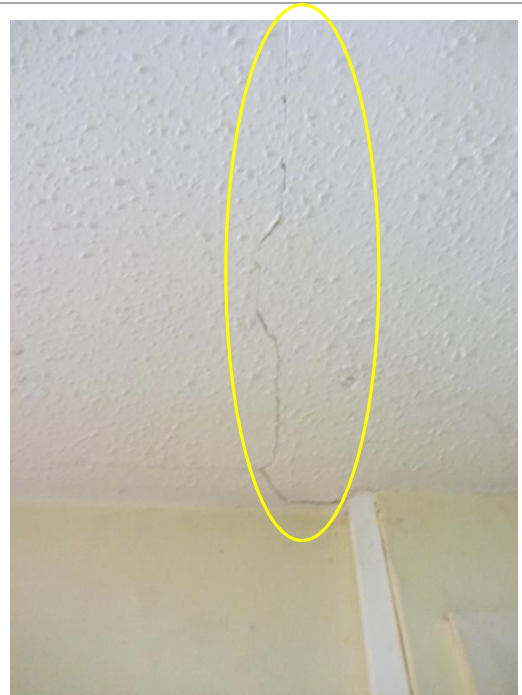
Photo 42: Cracking to Ceiling Lining
