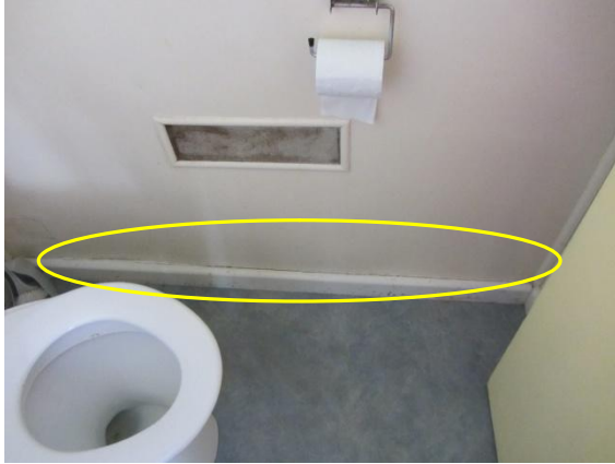
Photo 65: Cracking along Wall Lining and Scotia Joint
