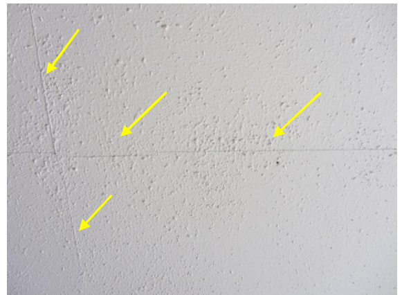
Photo 52: Hairline Cracking along Ceiling Lining Joints
