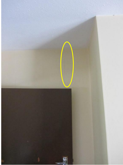
Photo 29: Hairline Cracking along Wall Lining Joint on East Wall near South Corner
