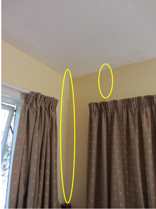
Photo 53: Cracking along Wall Lining Joint in South-West Corner and above Window
