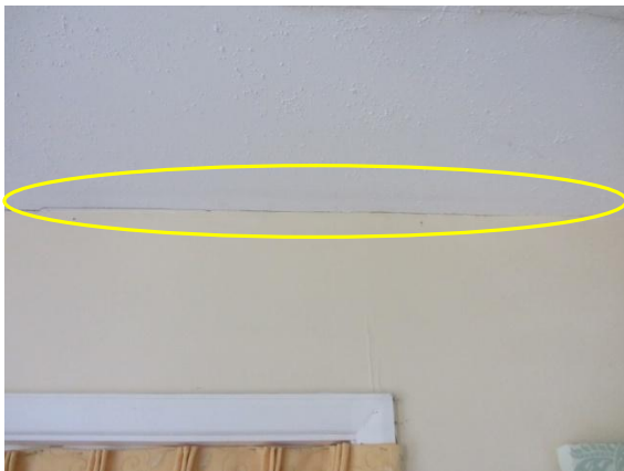
Photo 25: Hairline Cracking along Wall and Ceiling Lining Joint
