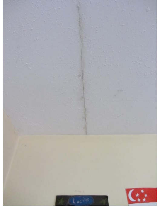
Photo 24: Hairline Cracking along Ceiling Lining
