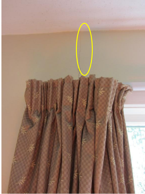
Photo 45: Hairline Cracking along Wall Lining Joint above Window
