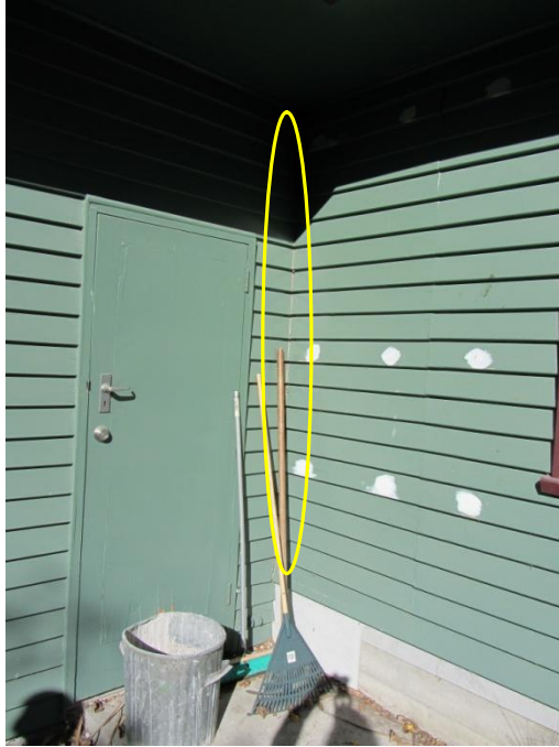
Photo 5: Hairline Cracking along Cladding Joints
