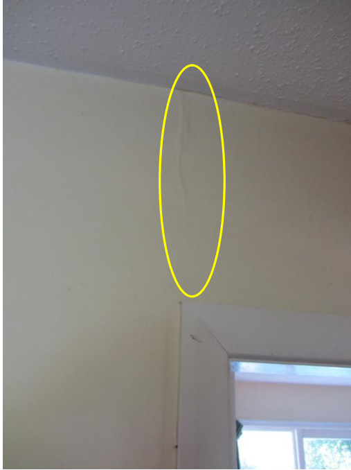
Photo 43: Hairline Cracking to Wall Lining Joint above Doorway (Typical)
