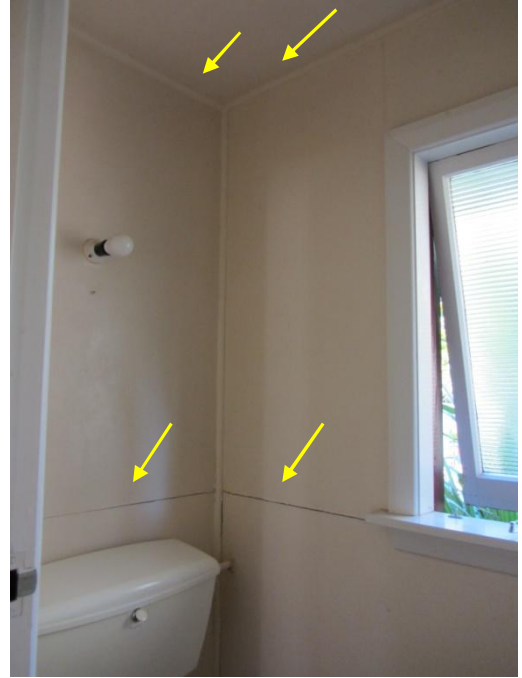
Photo 62: Cracking along Wall Lining Joints in Toilet
