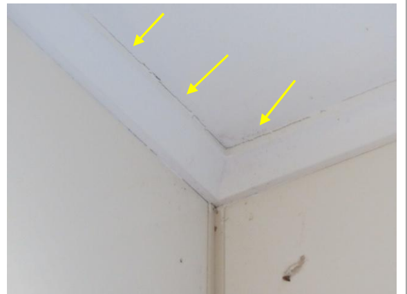
Photo 68: Hairline Cracking along Ceiling Lining and Scotia Joint
