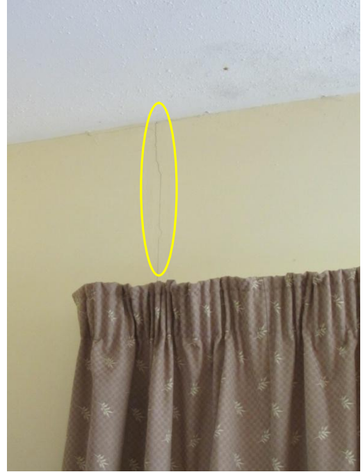
Photo 54: Hairline Cracking along Wall Lining Joint above Window (Typical)
