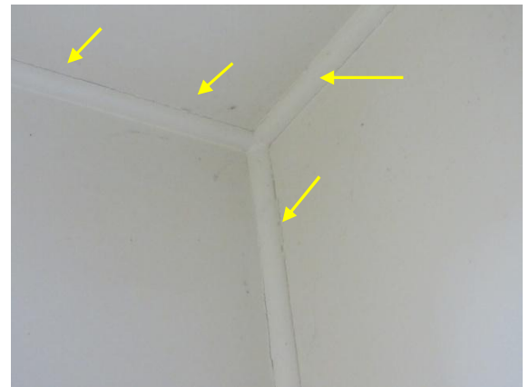
Photo 64: Hairline Cracking along Ceiling Lining and Scotia Joint and along Wall Lining and Timber Trim Joint
