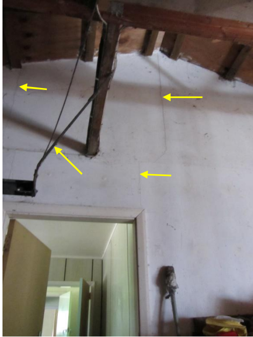
Photo 31: Cracking along Wall Lining Joints in Garage on East Wall
