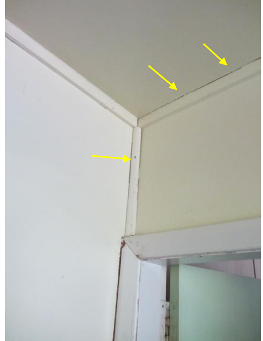
Photo 34: Cracking along lining and scotia joints and lining and timber trim joints
