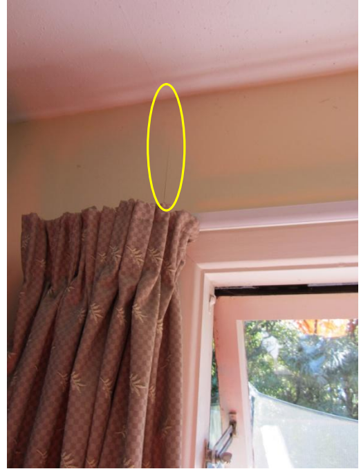
Photo 50: Hairline Cracking along Wall Lining Lining Joint above Window
