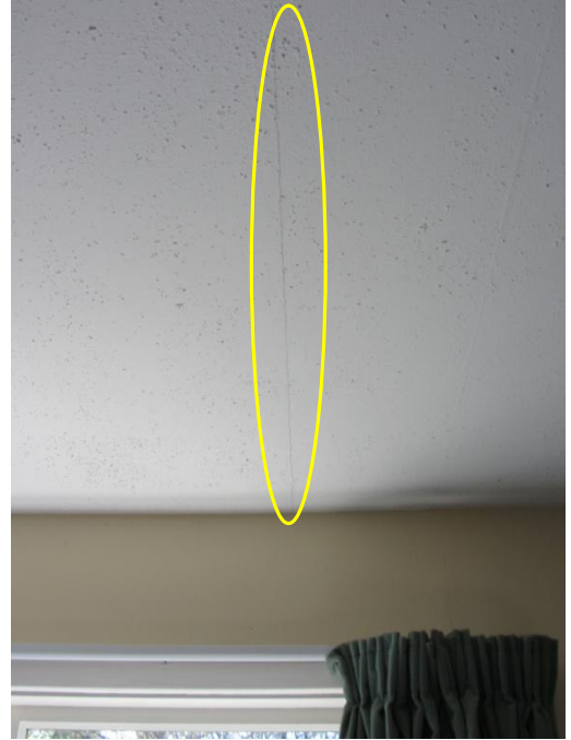
Photo 22: Hairline Cracking along Ceiling Lining Joint above East Window
