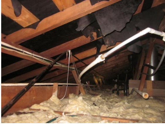
Photo 73: View of roof trusses.
