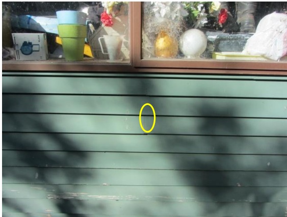
Photo 3: Cracking along Weatherboard Joints
