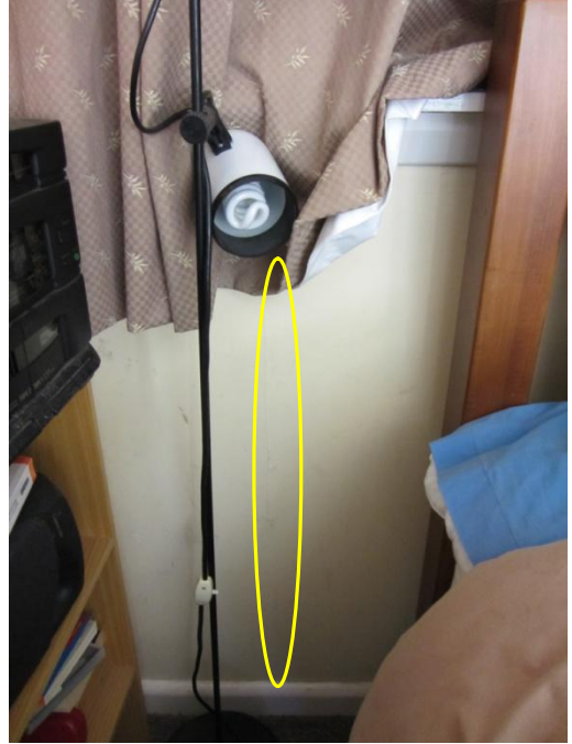
Photo 60: Hairline Cracking along Wall Lining Joint under South Wall Window
