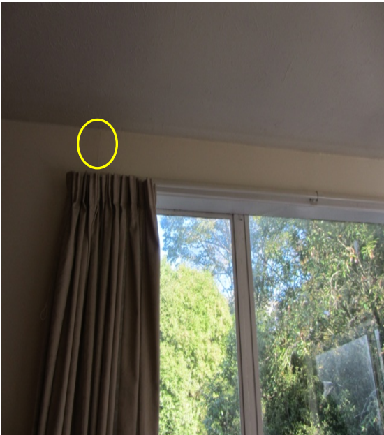
Photo 57: Hairline Cracking along Wall Lining Joints above Windows in Master Bedroom
