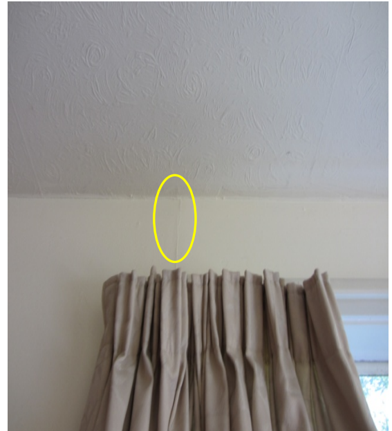
Photo 58: Close Up of Photo 57
