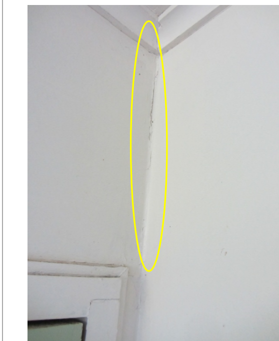
Photo 45: Hairline Cracking along Wall Lining Joint in NW Corner of Bathroom
