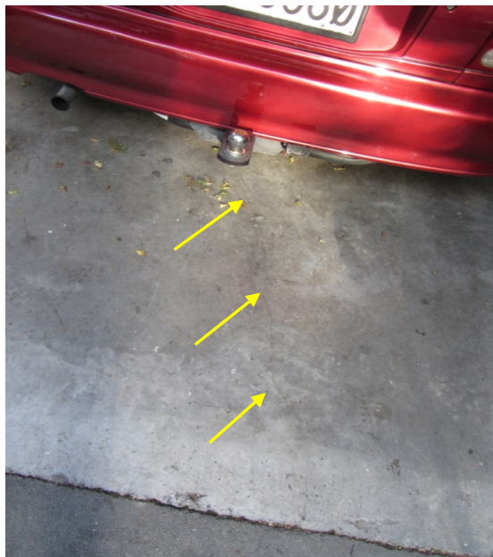
Photo 17: Hairline Cracking to Concrete Slab in Main Garage
