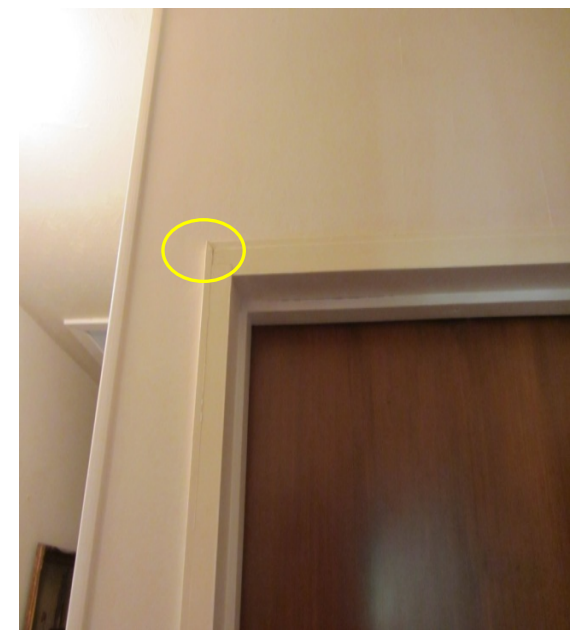
Photo 50: Hairline Cracking to Toilet & Bathroom Door Architrave Joints
