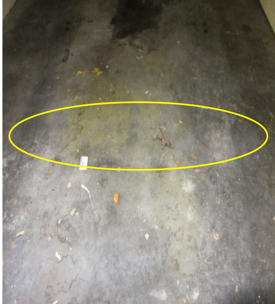
Photo 23: Hairline Cracking to Concrete Slab in NW Garage / Storage Room
