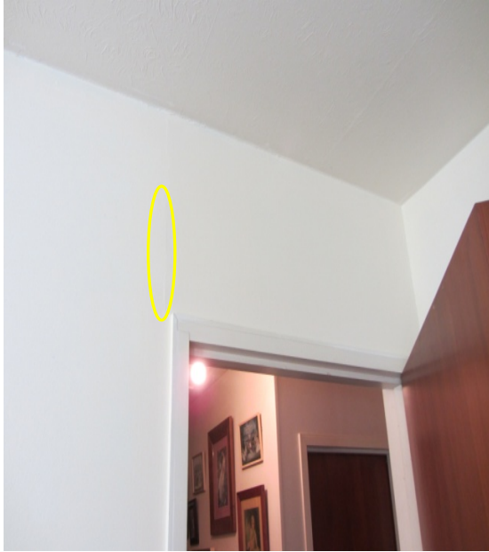
Photo 55: Hairline Cracking along Wall Lining Joint above Doorway in Master Bedroom
