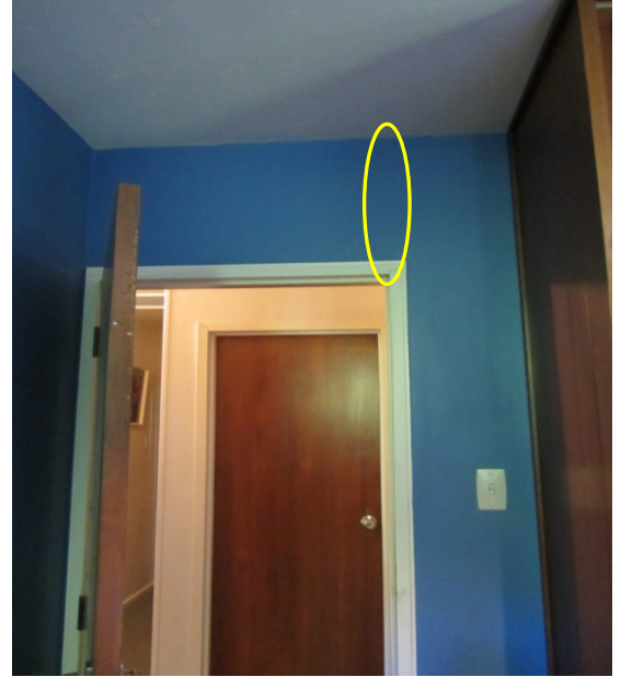
Photo 52: Hairline Cracking along Wall Lining Joint above Doorway in SW Bedroom
