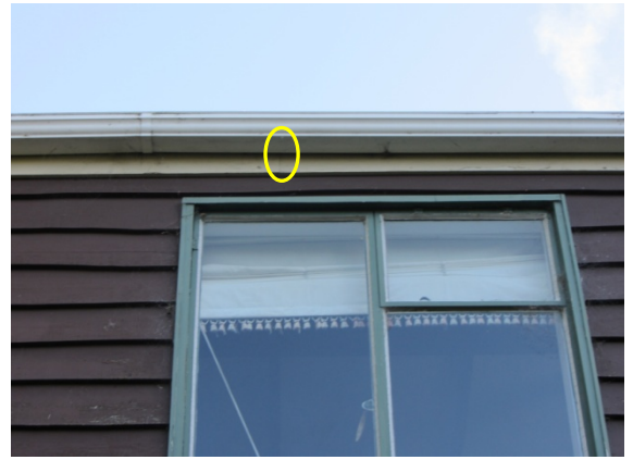
Photo 6: Hairline Cracking along Fascia Board Joints
