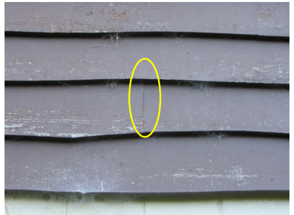
Photo 4: Hairline Cracking along Joints in External Cladding
