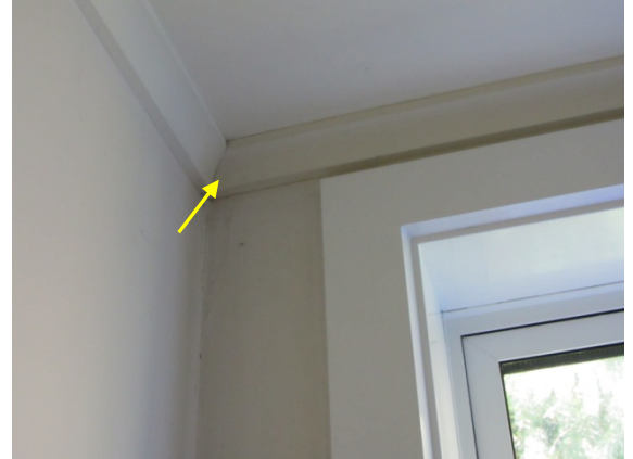
Photo 48: Hairline Cracking along Scotia and Wall Lining Joint
