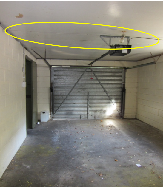
Photo 21: North-West Garage / Storage Room
