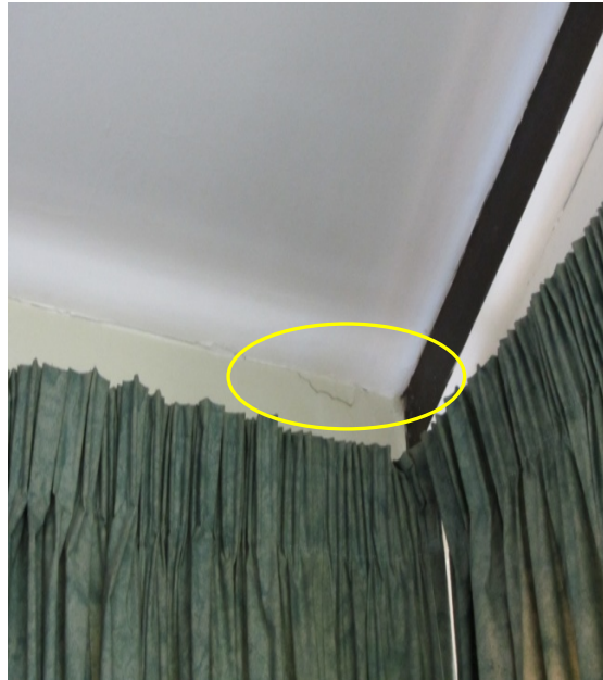
Photo 29: Hairline Cracking to Wall Lining in NE Corner
