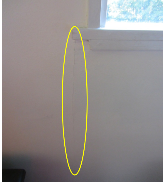
Photo 35: Hairline Cracking Present along Wall Lining Joint under South Wall Window
