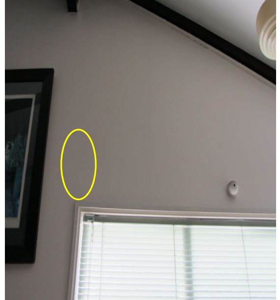
Photo 32: Hairline Cracking along Wall Lining Joint above Window
