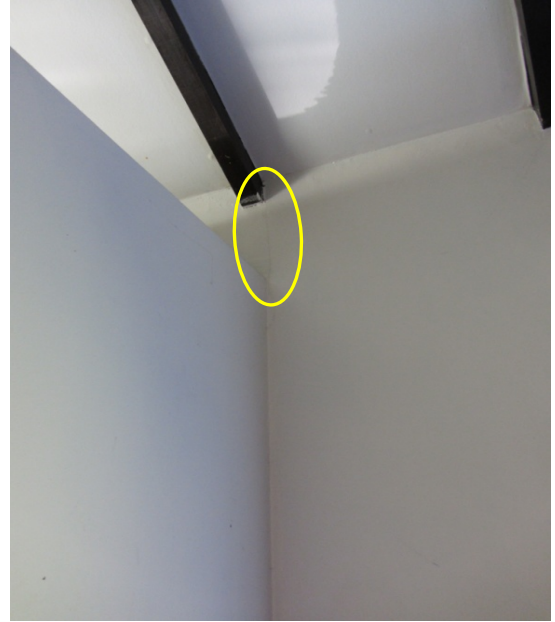
Photo 36: Hairline Cracking Present along Wall Lining Joint on South Wall above Kitchen Partition
