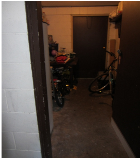
Photo 25: Continuation of Hairline Crack running N/S in Main Garage Floor Slab
