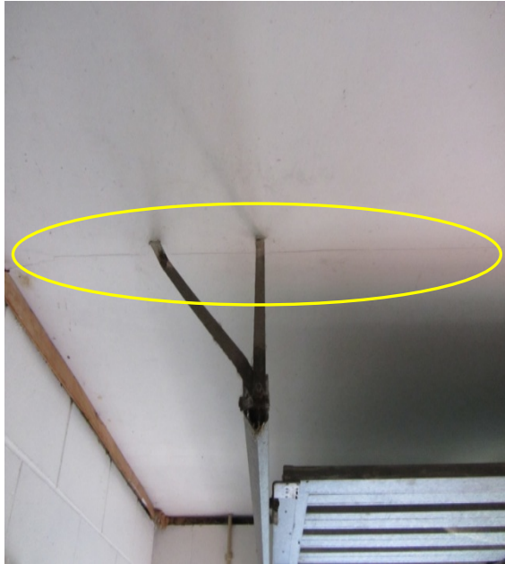
Photo 15: Hairline Cracking to Ceiling Lining Joint in Main Garage
