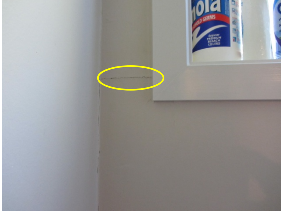
Photo 47: Hairline Cracking along Wall Lining Joint Each side of Toilet Window
