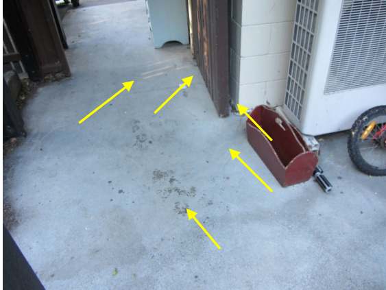
Photo 11: Hairline Cracking to Concrete Patio in North-East Corner
