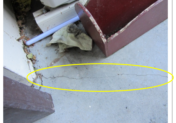
Photo 12: Close Up of Photo 11
