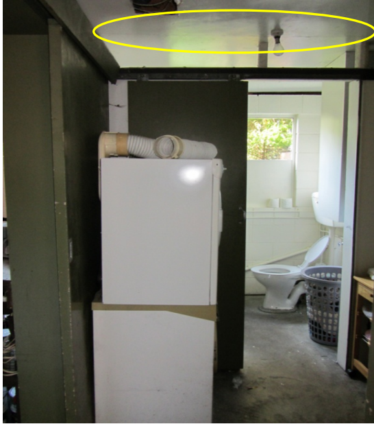
Photo 19: Hairline Cracking to Ceiling Lining Joints in Laundry
