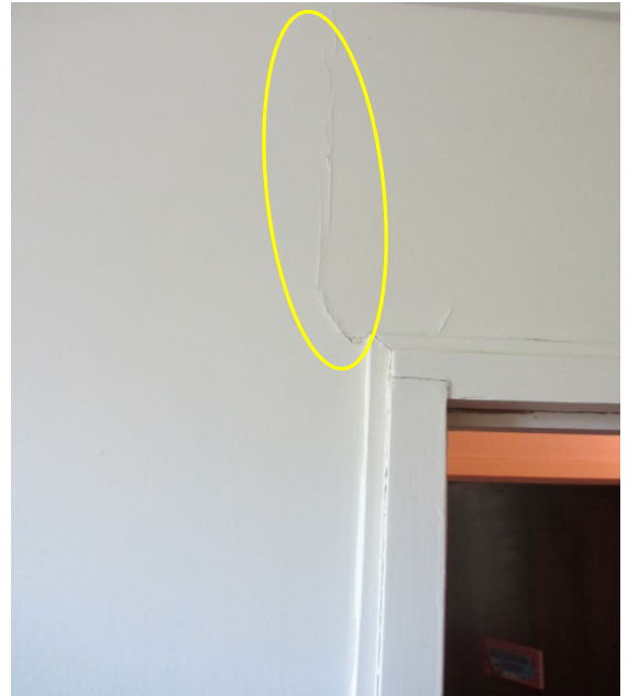
Photo 44: Hairline Cracking to Wall Lining above Bathroom Doorway
