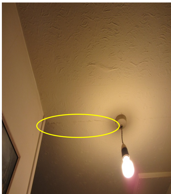
Photo 41: Hairline Cracking to Ceiling Lining in SW Corner of Hallway
