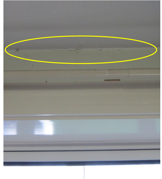
Photo 30: Hairline Cracking Present along Wall and Ceiling Lining Joint on North Wall
