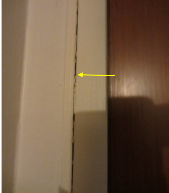
Photo 39: Gaps between Door Architrave and Door Jamb on East Wall have Opened Up
