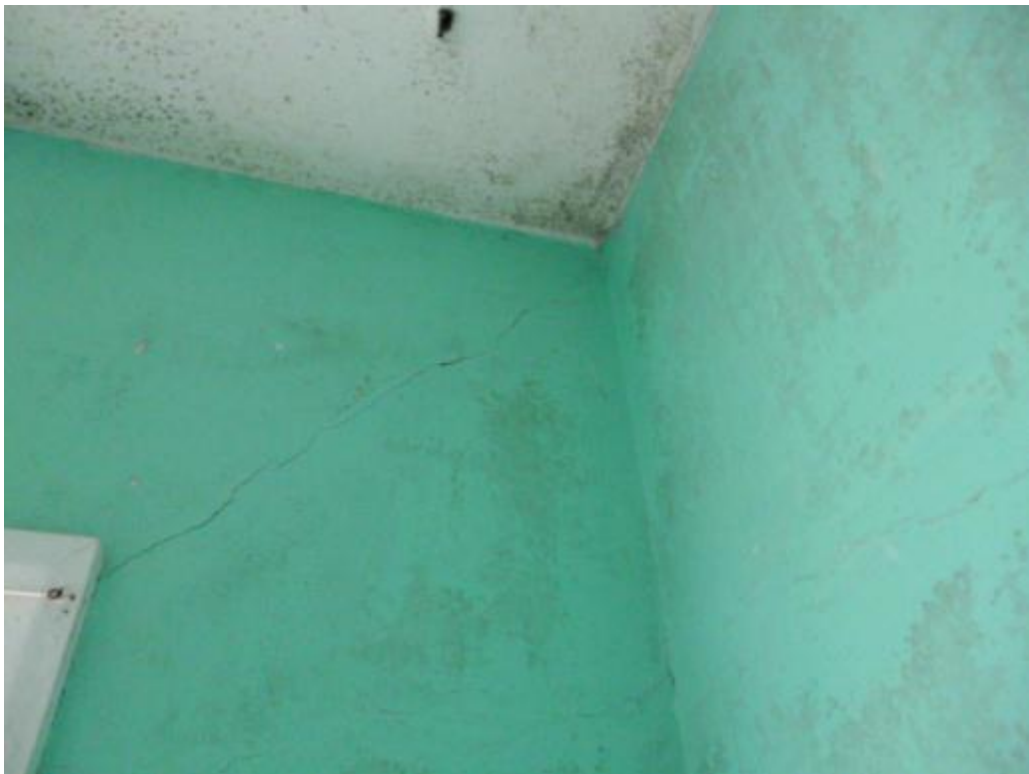
Photograph 7 Cracking in foundation
