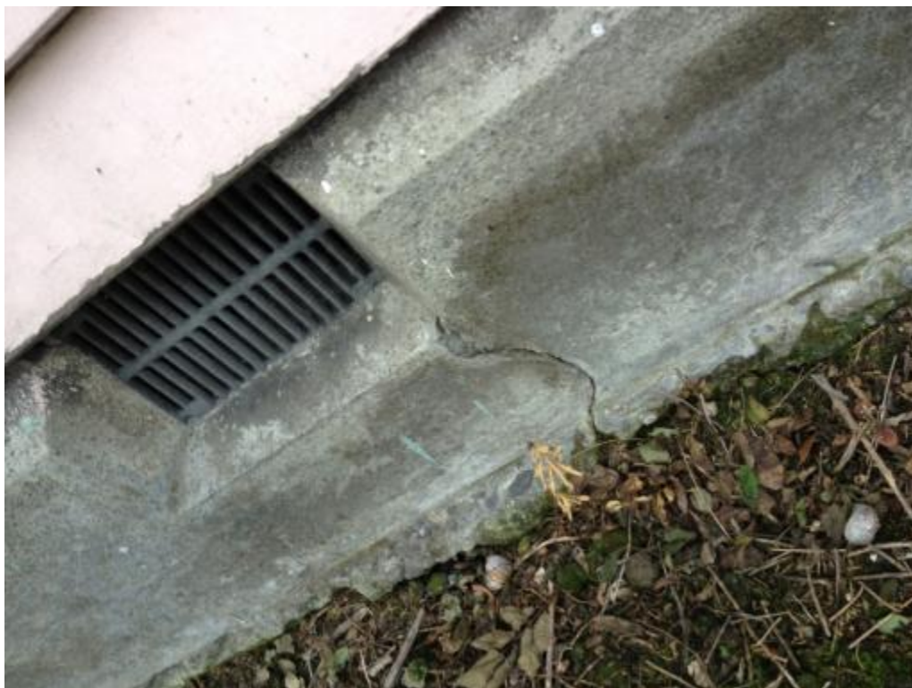
Photograph 5 Vertical cracking in foundation.
