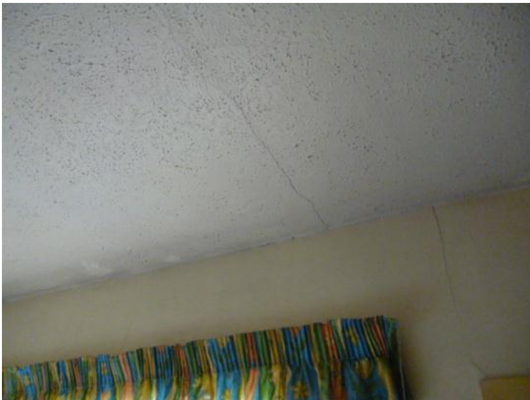
Photograph 12 Cracking in ceiling
