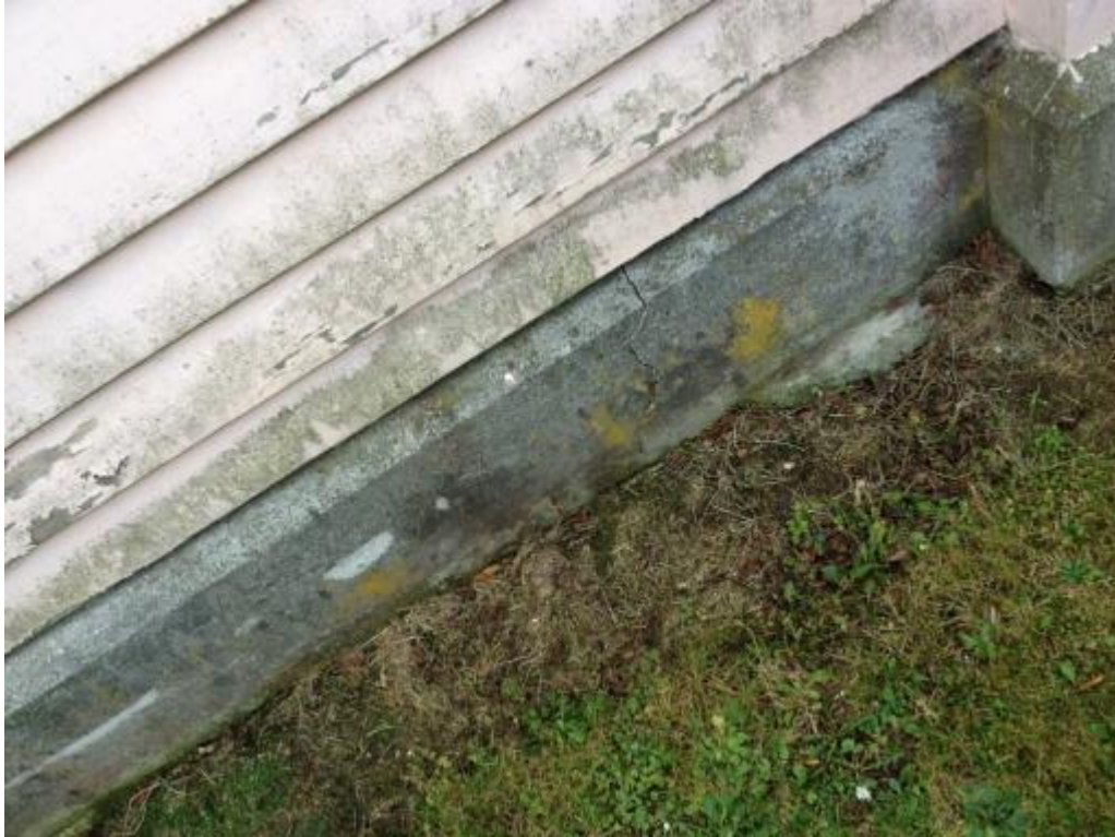
Photograph 7 Cracking in foundation
