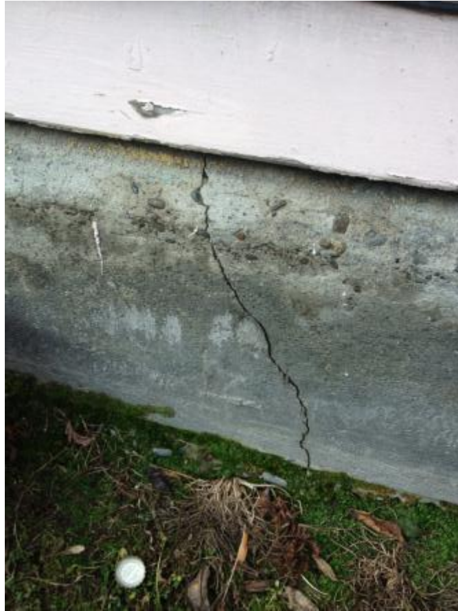
Photograph 5 Vertical cracking in foundation.
