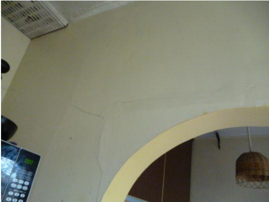
Photograph 11 Cracking in plasterboard.
