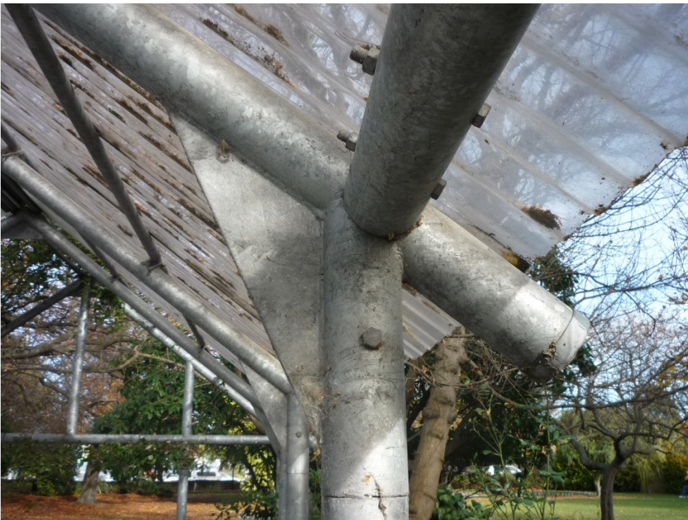
Photo 2: Typical roof beam columns joint.
