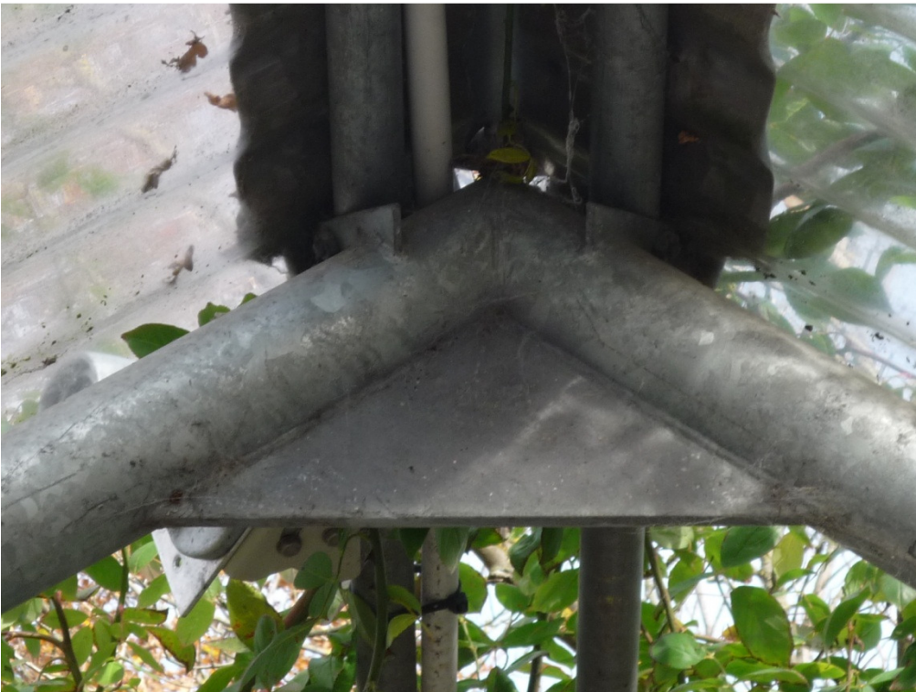
Photo 3: The apex joint.
