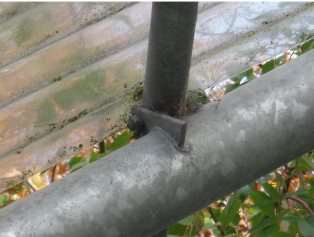
Photo 4: View of purlin connection.
