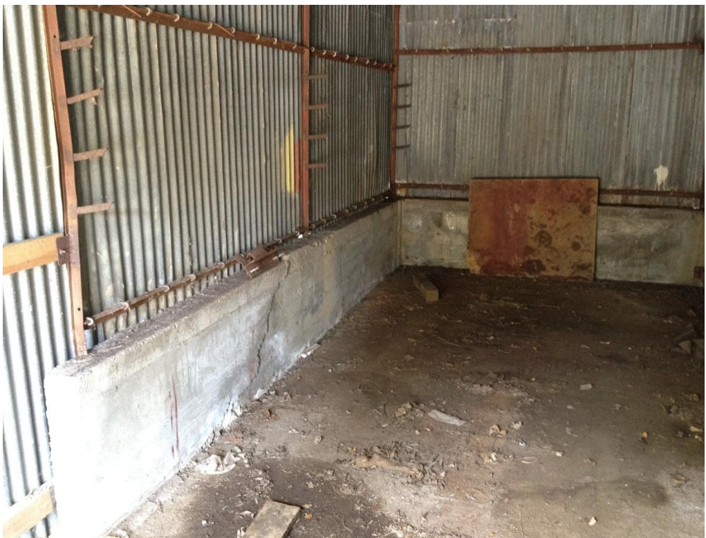
Photograph 2: Concrete perimeter surround with existing concrete crack
