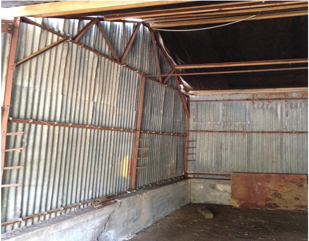
Photograph 3: Steel framed structure with lightweight metal cladding connected into concrete perimeter
