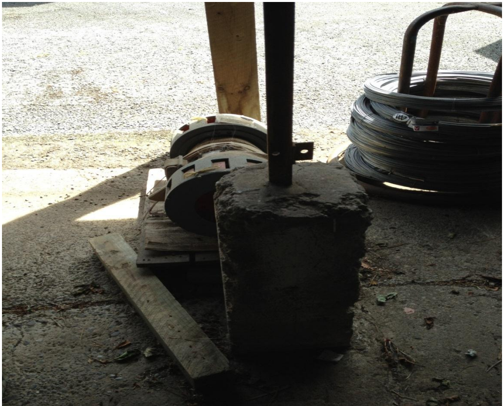
Photograph 5: T-sections posts set into concrete
