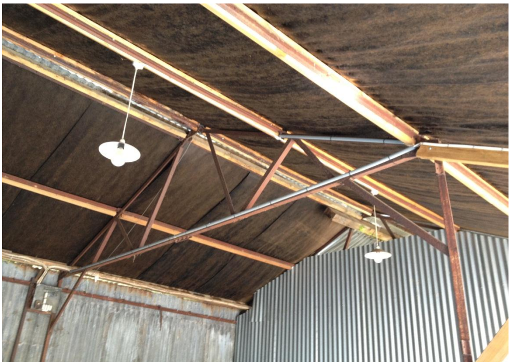
Photograph 4: Equal angel truss connected into T-section posts. Timber supports added to strengthen the structure previously
