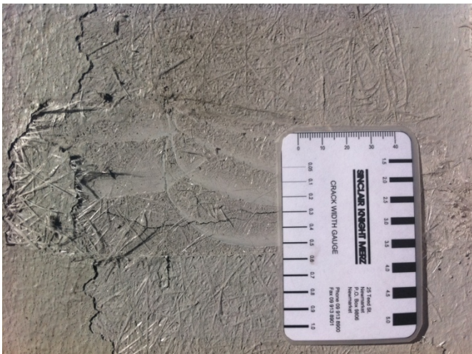
■ Figure 8 – Grandstand – cracking under fibreglass topping.
