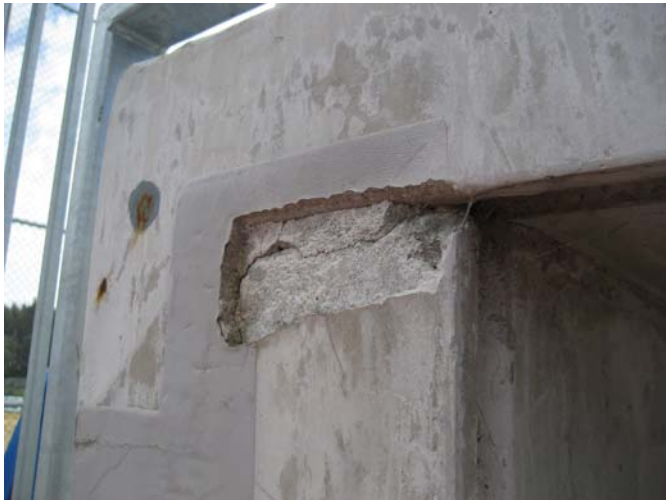
■ Figure 10 – Grandstand – Section of plastering has broken out damaging the waterproofing.
