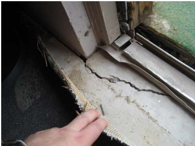
■ Figure 10 – Grandstand – Section of plastering has broken out damaging the waterproofing.
