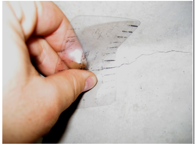
■ Figure 11 – Grandstand – Typical concrete wall cracking.
