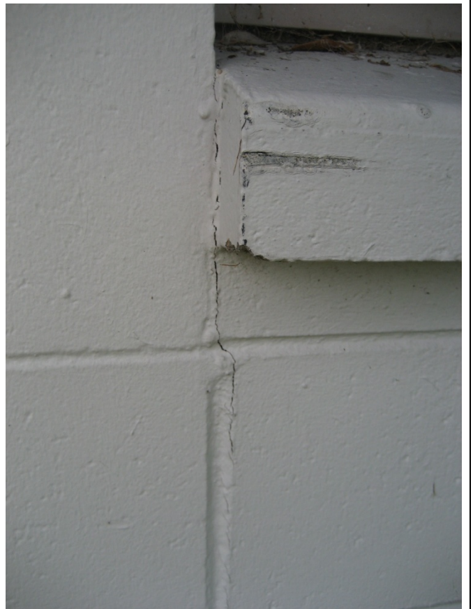
■ Figure 13 – Groundsmans Shed – Typical Blockwork cracking.
