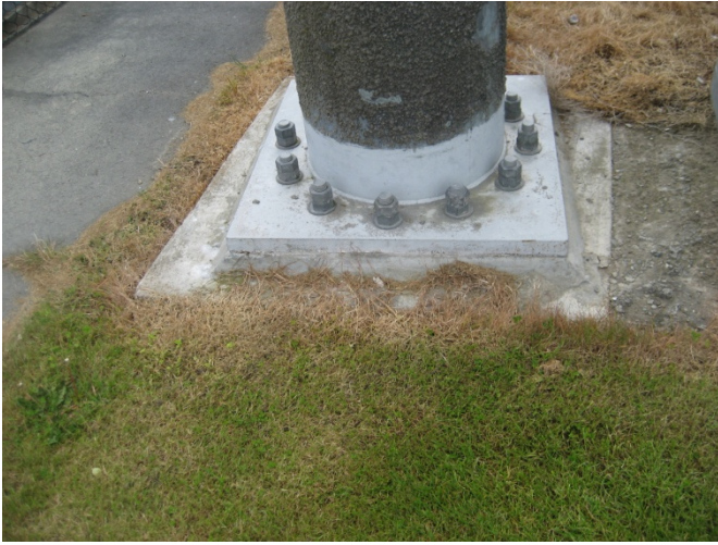
■ Figure 14 – Light Towers – Typical Base detail, some require relevening.
