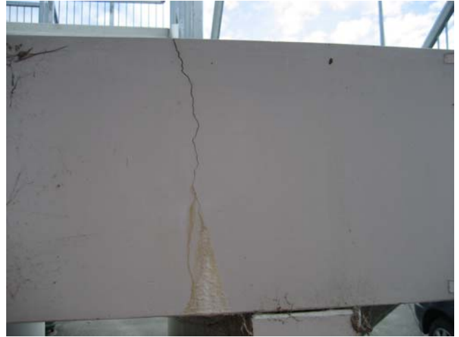
■ Figure 7 – Grandstand – Cracking of stair landing.
