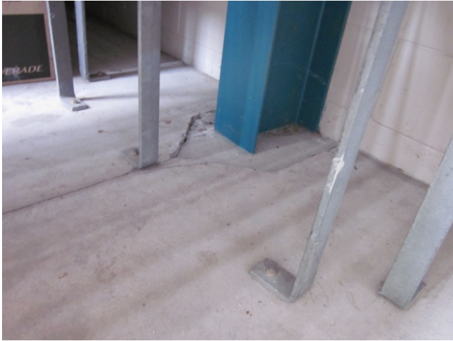
■ Figure 6 – Complex – Differential movement of column base and ground floor slab.
