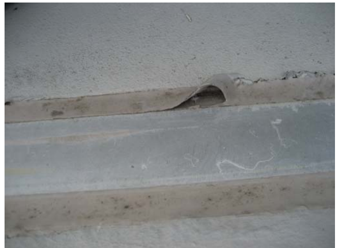
■ Figure 9 – Grandstand – Damage to separation joint at Softball Complex.
