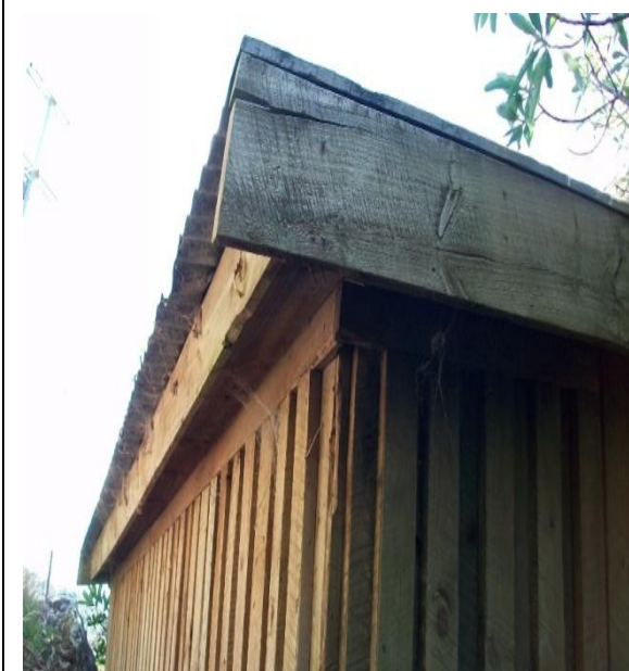
Photo 3: Crack in timber roof beam on the southeast corner
