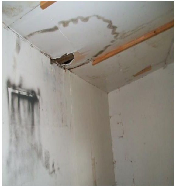
Photo 6: Water damage on the southern area of the ceiling noted due to sagging ceiling cladding panels.
