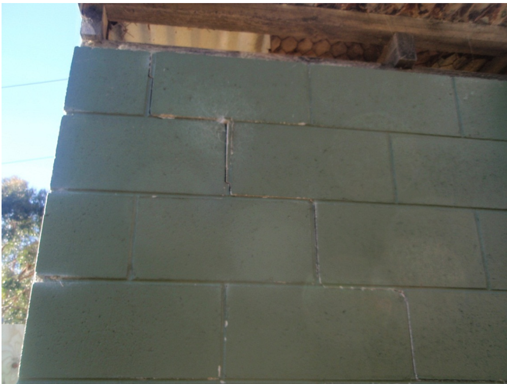
Cracked exterior wall at the rear of building
