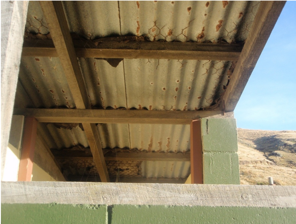
Corroded corrugated iron roofing
