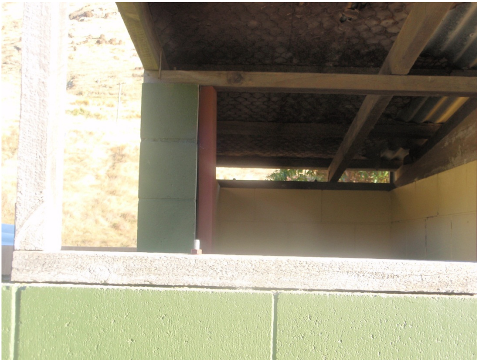
Roof timber framing to masonry walls connection
