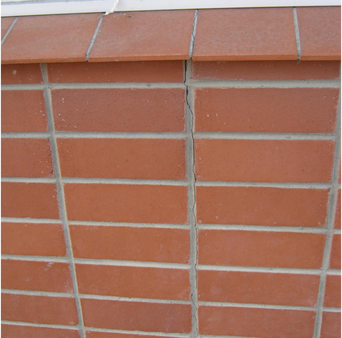
Typical crack at masonry mortar
