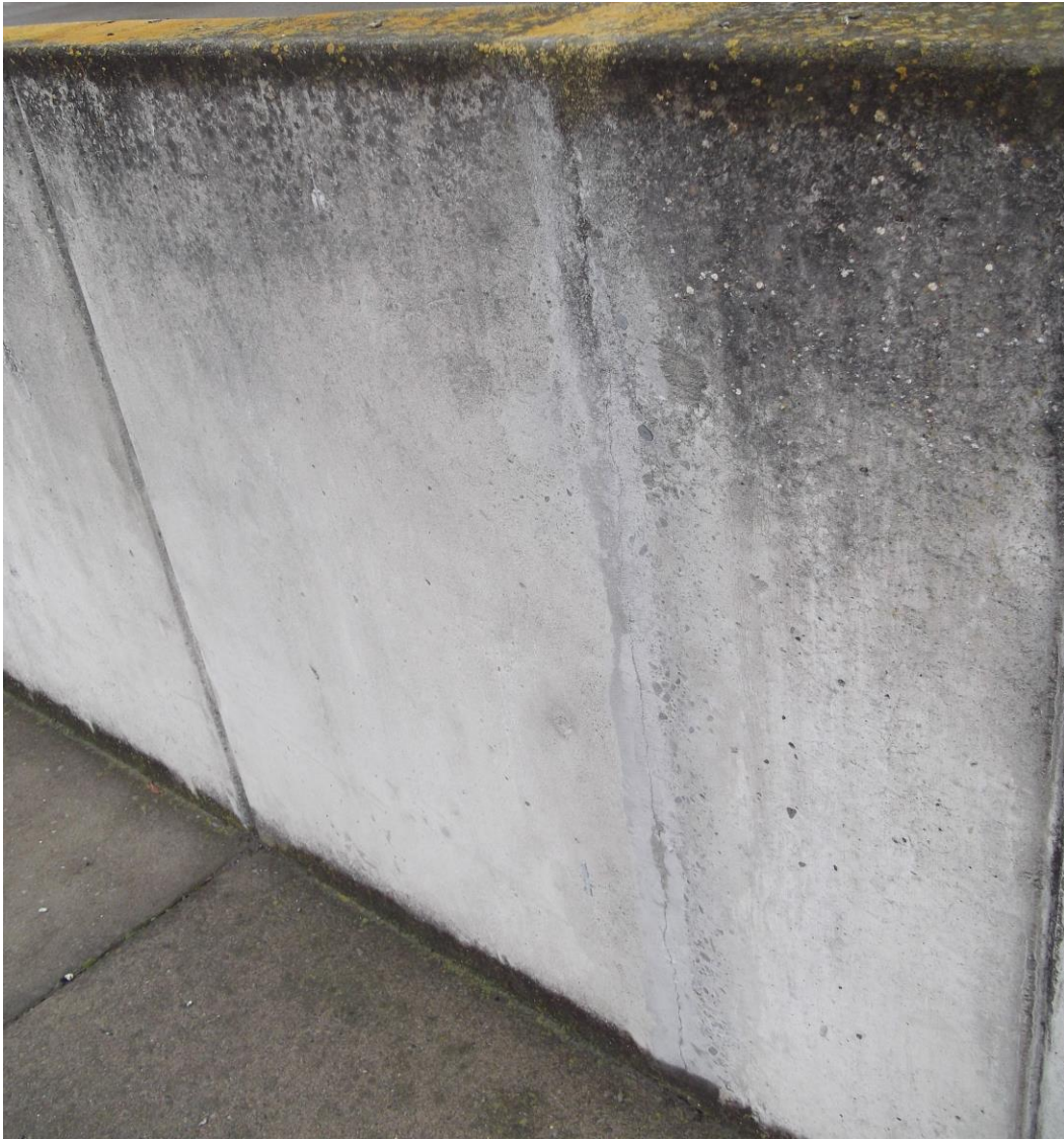
Typical minor cracking at retaining wall
