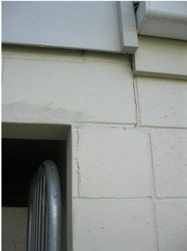
Photograph 5 Cracking to masonry walls at entrance to men's toilet.
