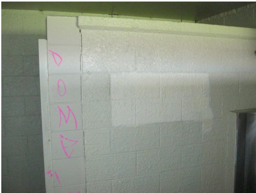
Photograph 5 Cracking to masonry walls at entrance to men's toilet.
