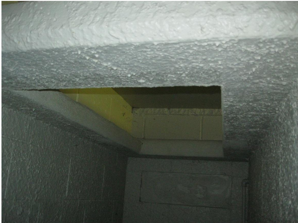
Photograph 7 Concrete panel capping the cubicle walls in men's toilet.
