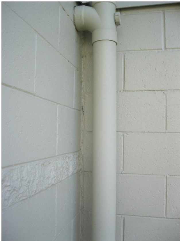
Photograph 8 Cracking to flexible seal.
