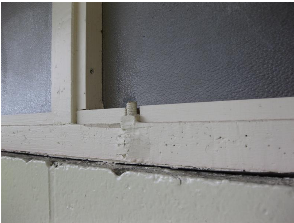
6. Weak window connection to masonry wall
