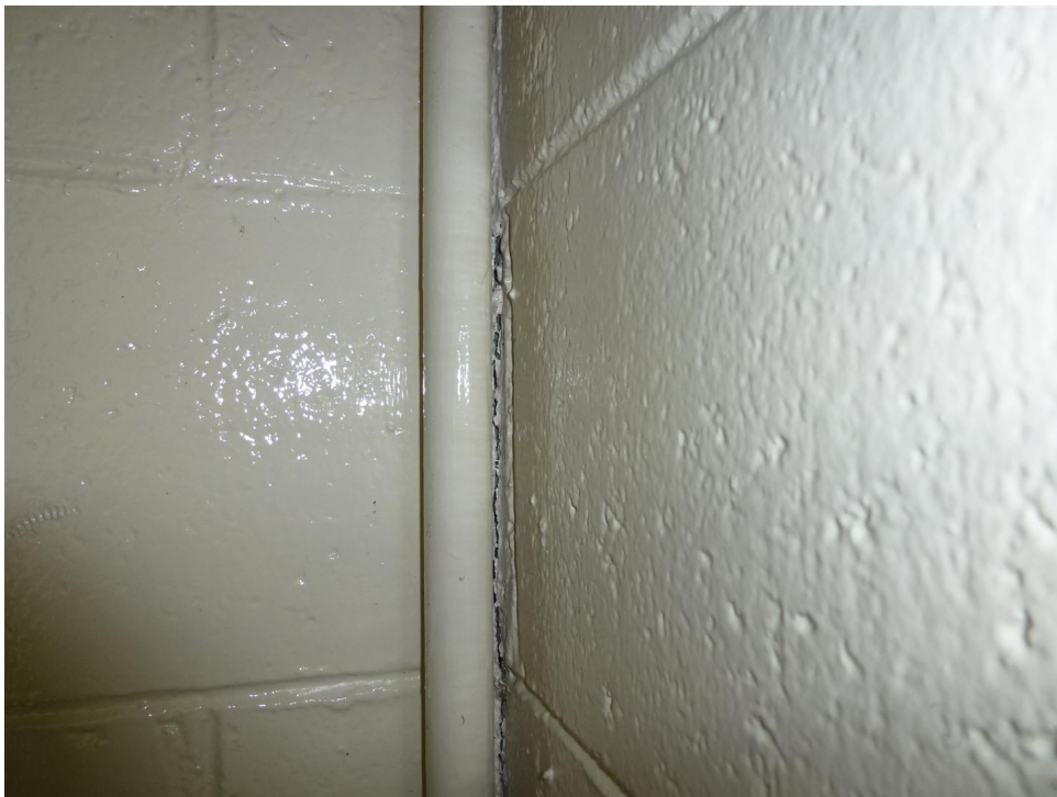
8. Moderate width wall crack requiring sealant
