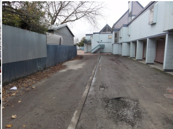
Heave and damage to driveway.
