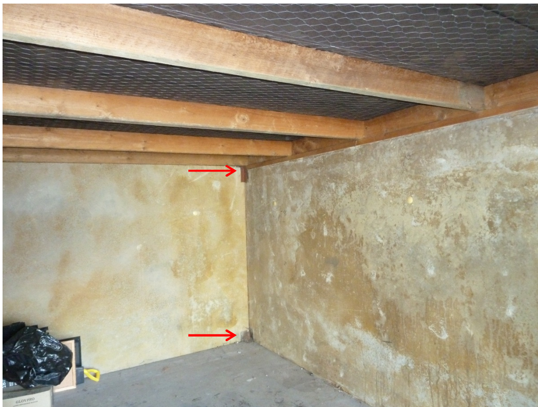
Photo 2: View of the interior of one of the garages. Welded steel plate connections have been indicated
