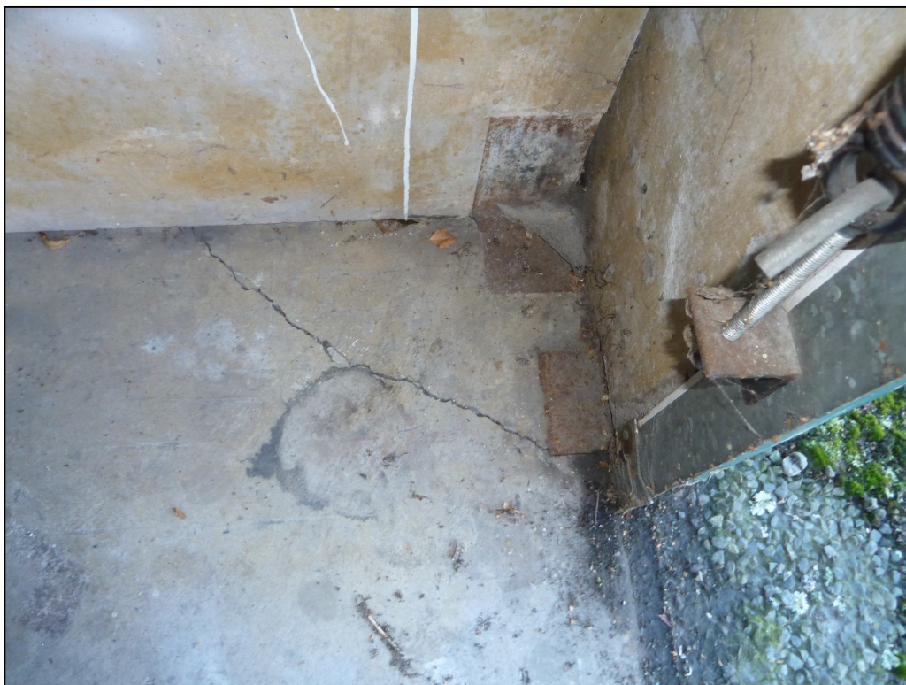
Photo 4: Typical cracking in corners of slabs
