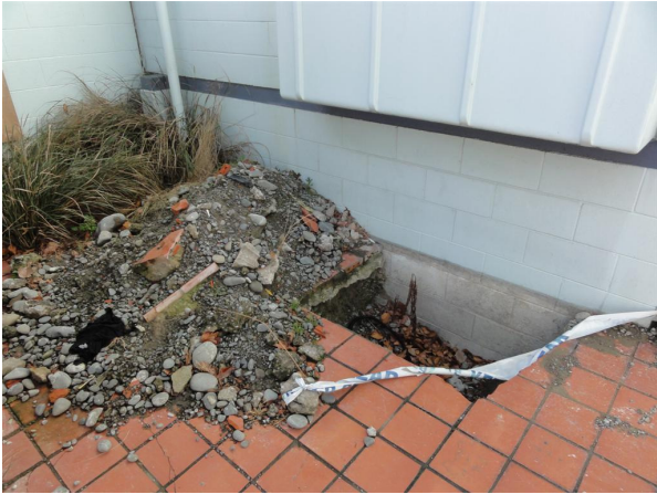
Open excavation showing rounded pit run.
