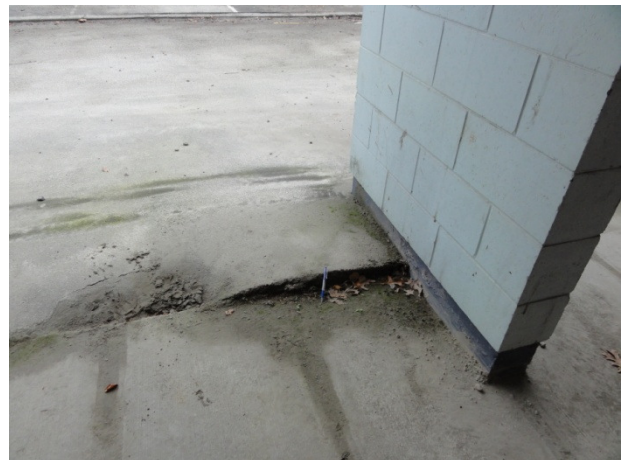
Ground Heave at footing adjacent to Unit 364
