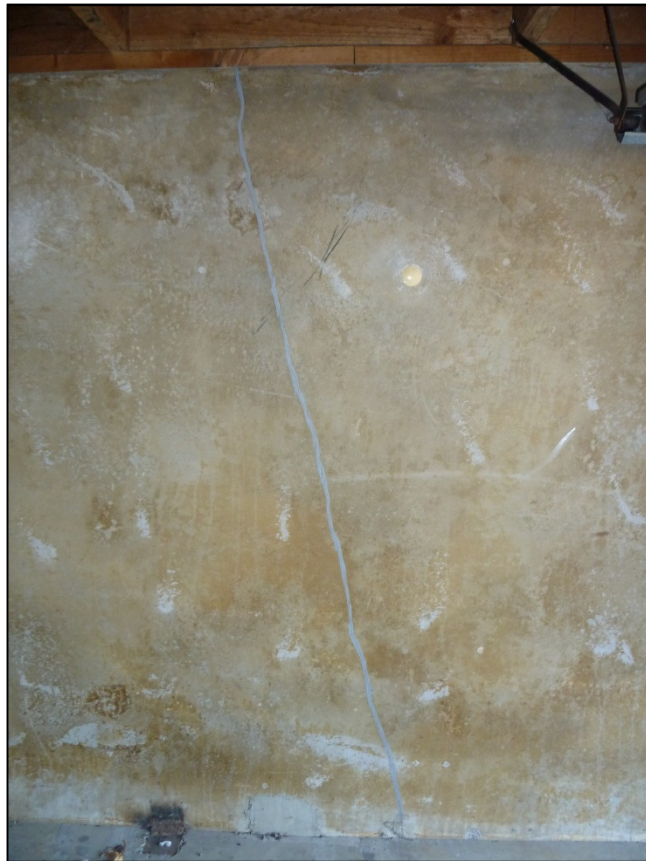
Photo 3: 1mm crack up the full height of one panel. The crack has been repaired/sealed
