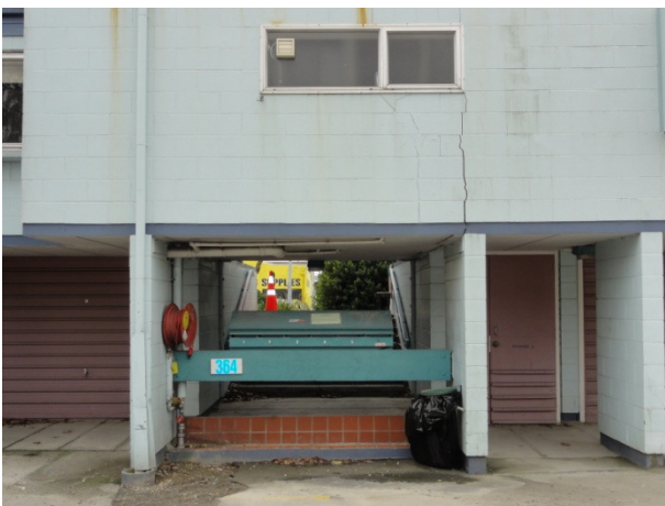
Structural Damage to 2 nd and 3 rd Storey at Unit 364
