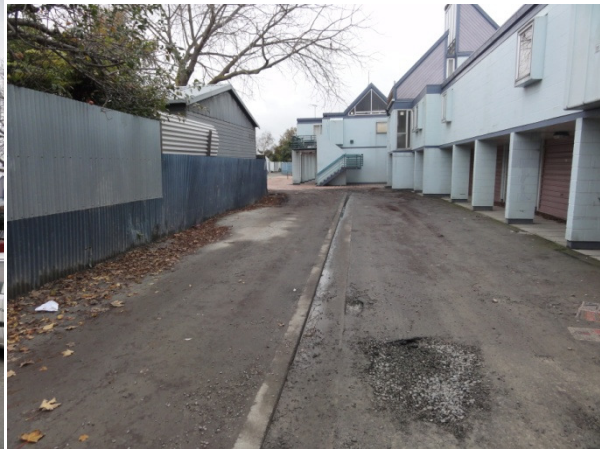
Heave and damage to driveway.
