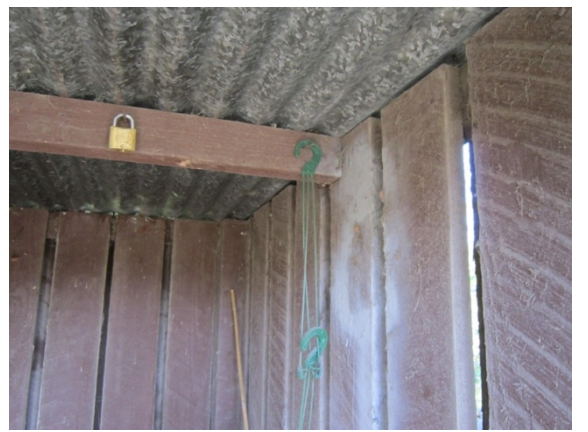
Photo 8: Timber ceiling element with corrugated sheeting
