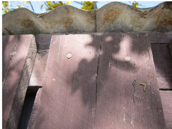
Photo 5: Splitting of timber elements along the grain (typical)
