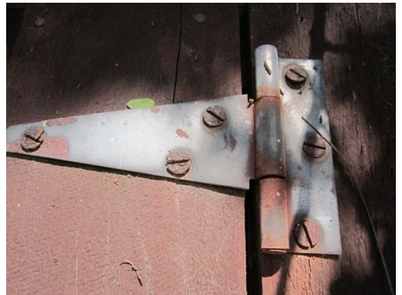
Photo 6: Rusting of steel elements (typical)
