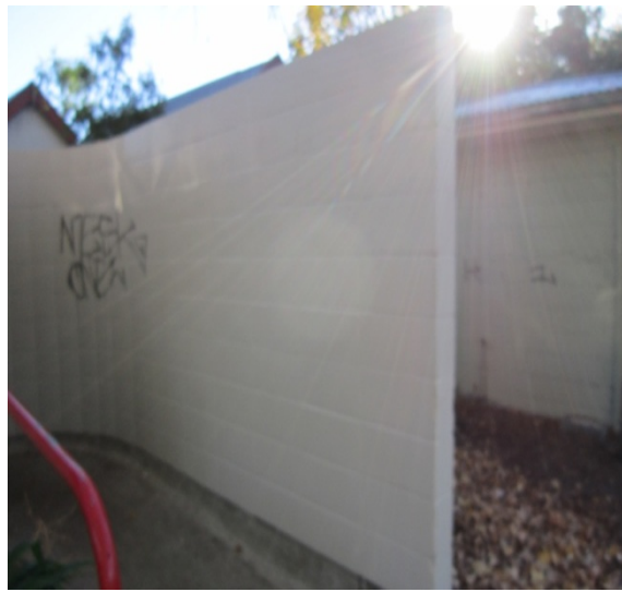
Photo 5: East wall at east toilet entrance
