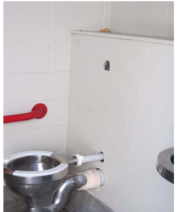
Photo 12: West toilet interior layout.
