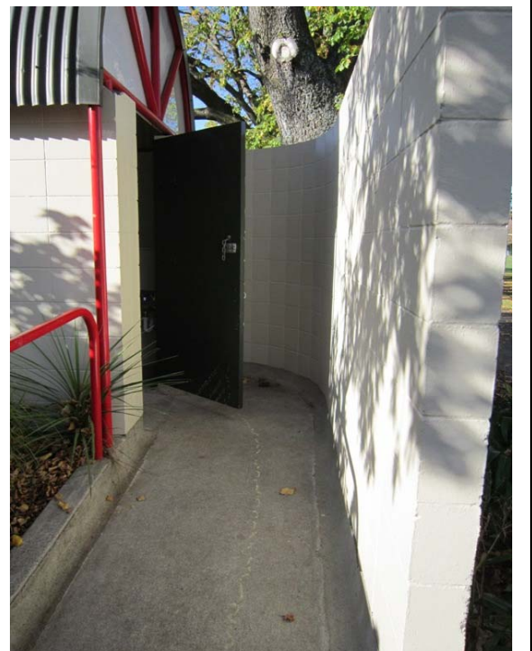
Photo 8: West toilet entrance.
