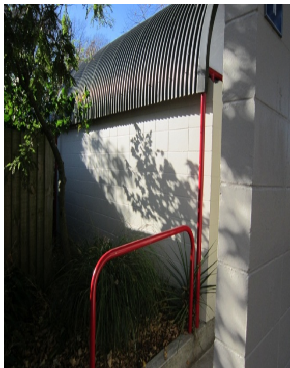
Photo 7: Corrugated metal roof sheeting.
