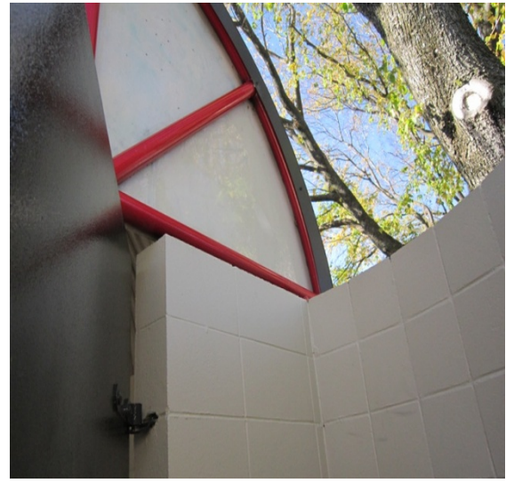
Photo 10: West toilet entrance wall layout.
