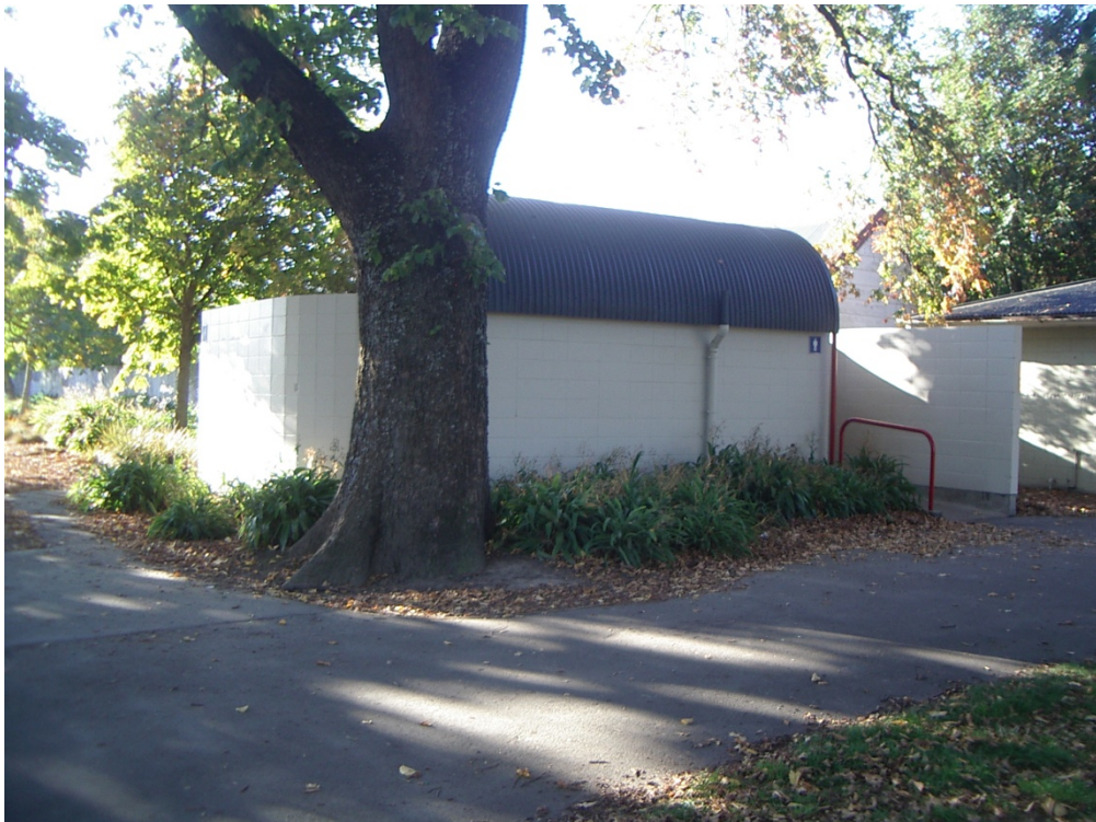
■ Figure 10 Overview of public toilets
