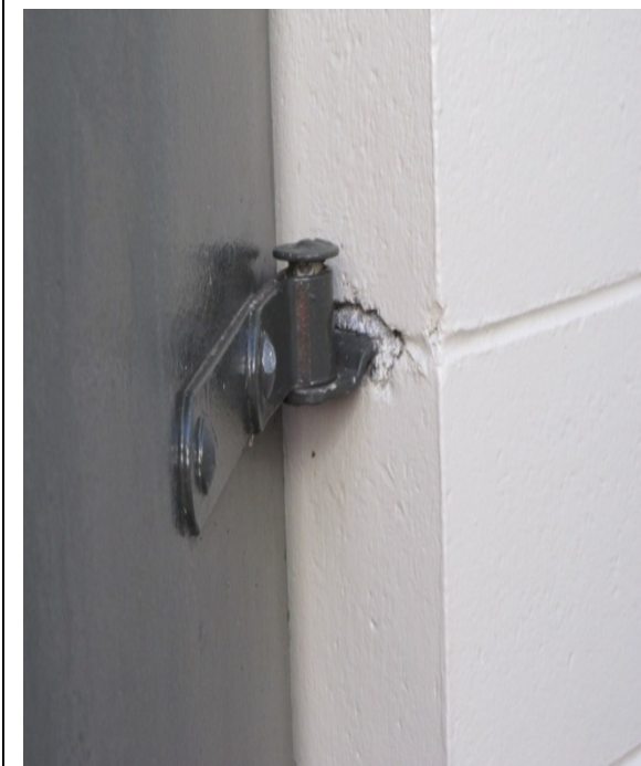
Photo 15: West toilet door connection to masonry wall.
