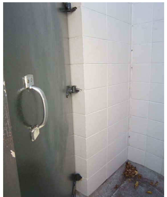
Photo 16: West toilet door connection to masonry wall.
