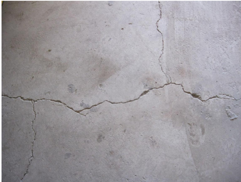
Photograph 9: Typical shrinkage cracks to the concrete floor slab throughout the building
