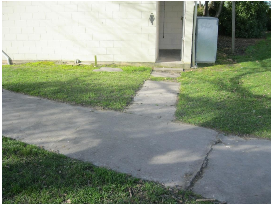
Photograph 10: Damage to the pavement outside the building
