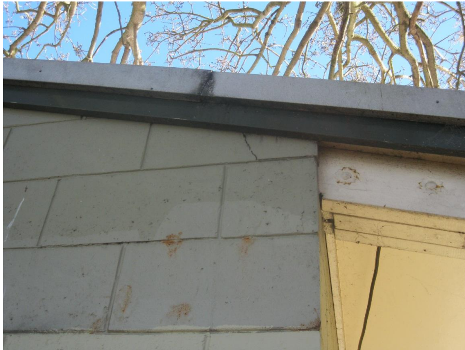
Photograph 5: Cracking to the top of the external blockwork walls on the eastern side
