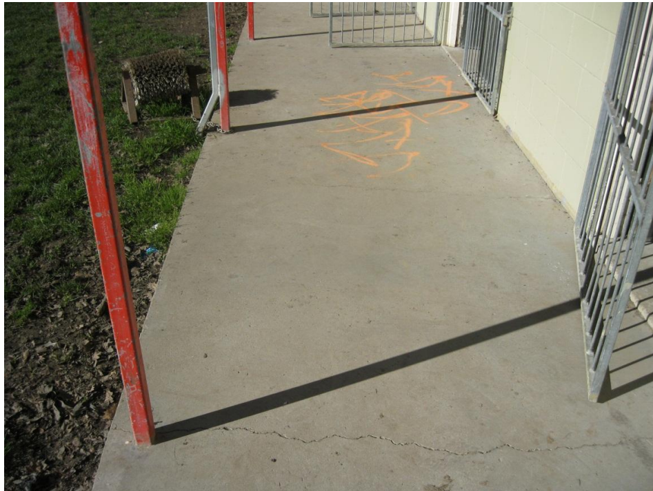
Photograph 7: Cracking to the concrete pavement under veranda canopy
