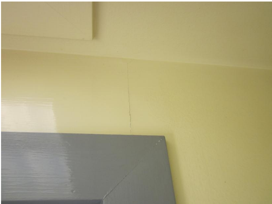
Photo 4: Crack above the door frame
