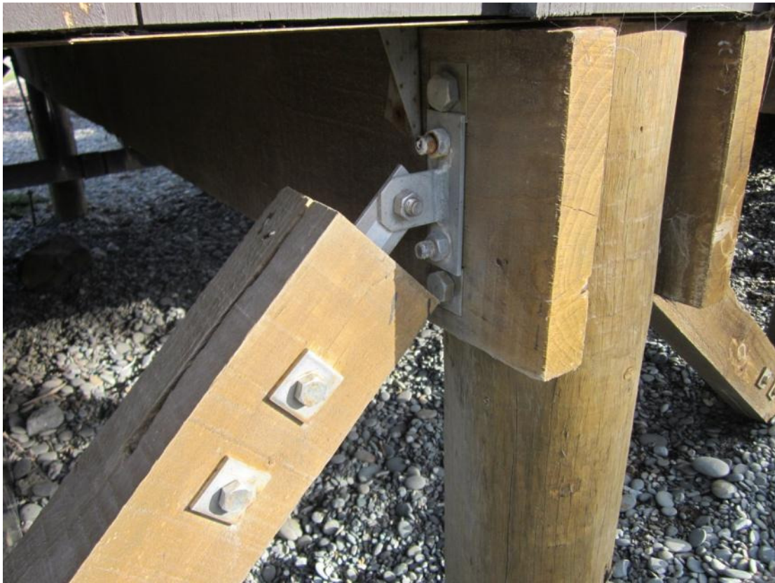
Photo 7: Subfloor bracing
