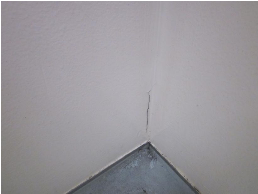
Photo 6: Crack in the corner wall at floor level
