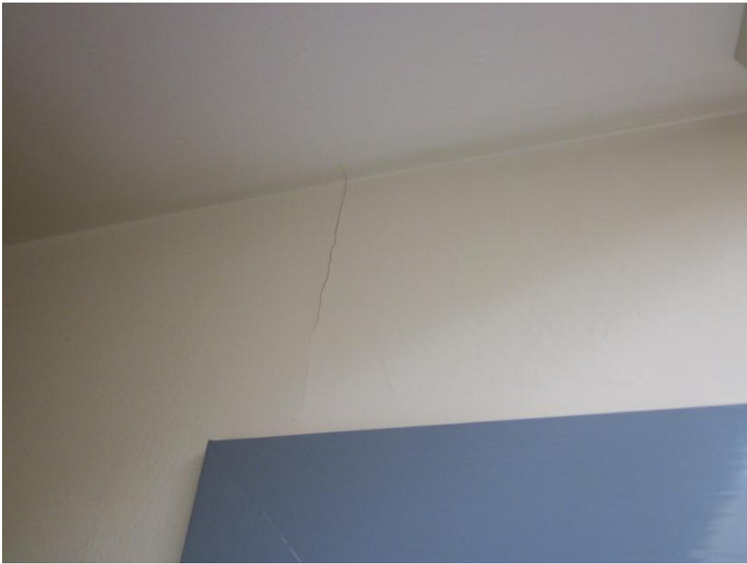
Photo 5: Crack in the wall above the door frame
