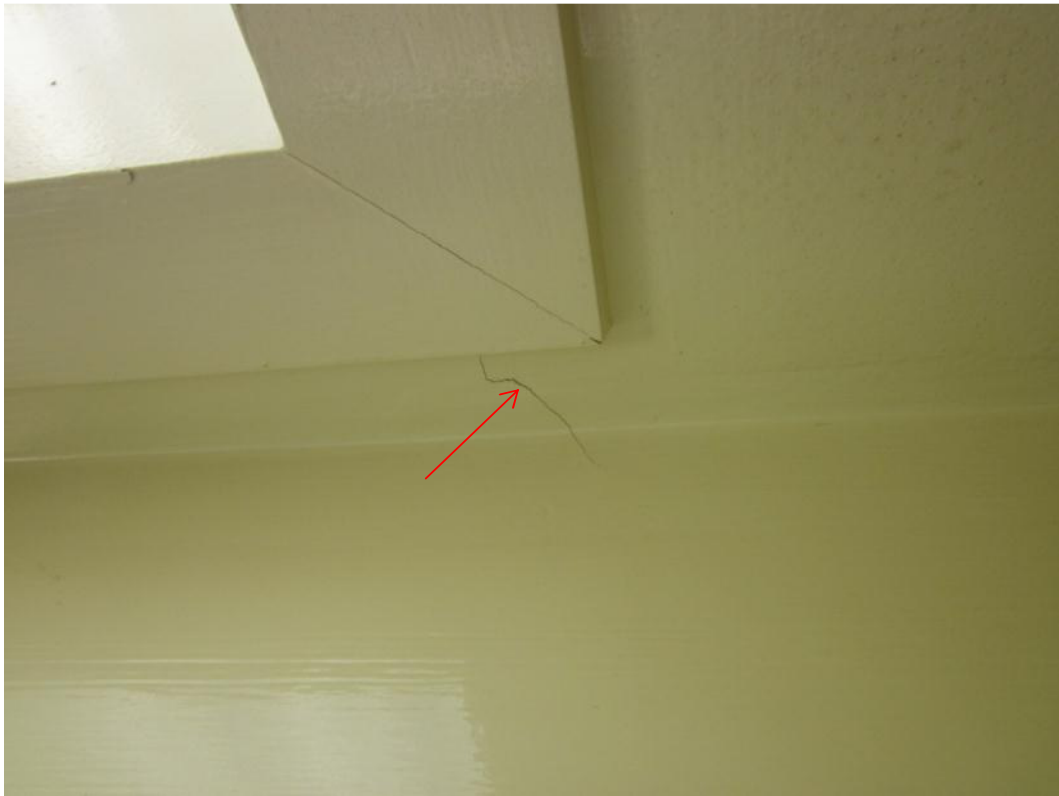
Photo 3: Crack in the roof ceiling
