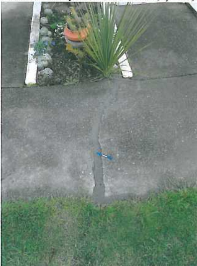
Photo 12: Crack in path with sand boil infill, by Unit 7 and 8
