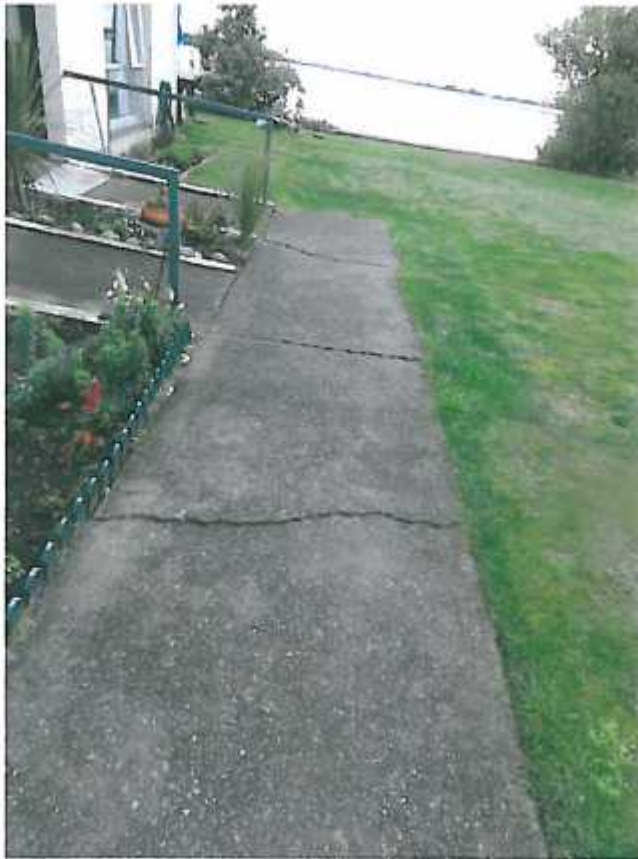
Photo 13: Cracks in path on eastern side of units 7 and 8
