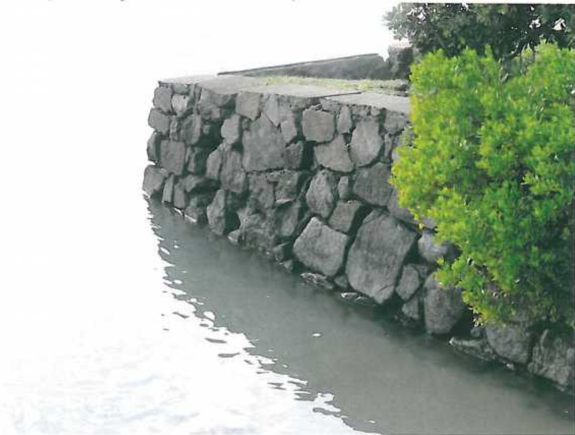
Photo 14: Crack damage to retaining wall in north part of the site.
