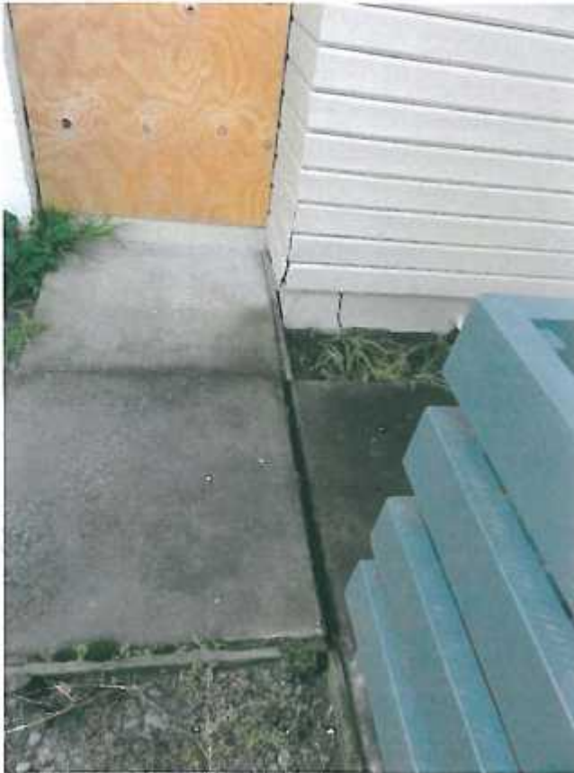
Photo 3: Crack in foundation in western side of Unit 8.
