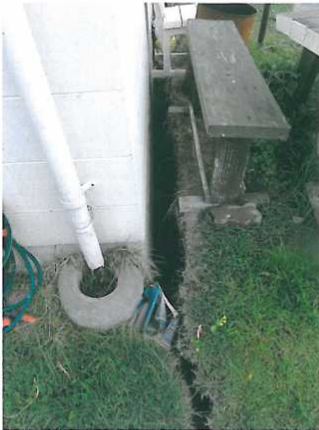
Photo 7: Crack in ground adjacent to northern wall of Unit 6
