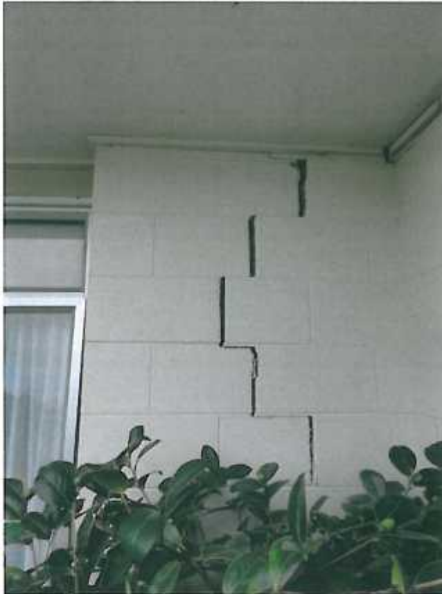
Photo 4: Crack in block-work on north east corner of Unit 9
