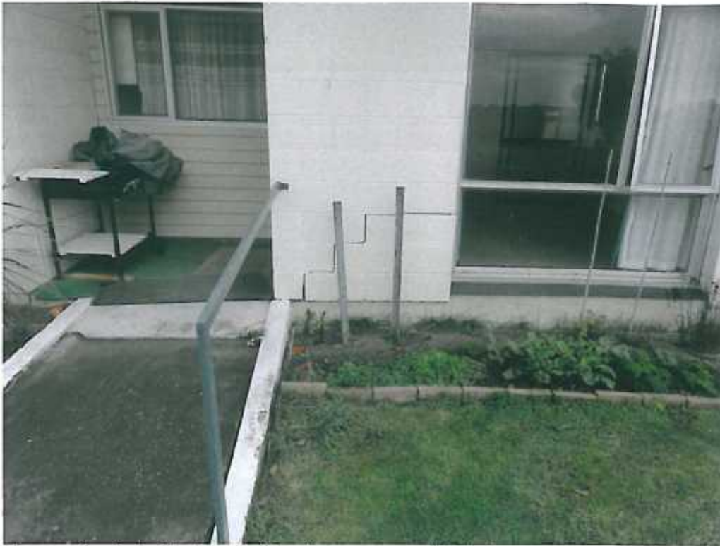
Photo 1: Cracks in block-work of north east corner of Unit 6
