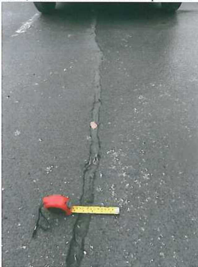
Photo 10: Crack in car park, with sand boil infill
