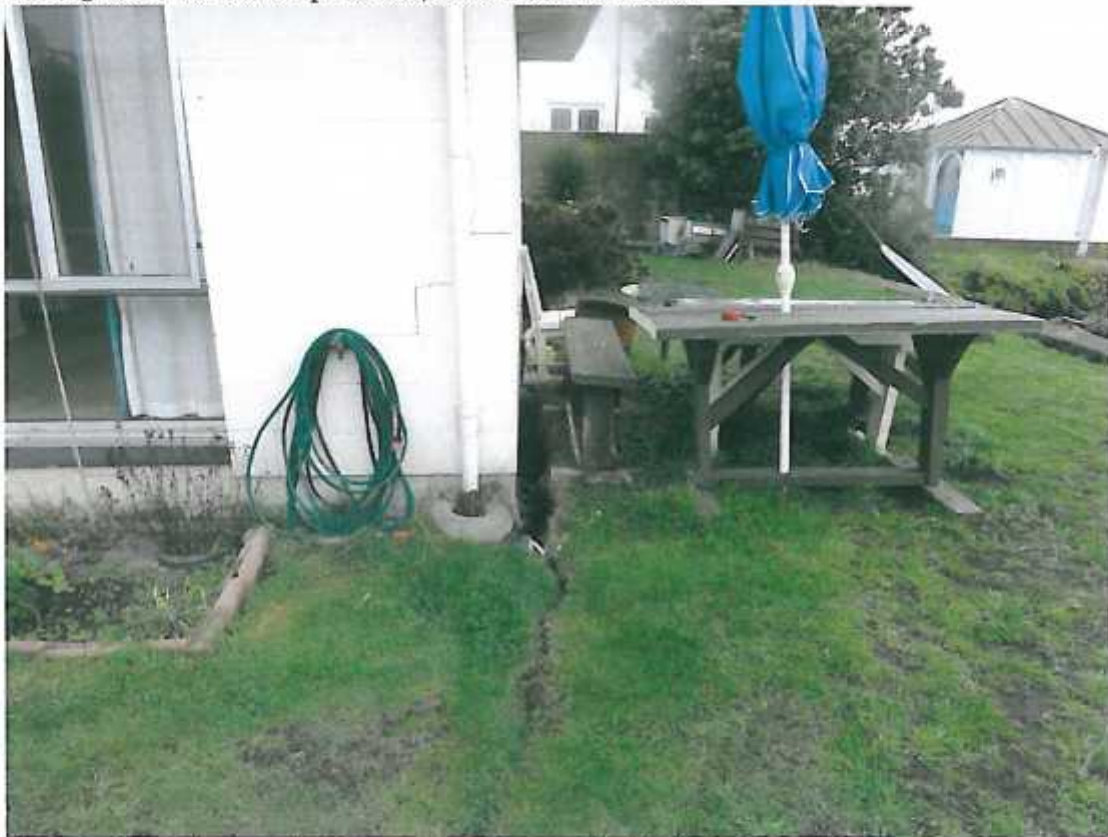
Photo 6: Crack in ground adjacent to northern wall of Unit 6
