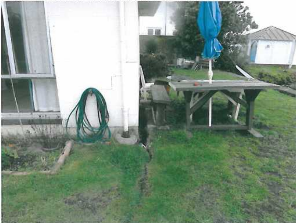
Photo 2: Cracks in block-work of north east corner of Unit 6
