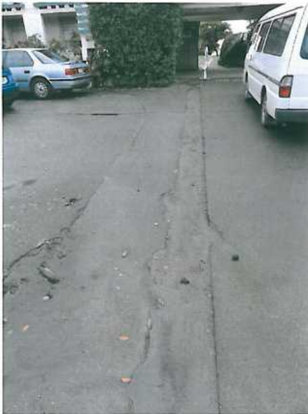
Photo 5: Sand boils in car park area, close to service trench
