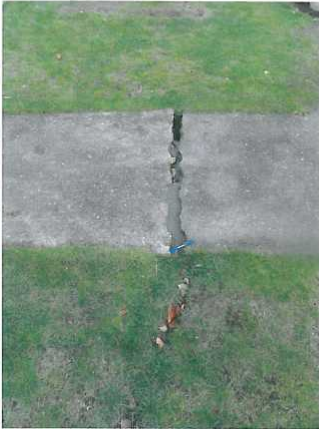
Photo 11: Crack in path with sand boil infill, by Unit 9 and 10
