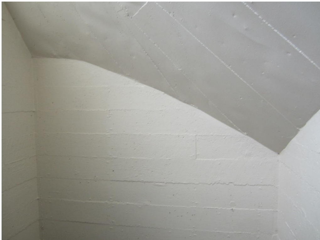
Photograph 4 Reinforced concrete walls and roof slab soffit.
