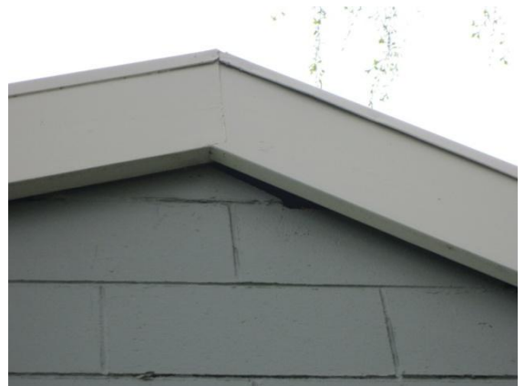
Photo 8: Masonry block at apex cut at a different angle to the timber roof edge beam, reducing weather tightness.
