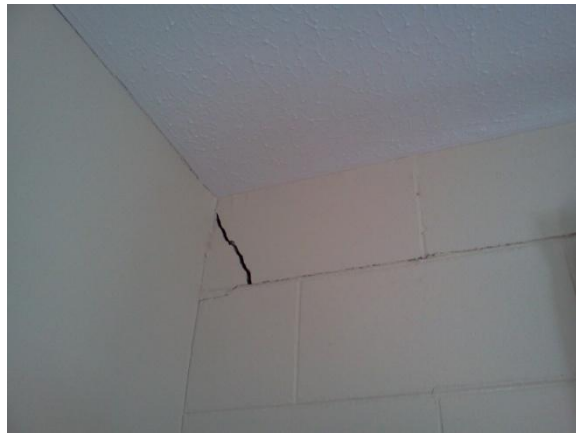
Photo 5: 8mm wide crack through masonry block. Visible from the exterior. (refer to Photo 7 for external view).
