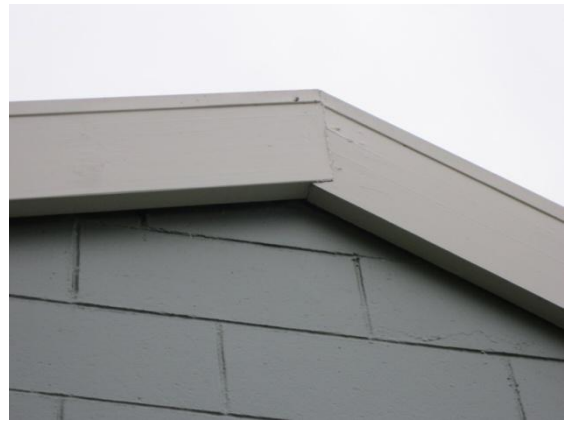
Photo 6: Gap between masonry wall and timber roof edge beam.
