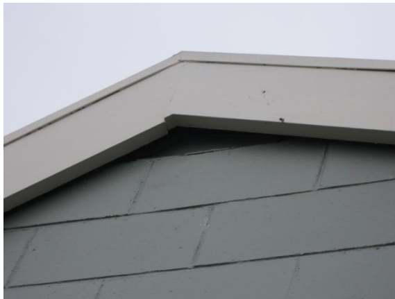
Photo 5: Dislodged or missing block near the apex.
