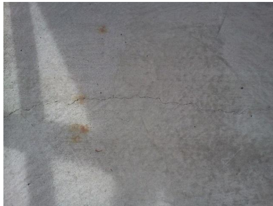
Photo 9: Hairline crack in concrete deck slab
