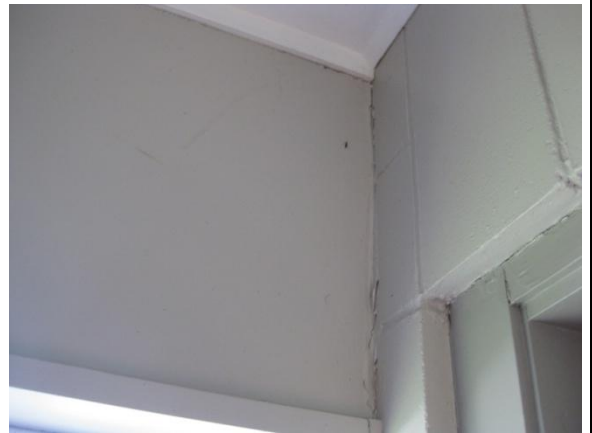
Photo 6: Gap opening up between wall cladding elements
