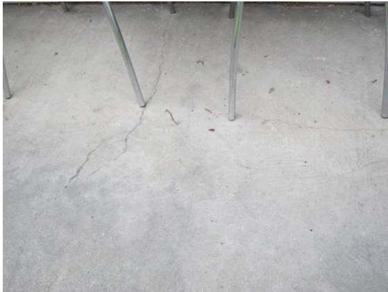
Photo 11: Hairline cracking in external concrete ground slab
