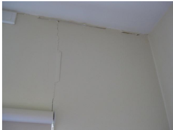
Photo 5: Tearing of wall lining along joints
