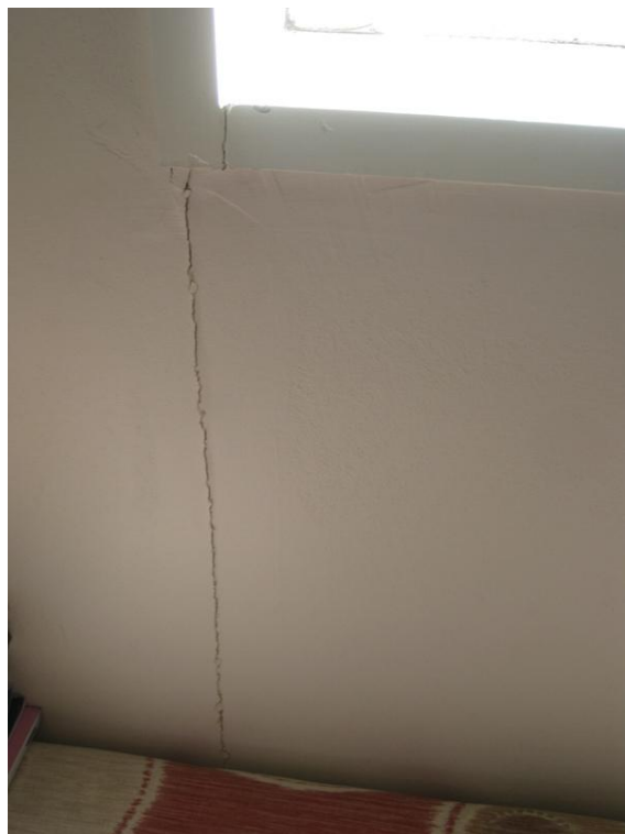
Photo 7: Tearing of wall lining along joints
