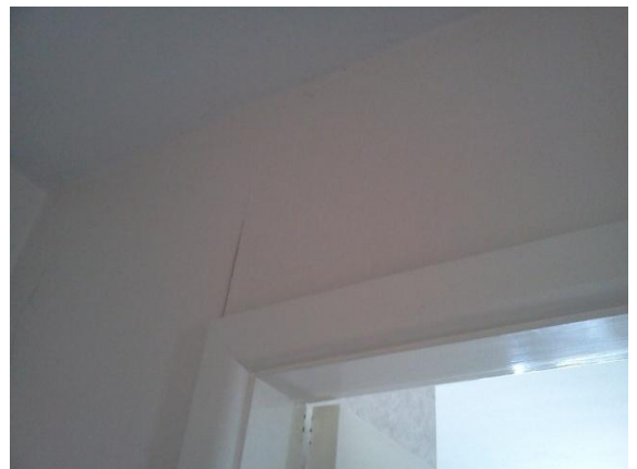
Photo 12: Tearing of wall lining at joints
