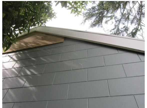
Photo 6: Plywood sheeting near apex appears to be a temporary weather tightness repair.
