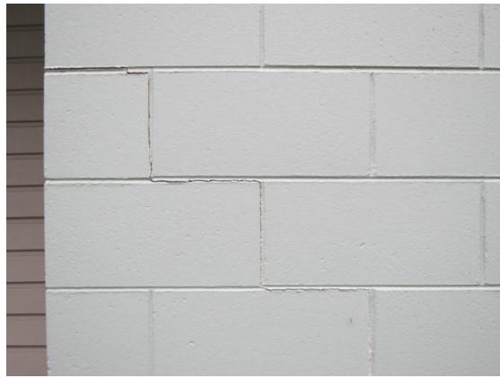
Photo 5: Step cracking along masonry joints
