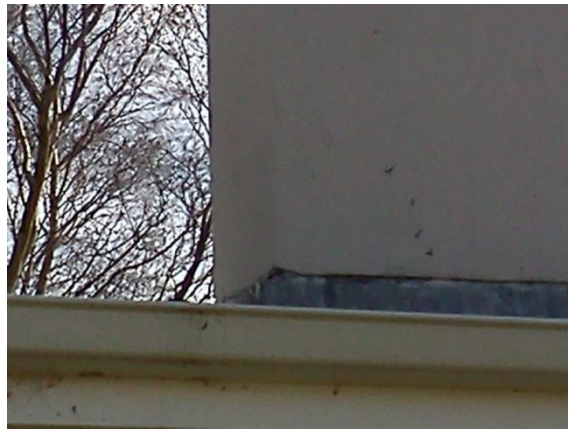
Photo 9: Suspected opening between cladding elements on the west side of the chimney on the south side of the building that is causing water damage inside
