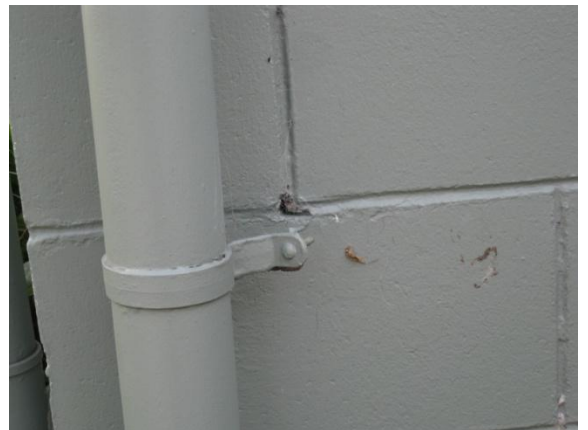
Photo 12: Damaged connection between masonry wall and downpipe. Not structural damage.
