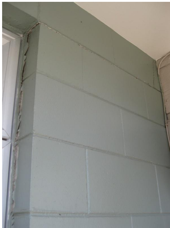
Photo 7: Crack formed between masonry wall and aluminium window frame
