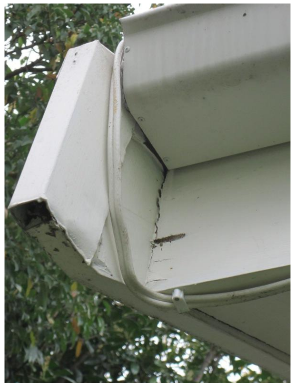
Photo 8: Gap opening up between timber roof cladding elements
