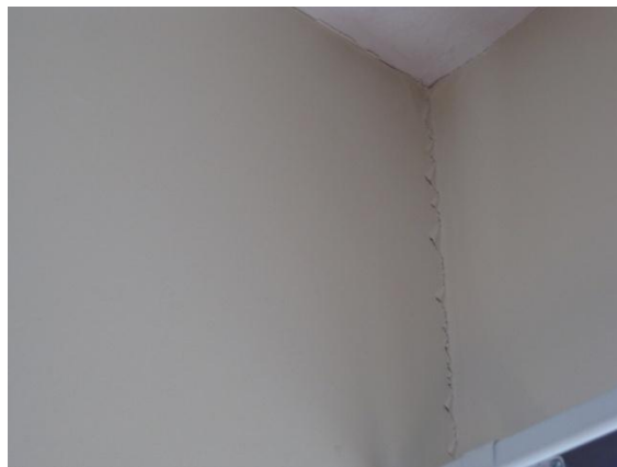
Photo 11: Tearing of wall lining at joints
