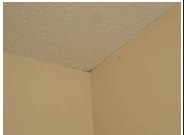
Photo 6: Gap opening up between wall cladding elements
