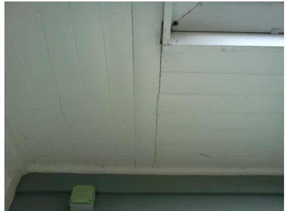
Photo 8: Gap opening up between timber roof cladding elements
