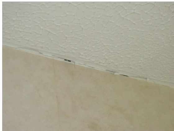
Photo 11: Gap opening up between wall lining and ceiling cladding
