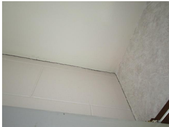
Photo 9: Gap opening up between wall lining, masonry wall and ceiling cladding
