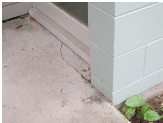
Photo 7: Crack in external concrete ground slab
