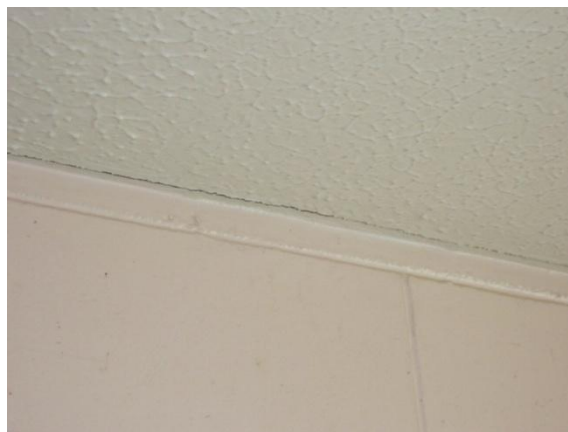
Photo 7: Gap opening up between masonry wall and ceiling cladding
