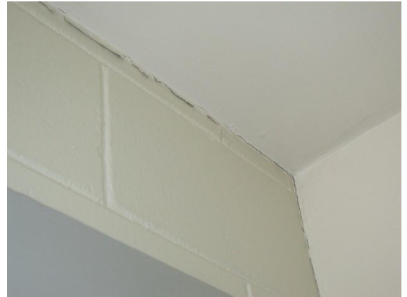
Photo 6: Gap opening up between masonry wall and ceiling cladding
