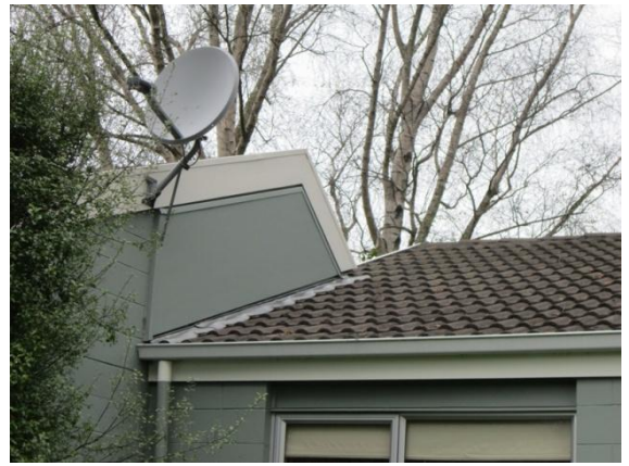
Photo 10: Steel flashing present between offset units
