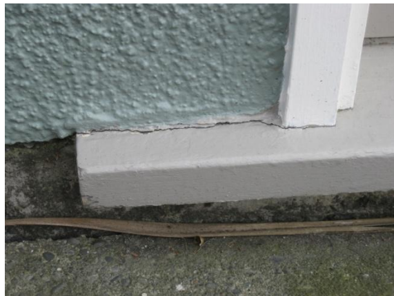
Photo 11: Cracking between timber doorstep and external masonry wall cladding
