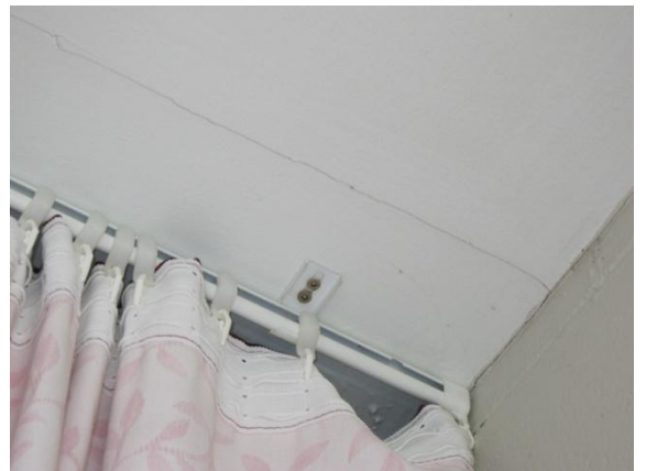
Photo 8: Gap opening up between ceiling cladding panels
