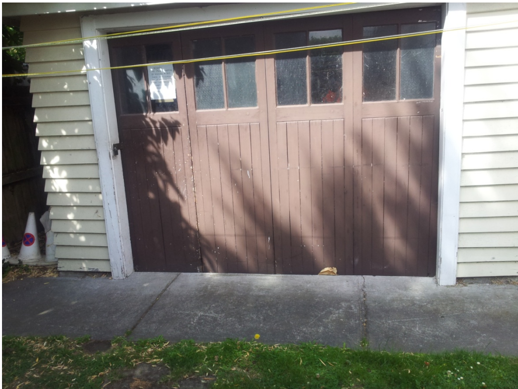
■ Figure 10 – Shed, middle of structure appeared to be sagging.
