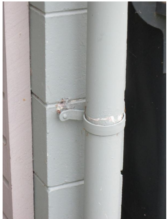
Photo 12: Damaged connection between masonry wall and downpipe. Not structural damage.
