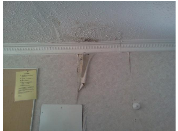
Photo 10: Suspected water damage
