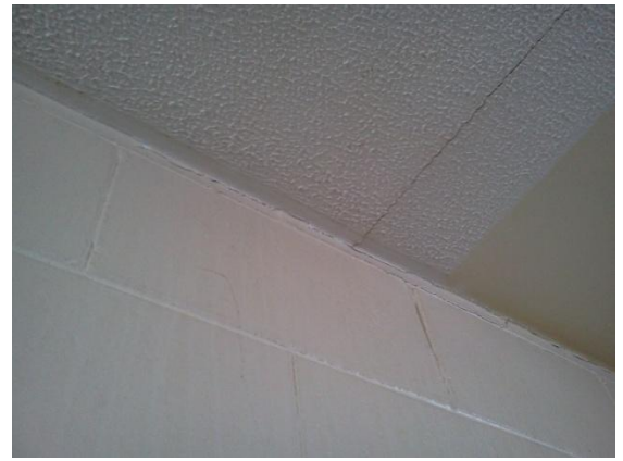
Photo 10: Gap opening up between ceiling cladding panels
