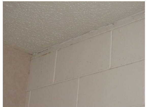
Photo 12: Gap opening up between masonry wall and ceiling cladding
