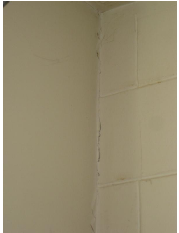
Photo 10: Gap opening up between masonry wall and wall cladding
