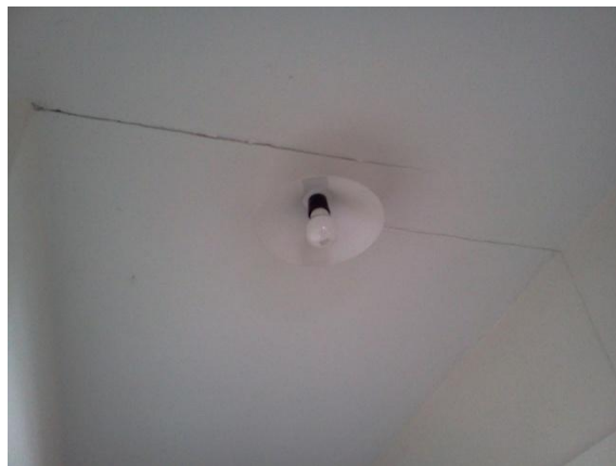
Photo 11: Tearing of ceiling lining at joints
