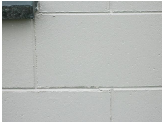
Photo 5: Step cracking along masonry joints
