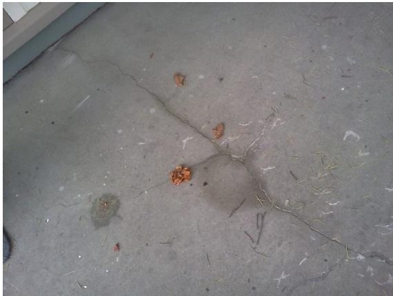
Photo 7: Cracking in external concrete ground slab
