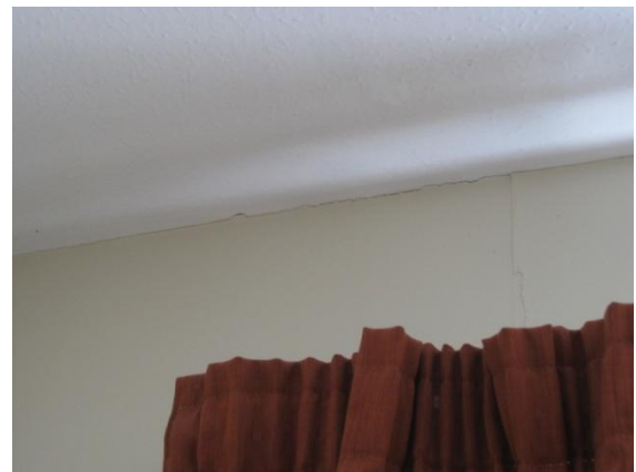
Photo 12: Tearing of wall lining at joints
