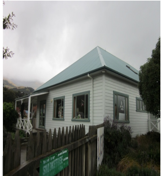
Photo 6: View looking north-west
