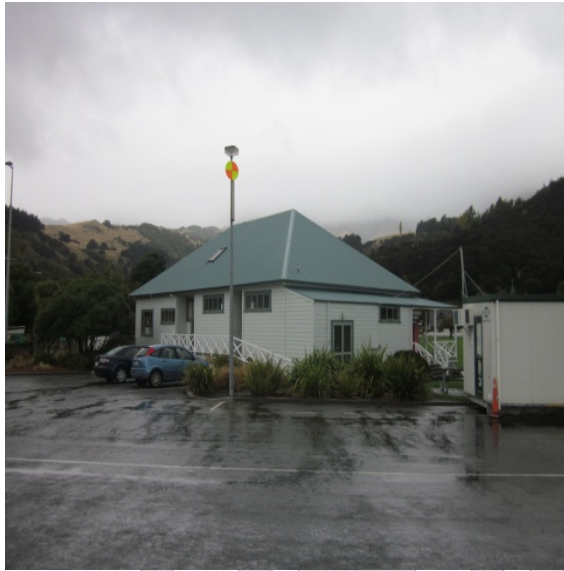
Photo 1: View of the building looking East
