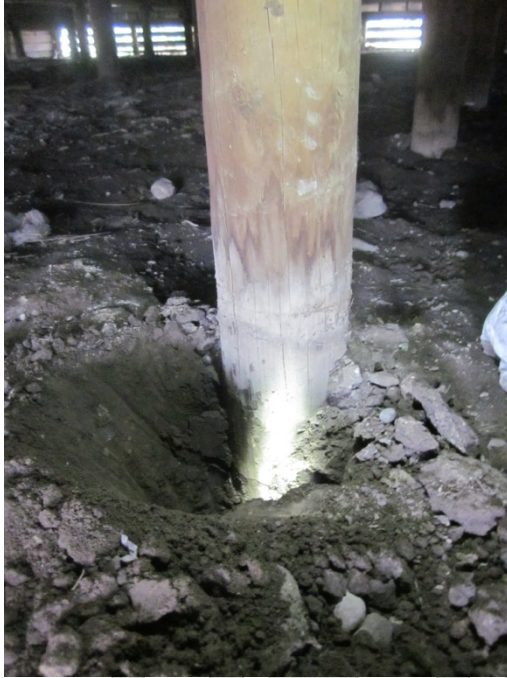
Photo 15: View of exposed timber pile beneath ground level
