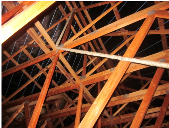
Photo 17: View of roof framing (2)
