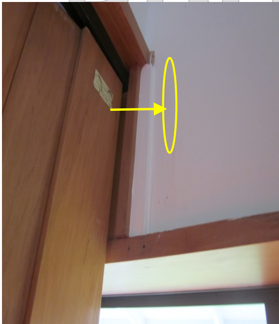
Photo 11: Lining damage
