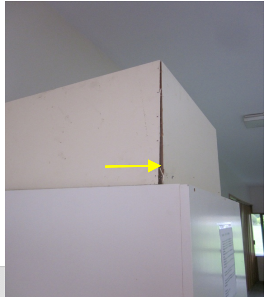
Photo 10: Damage to timber enclosure in kitchen.
