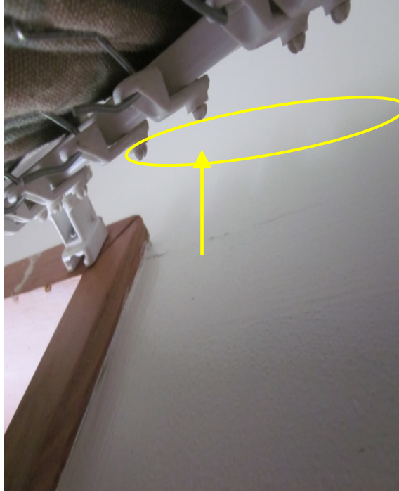
Photo 13: Lining damage
