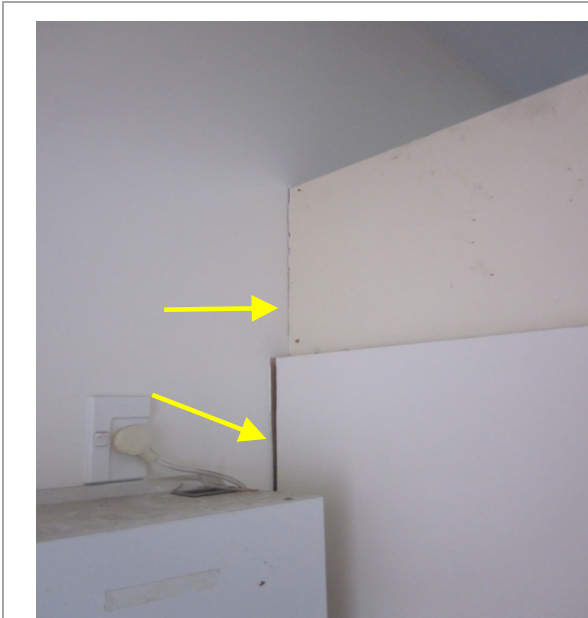
Photo 9: Movement between kitchen timber enclosure and adjacent wall.
