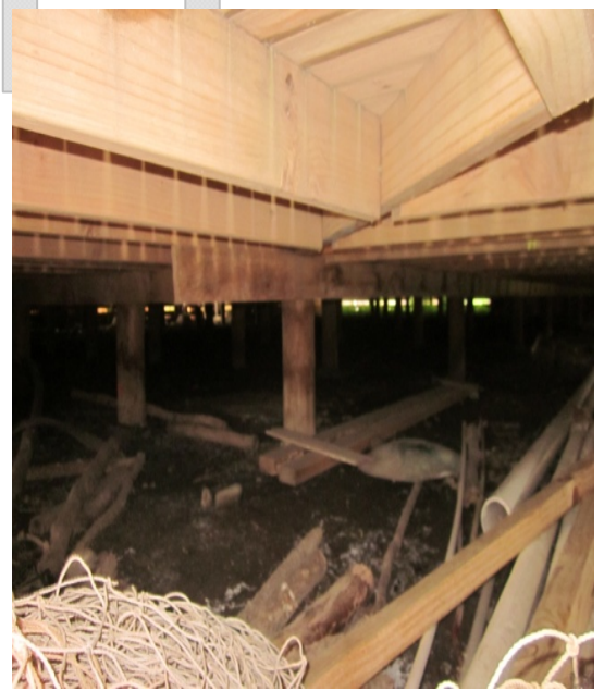
Photo 8: Typical view of the building substructure.
