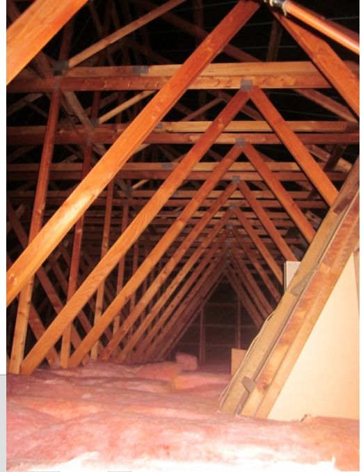
Photo 16: View of roof framing (1)
