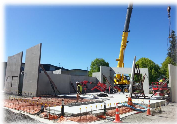
Arrival of pre-cast concrete panels on site
