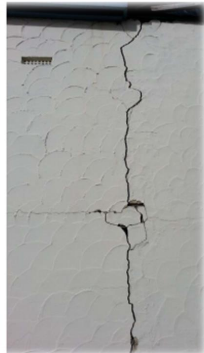
A significant exterior crack
