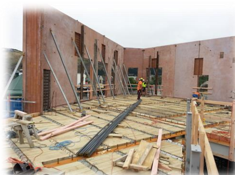
Carpenters preparing the first floor for a concrete pour
