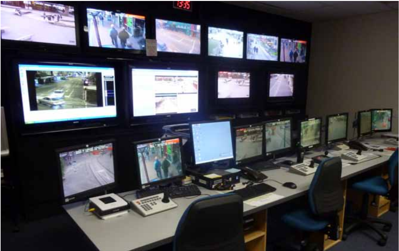
View of the new Camera Monitoring room in the Christchurch Central Police Station
