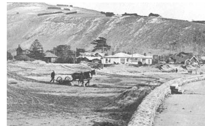
Figure 9. Sand hills being levelled and the new protective wall being reinforced at the Scarborough end of Sumner beach, 1931. Source: The Press.
