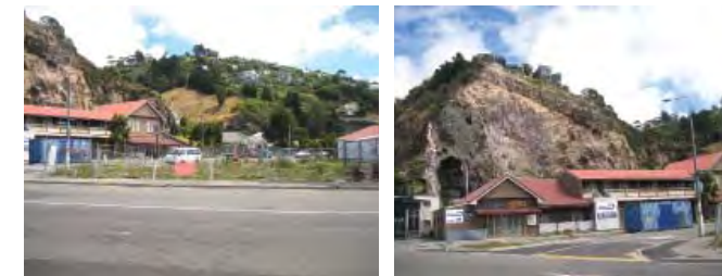
Figures 69 and 70. The site of the demolished Community Centre / Museum and 'The Marine', still standing but within the CERA Red Zone.
