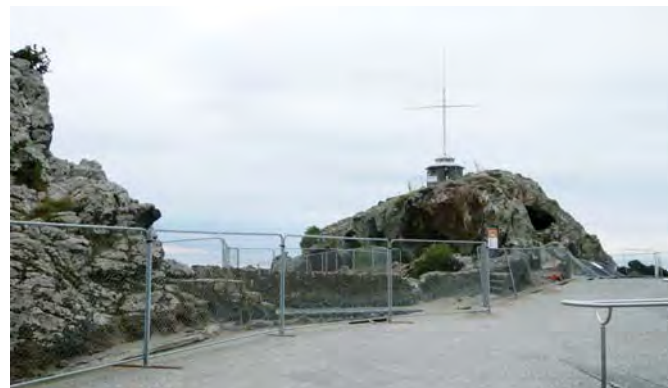
Figures 19 and 20. Sumner library post-2011 earthquake (now demolished) and Cave Rock / Tuawera 2012 (fenced off).
