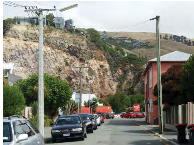
Figure 49. Burgess Street looking south.
