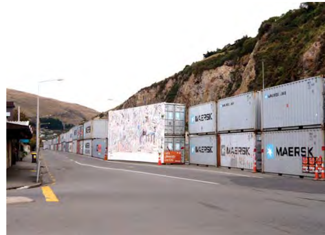
Figure 31. Containers placed for protection against rockfall along Wakefield Avenue.
