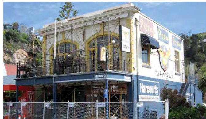
Figures 17 and 18. Sumner Community Centre and Museum and the Ruptured Duck Restaurant post-2010 earthquake (both now demolished).
