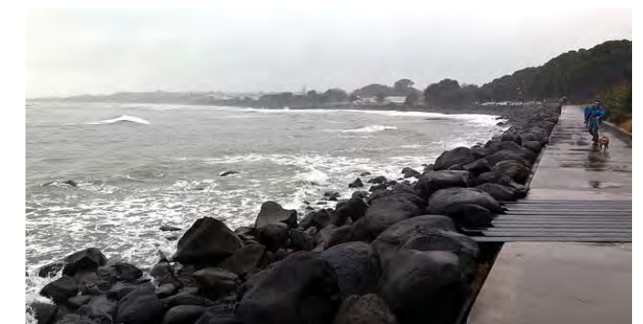
Figure 75. Coastal walkway in New Plymouth.
