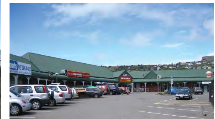
Figures 27, 28 and 29. Poor quality spaces and landscape elements.
