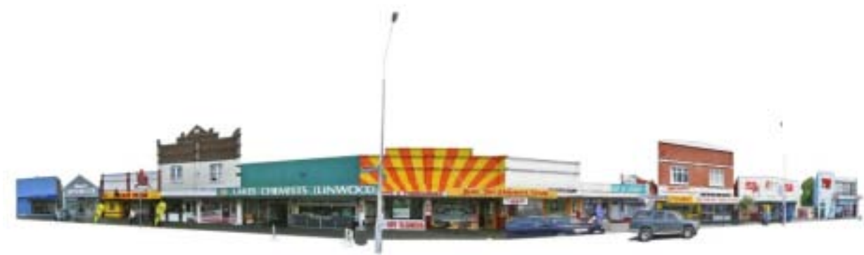
Figure 11. North-west corner of Worcester Street and Stanmore Road prior to demolition
