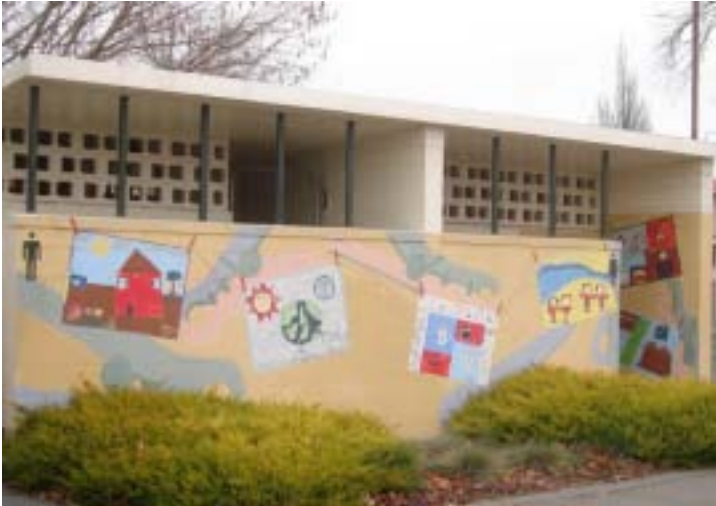
Figure 21. Toilet block on Worcester Street
