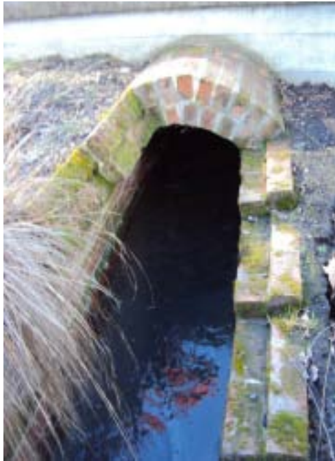
Figure 35. Exposed brick barrel culvert
