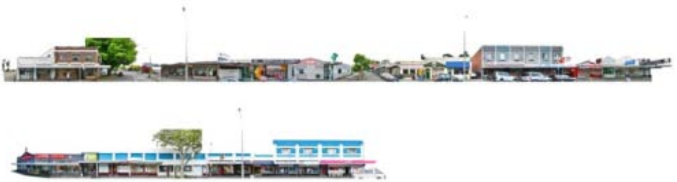
Figure 12. Pre-earthquake street frontage (2009)
