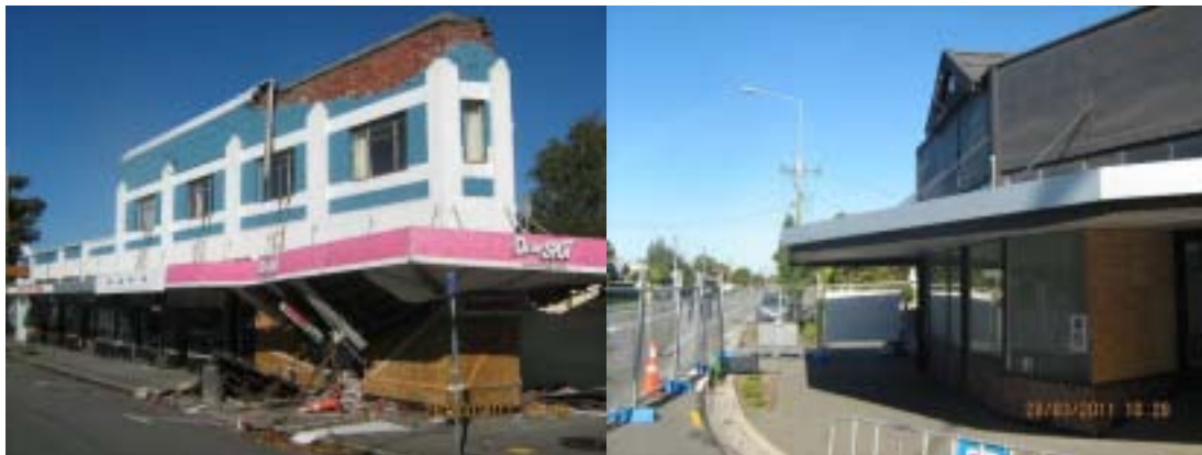
Figure 6. March 2011, damage to 299 Selwyn Street block
