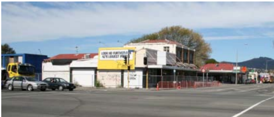
Figure 19. 320 Selwyn Street post-earthquake
