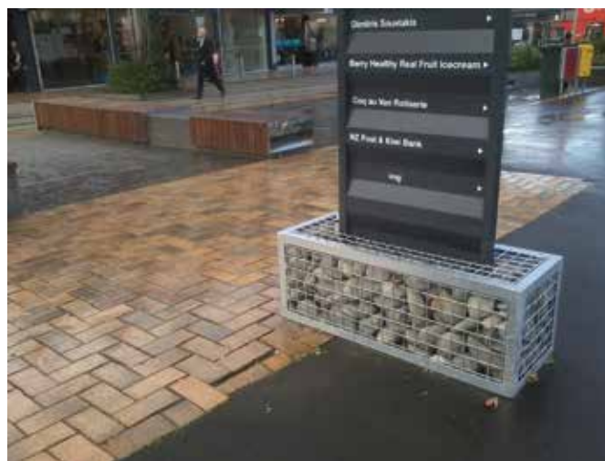
Figure 27 – An example of gabion street furniture using local materials, Re:Start Mall, Christchurch
