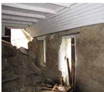
Figure 15 – Original Penfolds Cottage (source: NZ Historic Places Trust), and earthquake damage to the cob cottage
