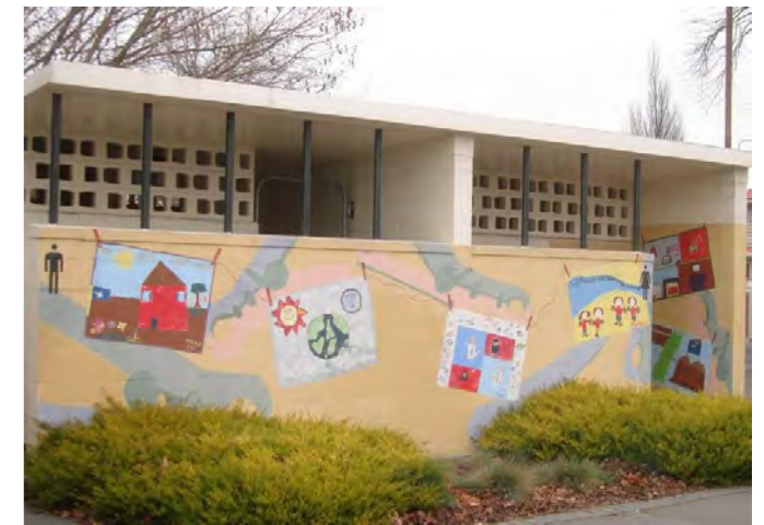
Figure 24. Toilet block on Worcester Street
