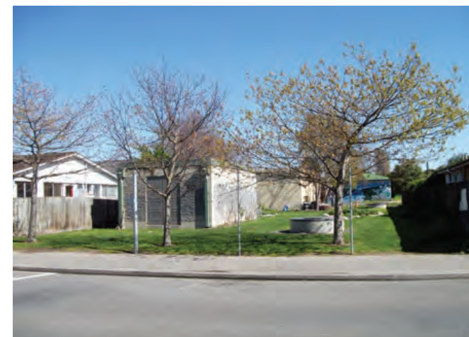
Figure 2j – site used by Edgeware Village Green showing a number of site constraints – the substation, wellheads and pump station
