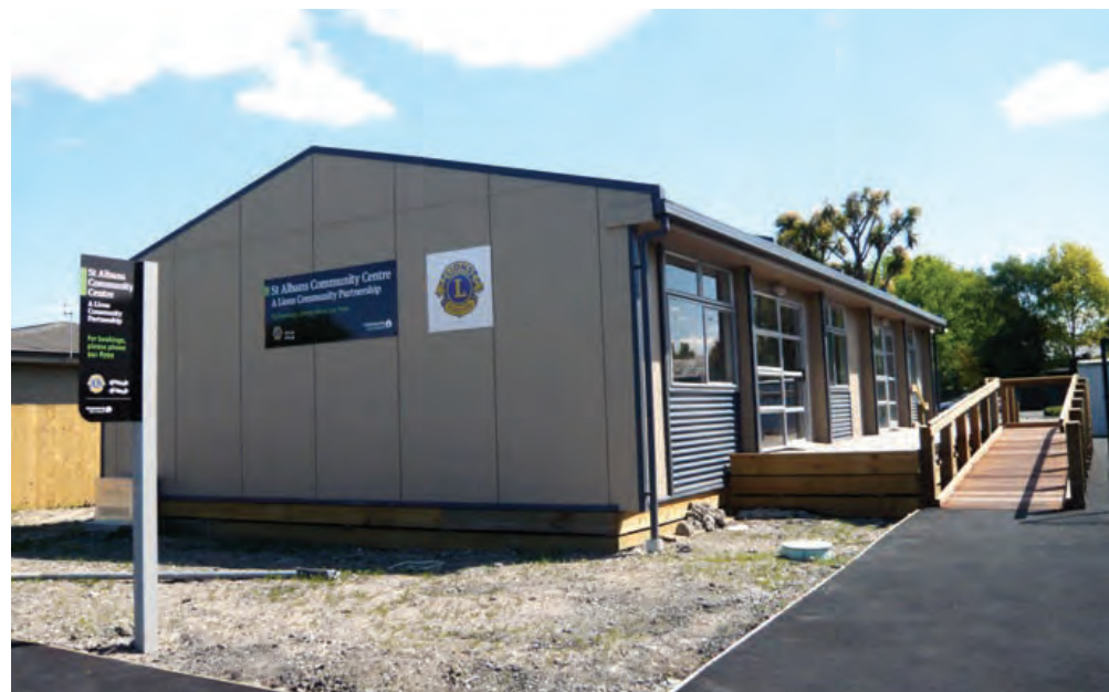
Figure 2l – the transitional community facility on Colombo Street
