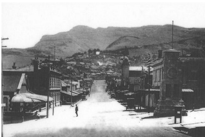
Below: Historically the cenotaph used to be located in the heart of the centre at the eastern end of London Street (www.ccc.govt.nz)
