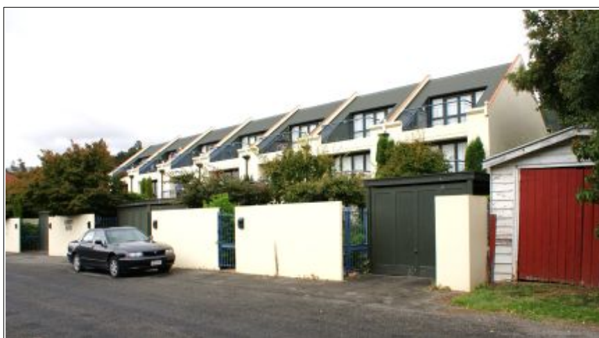
Figure 7.17. The Aubrey Mews, three storeys high and with garages and solid walls on the street frontage, was one of the first of the new, larger developments which aroused disquiet among those who felt such buildings had no place in Akaroa.
