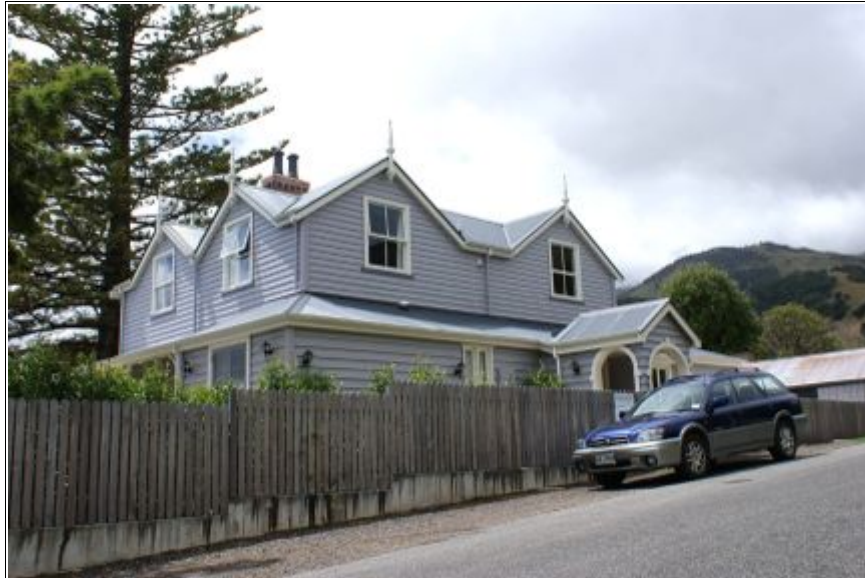
Figure 7.22. The Haylock House on Aylmer's Valley Road was one of Akaroa's most historic houses. The recent addition of a second storey seriously compromised its historic value.
