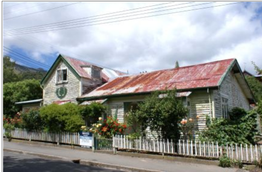
Figure 7.24. The survival of this historic house on Rue Balguerrie, for long the home of an Akaroa identity, hangs in the balance as the property awaits a new owner.
