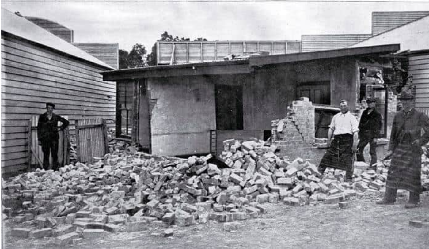
Some of the destruction by earthquake at Cheviot, North Canterbury, 16 Nov. 1901 : back of McTaggart's butcher/baker shop. [17 Nov. 1901] CCL PhotoCD 5, IMG0067ChristChurch Cathedral was damaged by three quakes during its construction – 1881 , 1888 and 1901 .
