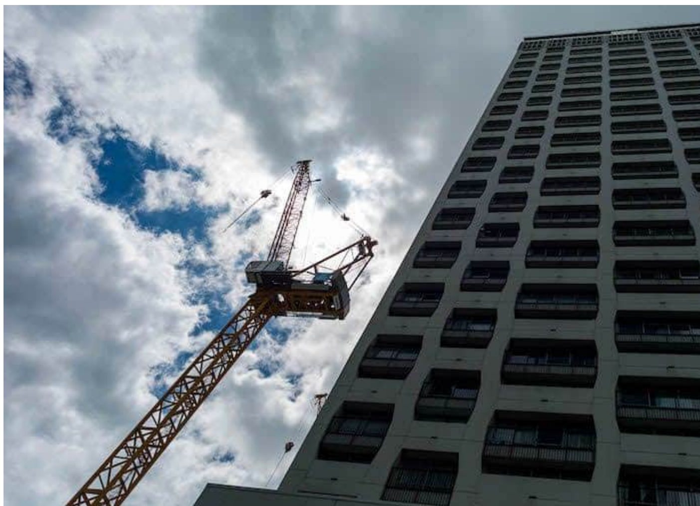
One of the buildings that is put under the microscope in Living Hell. (Photo: Sky)
