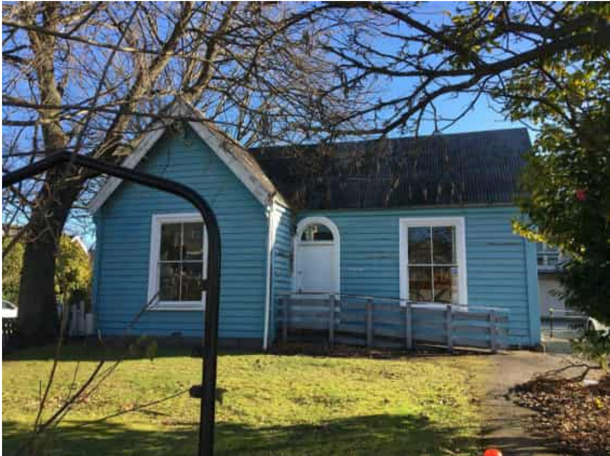
Former Townend cottage, 325 Montreal Street, c.1875. Dr A McEwan.
