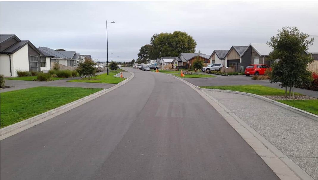
Photograph 3-12: Leistrella Road Looking North
