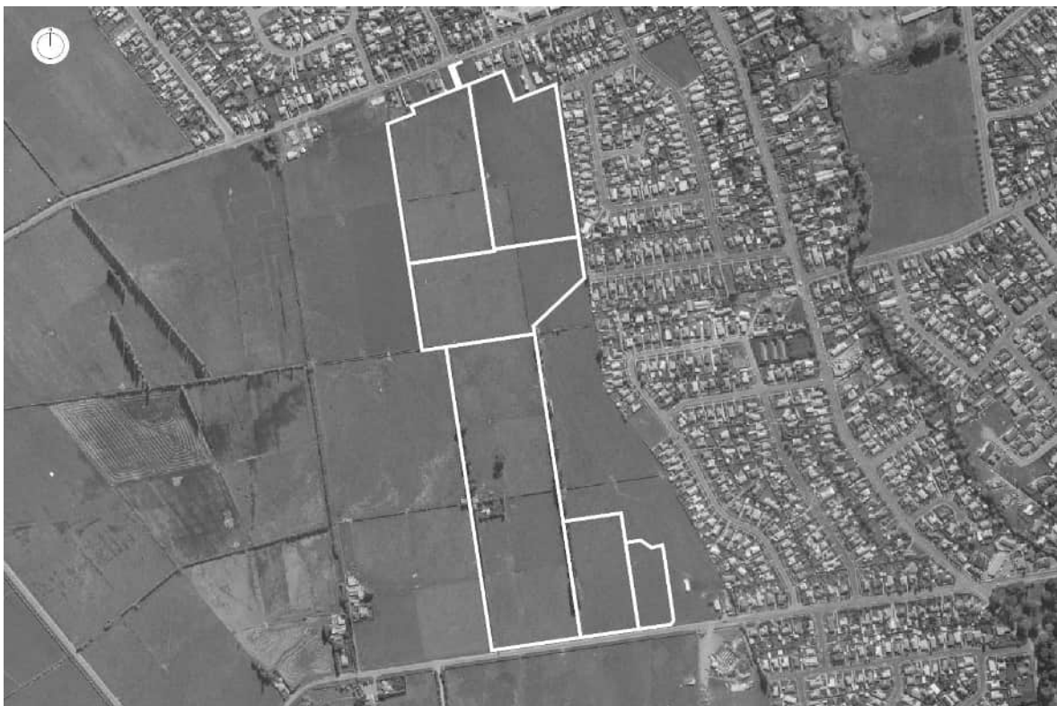
Aerial imagery of Cashmere properties in 1970-1974 (site boundary outlined in white). Retrieved from Eliot Sinclair Desktop Study.
