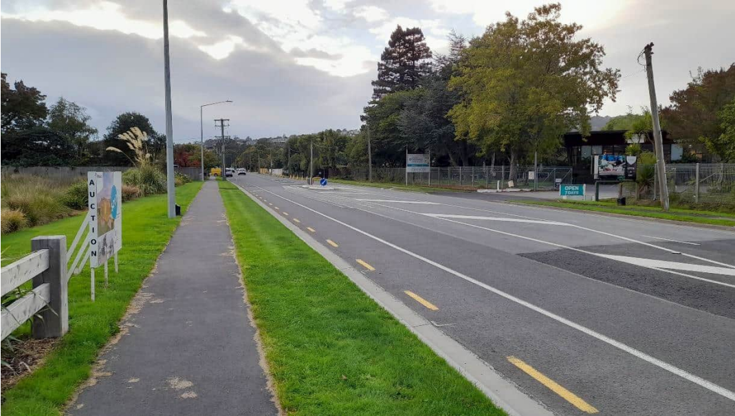
Photograph 3-14: Cashmere Road East of Leistrella Road
