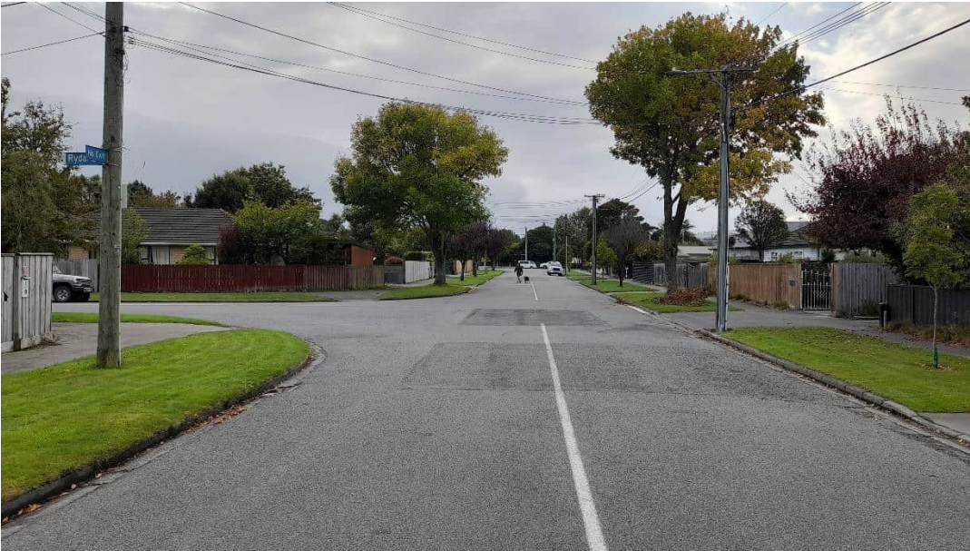
Photograph 3-10: Leistrella Road / Rydal Street Intersection
