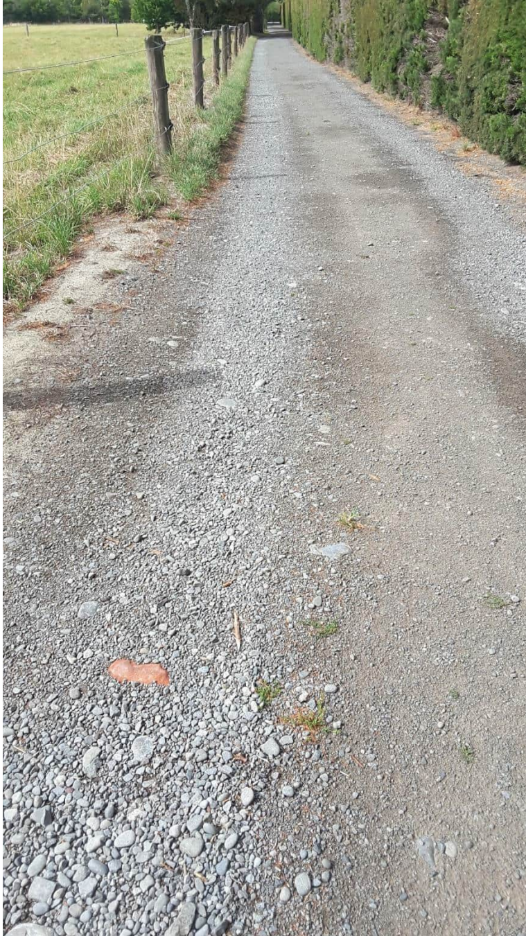
B) Driveway for 240 Cashmere Road that is possibly created with rubble material.
