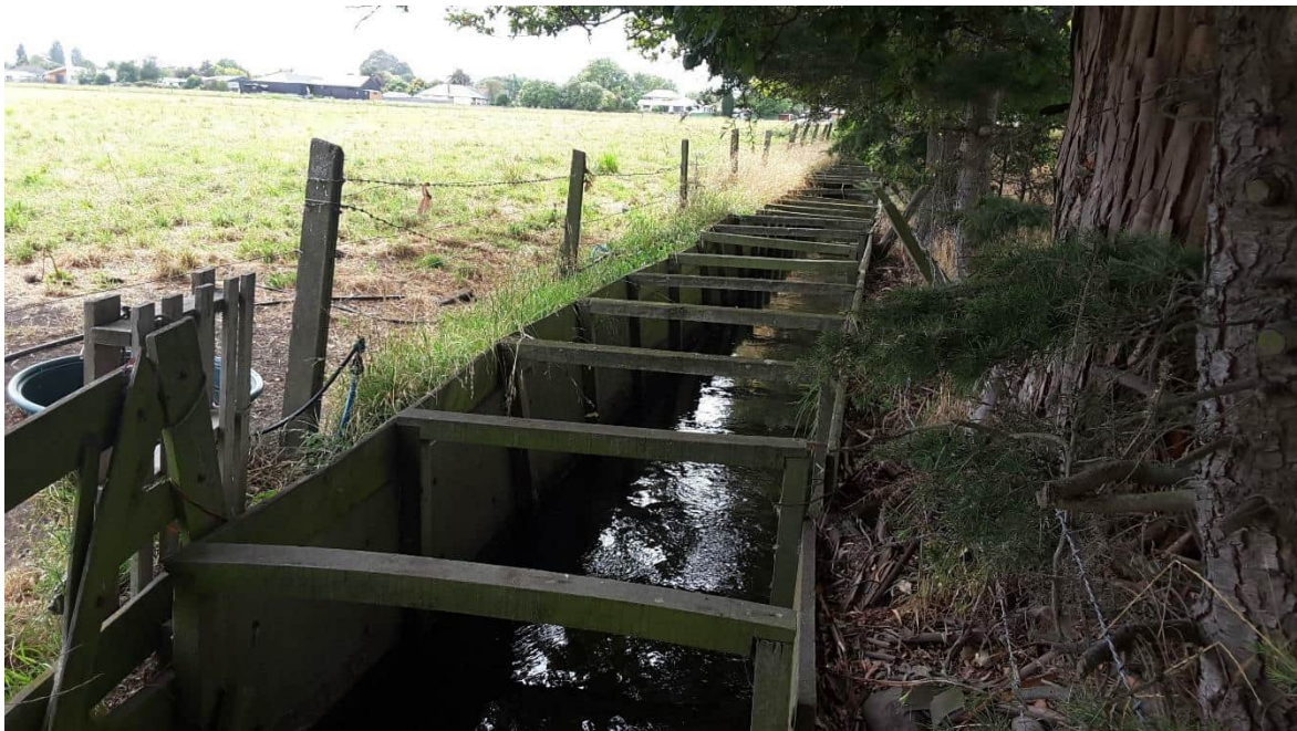
D) Box drain at the northern boundary of 240 Cashmere Road
