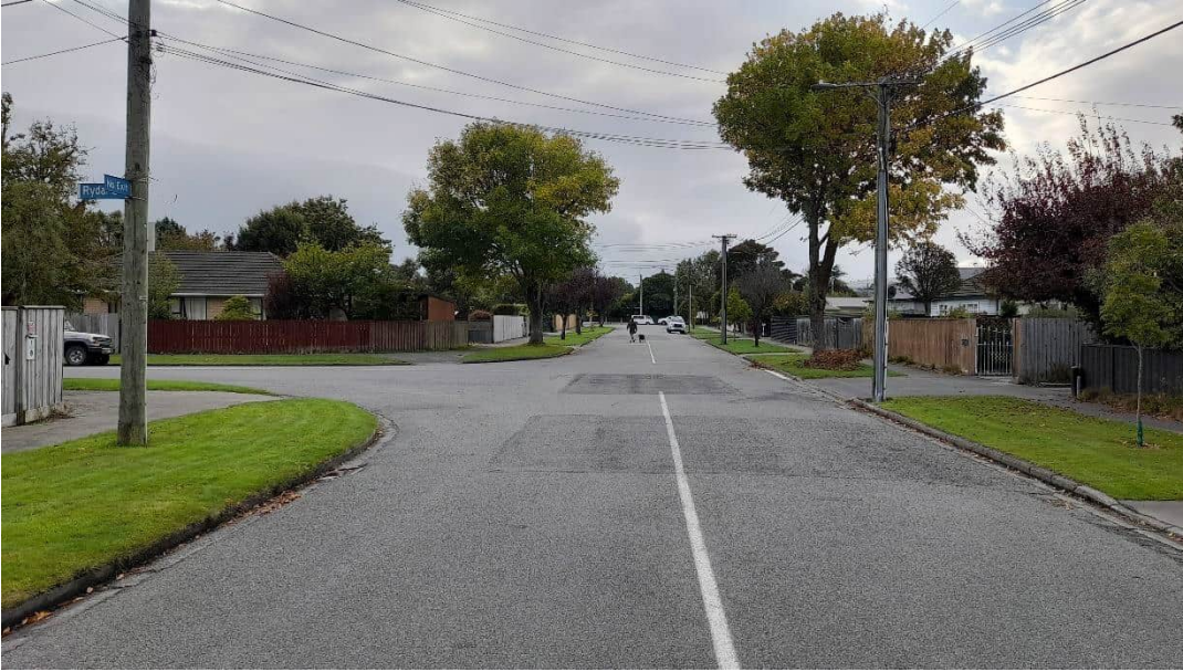
Photograph 3-10: Leistrella Road / Rydal Street Intersection
