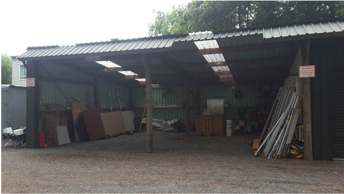
I) Pole shed at 236A Cashmere Road
