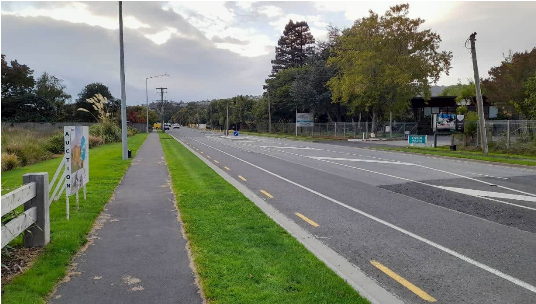
Photograph 3-14: Cashmere Road East of Leistrella Road
